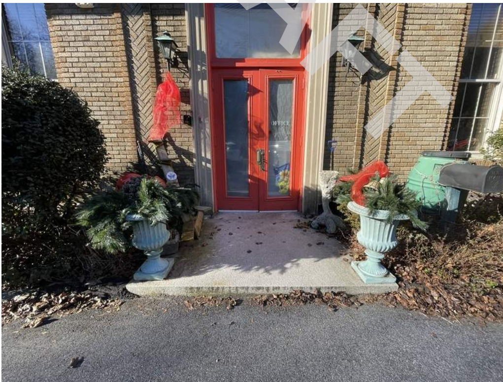
18 - Main entry door consists of a wood framed single pane glass assembly.
