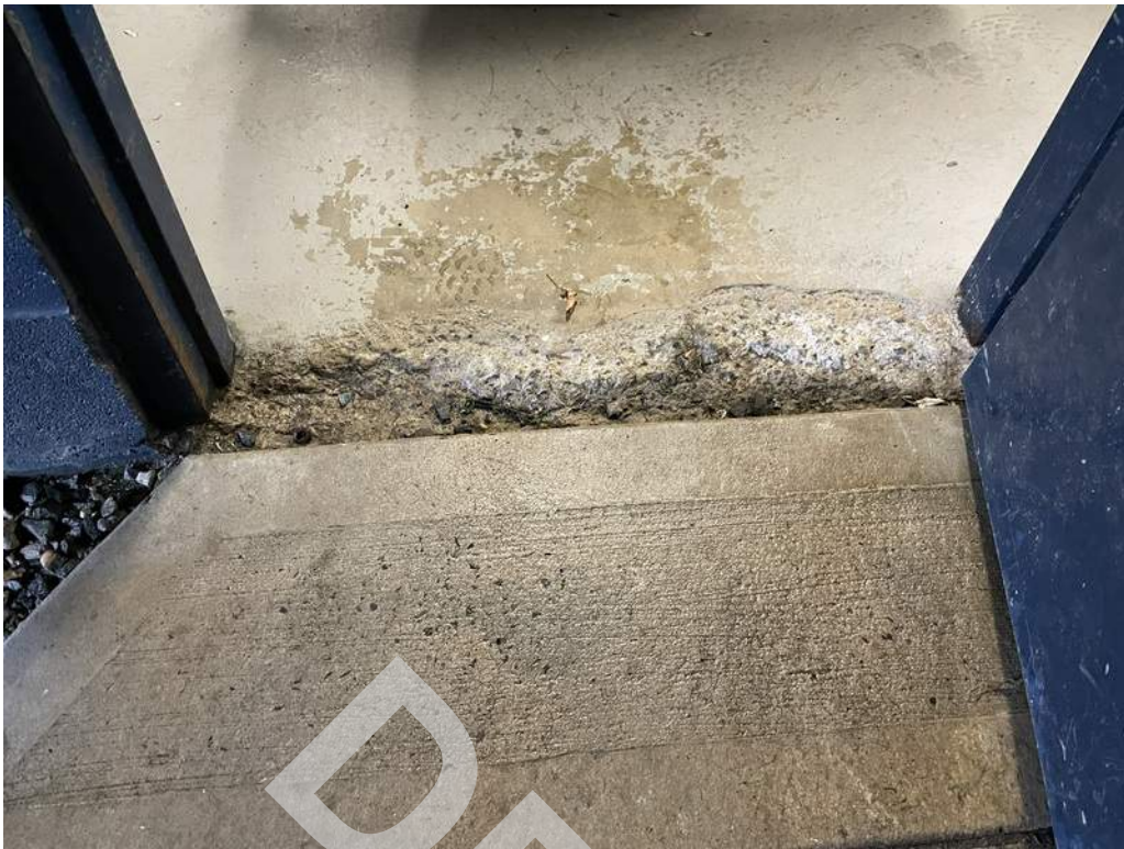
5 - Concrete floor is spalling along one of the entrances.
