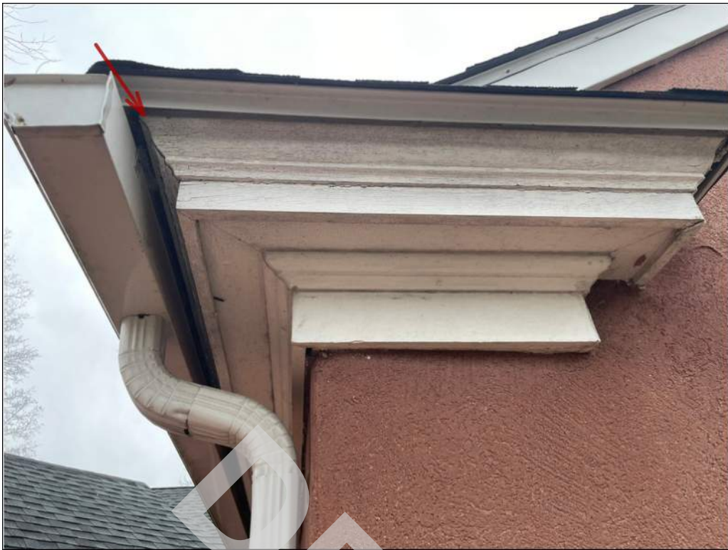
17 - Wood trim paint finishes are cracking.
