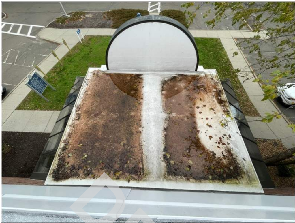
15 - Debris accumulation and water ponding at the low roof over the secondary building entrance.
