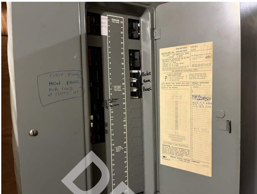
53 - Two electric panels located in the electric service room are Stab-Lok model Federal Pacific panels.
