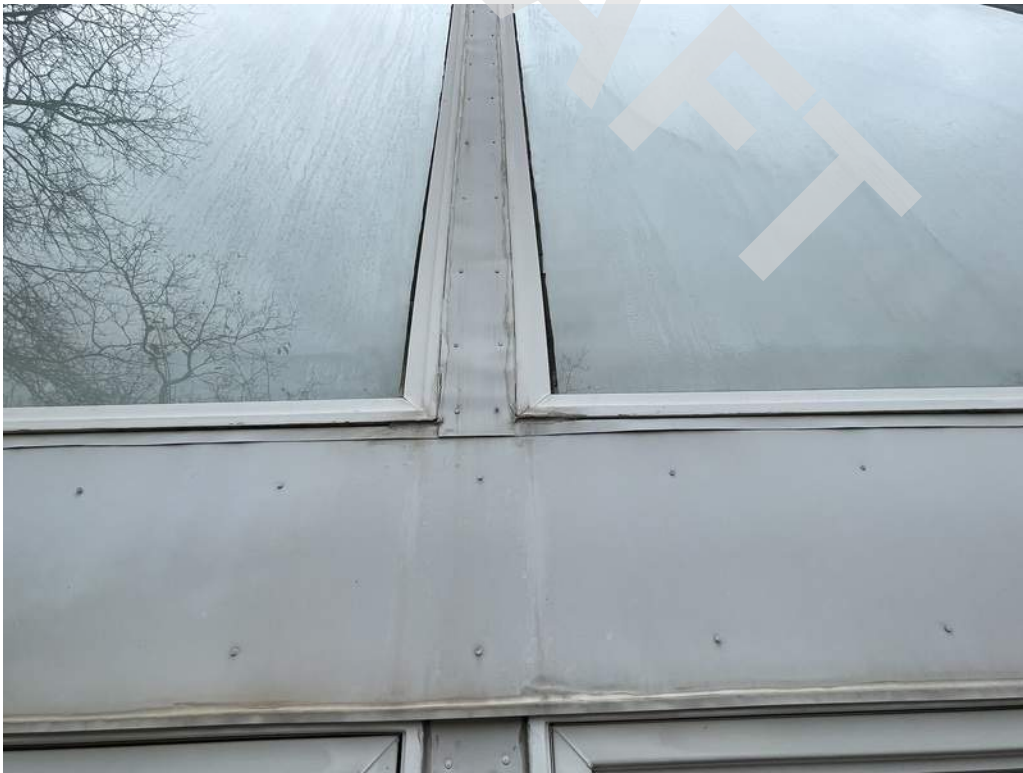
12 - Insulating glass units within the quarter round windows have failed and have internal condensation.
