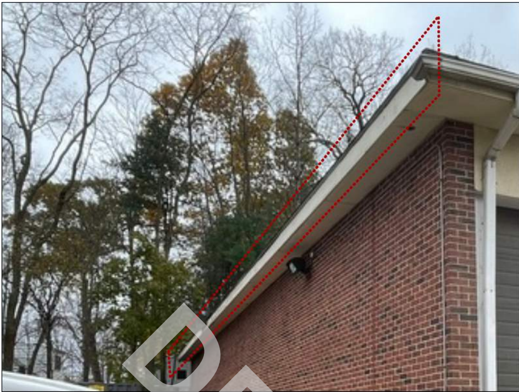
11 - Close up view of missing roof gutter along the east end of the building.
