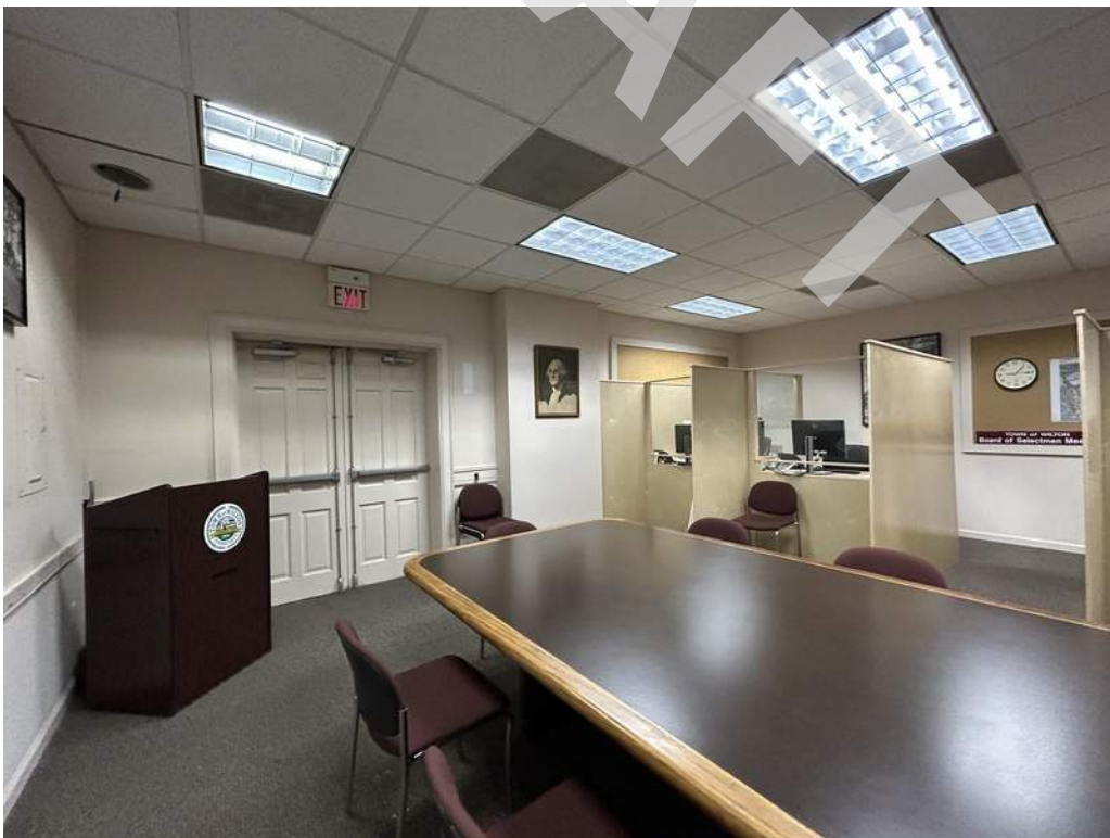
40 - Conference rooms generally consist of painted gypsum wall boards, suspended grid ceilings with acoustic tiles, and carpet floors.
