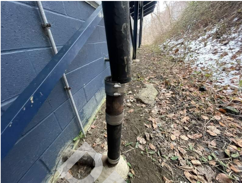
23 - A vent pipe on the exterior of one team room has broken and is currently disconnected.
