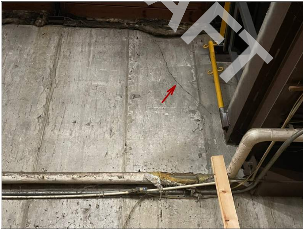
6 - Localized areas of the reinforced concrete wall have cracked.
