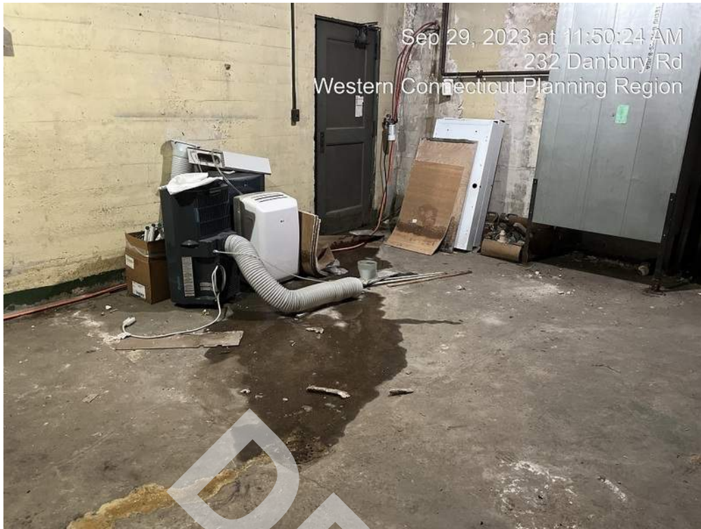
19 - Water intrusion at the boiler room.
