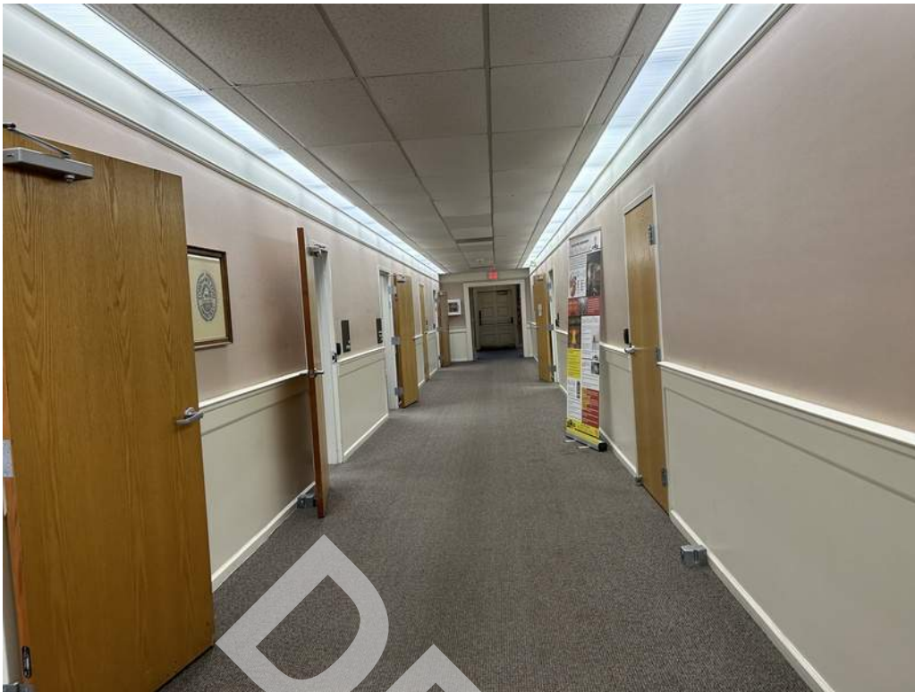
39 - Interior finishes at the corridors on the first floor typically consist of painted gypsum wall boards, suspended grid ceilings with acoustic tiles, and carpet floors.
