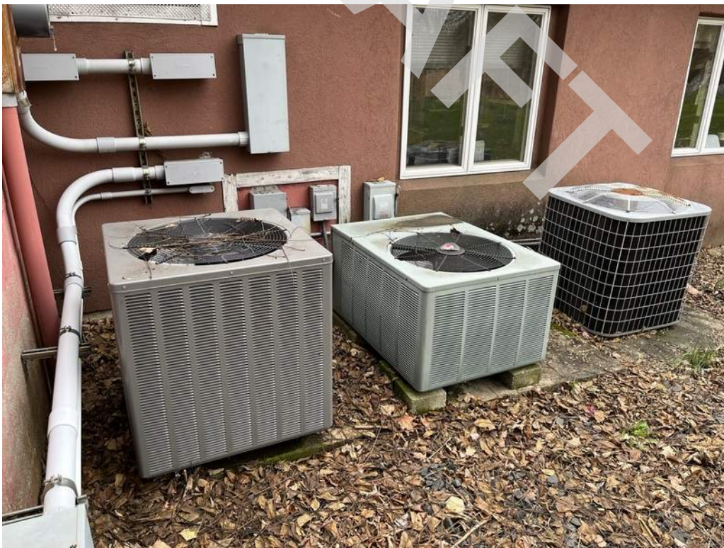
24 - Split system air conditioning units are located on the exterior and provide cooling to the building.
