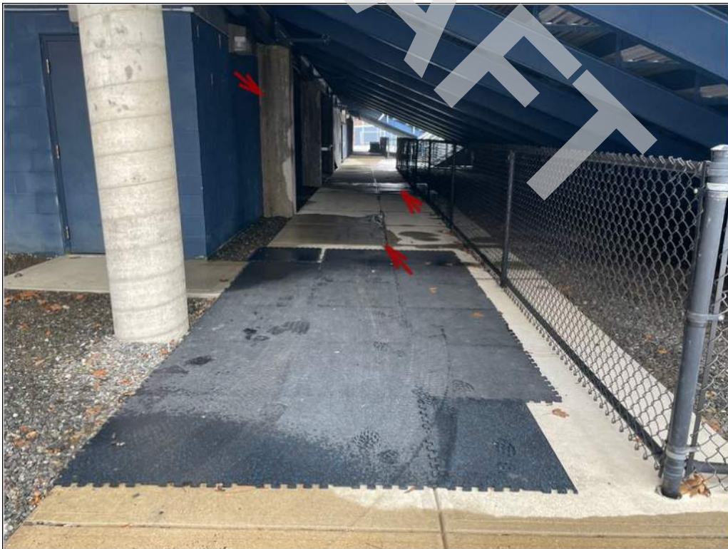
10 - Water from the grandstand is dripping along the team room CMU (Concrete Masonry Walls) and adjacent reinforced concrete walkway.
