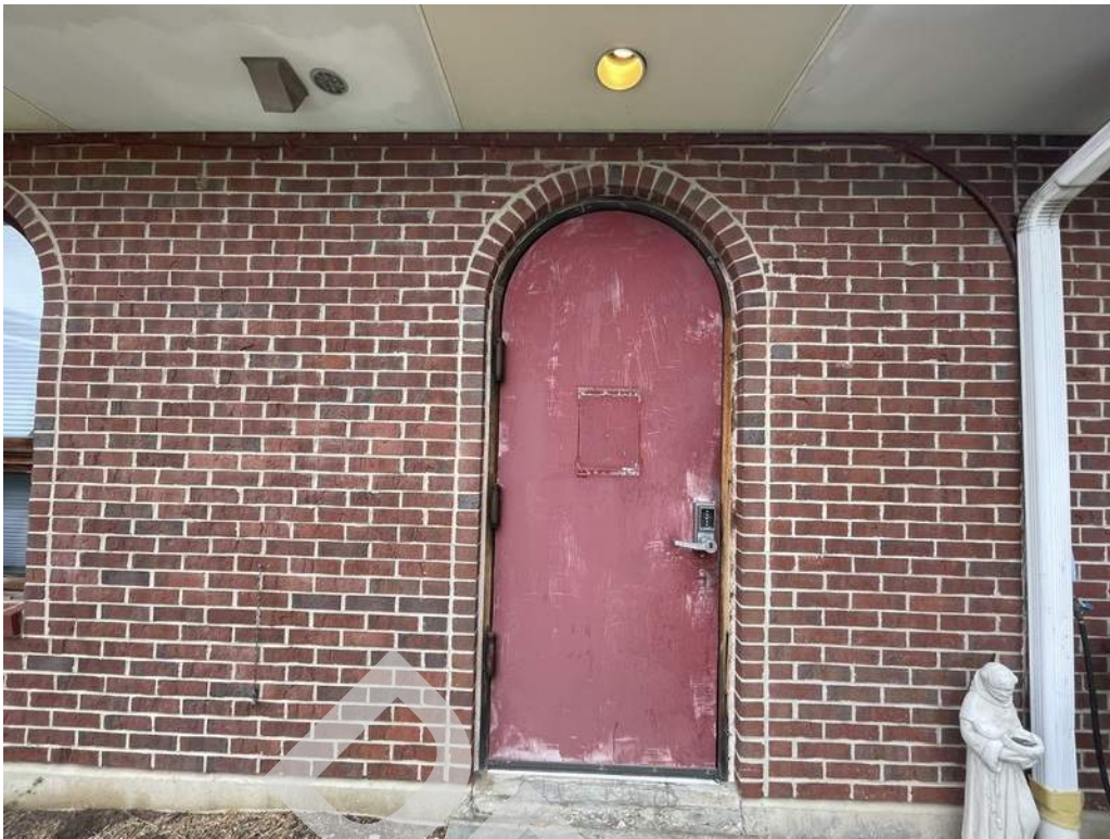
13 - Hollow metal door surface and finishes are in poor condition.
