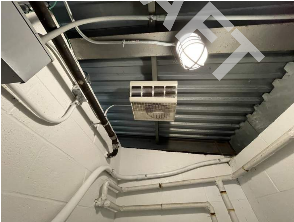
20 - Ceiling mounted electric unit heaters provide heating to the teams rooms.
