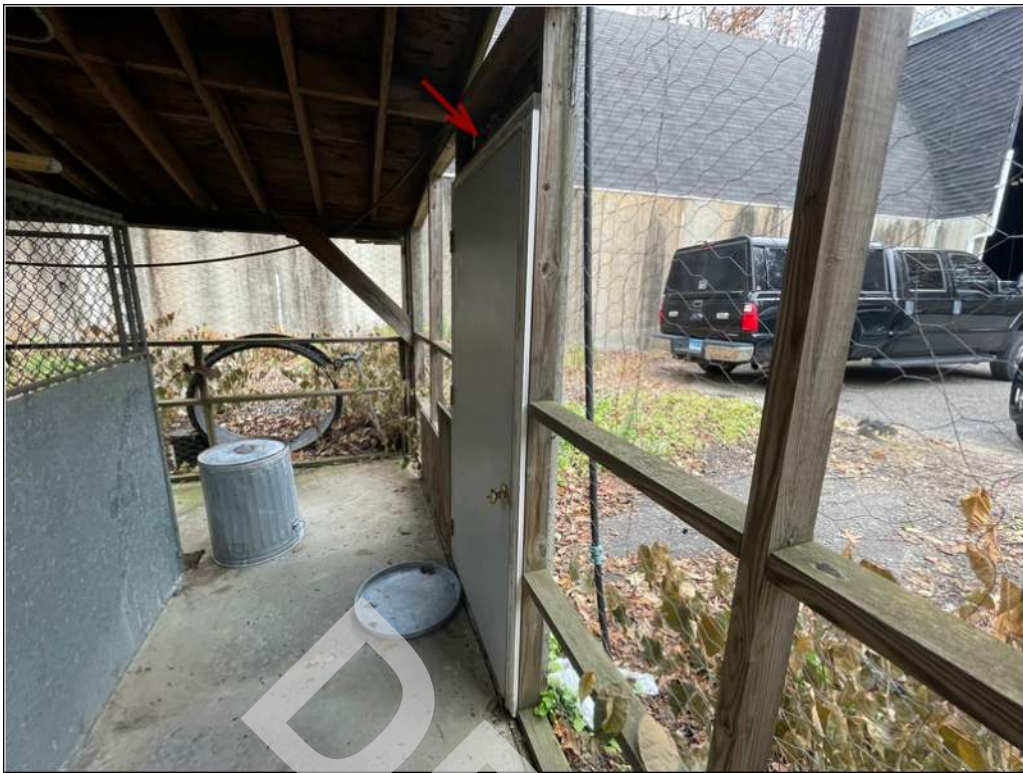
29 - Illuminated exit sign is not provided at the door exiting from the animal shelter kennel.
