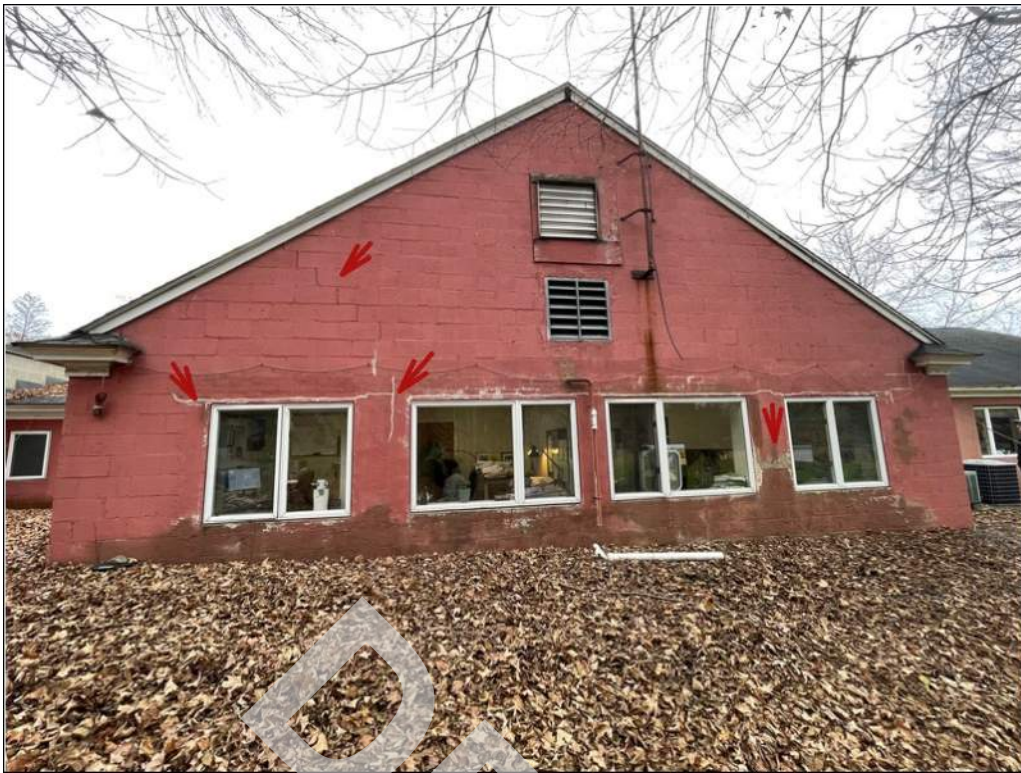
7 - Localized areas of the CMU (concrete masonry unit) facade have stepped cracking, cracked mortar joint and cracked units along the window lintel. Parging coat is peeling along the base CMU courses. Windows are in poor condition.
