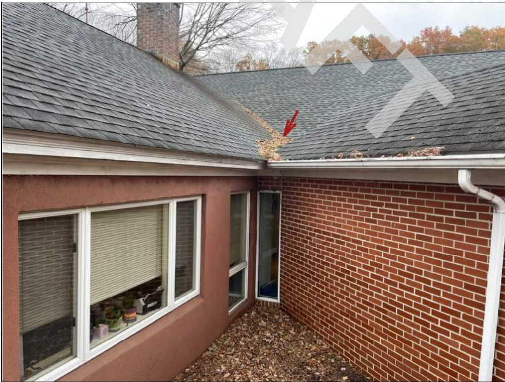
6 - Annex building roof consists of asphalt shingles. Interior areas below the roof valley had instances of water intrusion.
