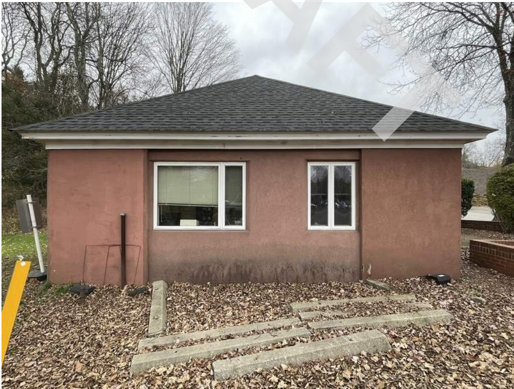
8 - Exterior surfaces along the façade have peeling paint finishes, debris accumulation, and organic growth stains.
