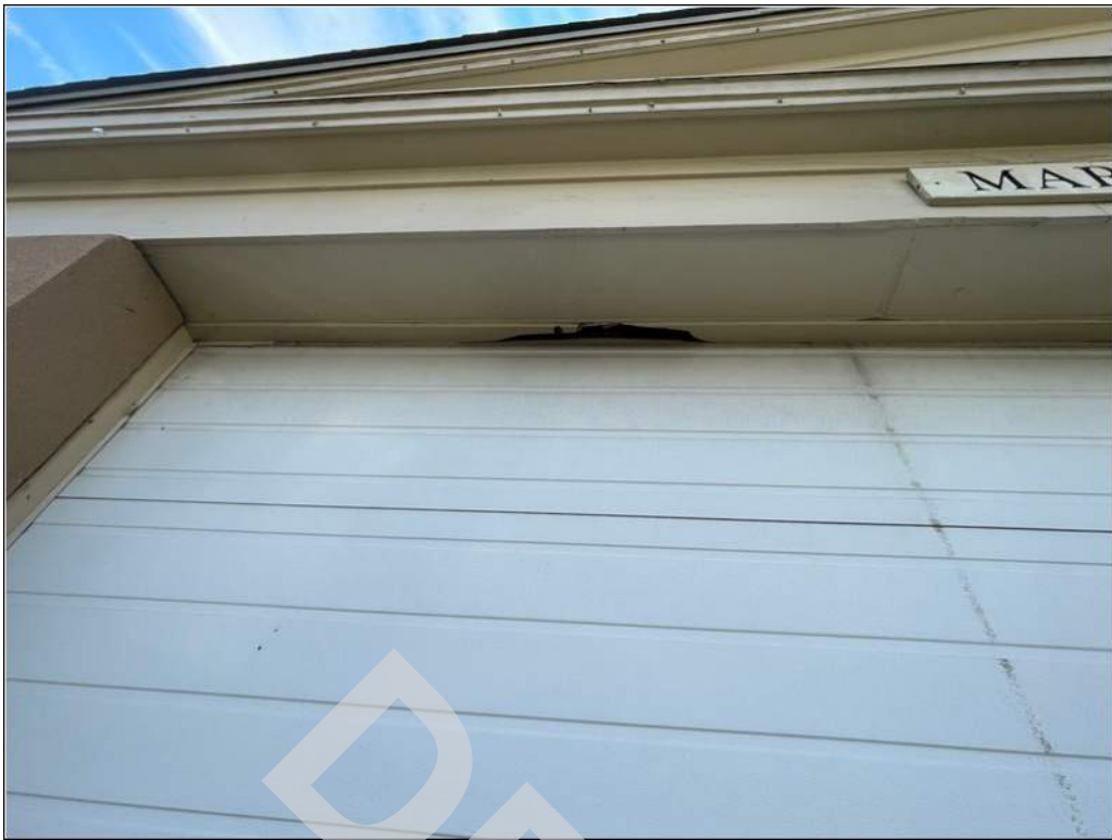
11 - Trim portions along the apparatus room door have broken.
