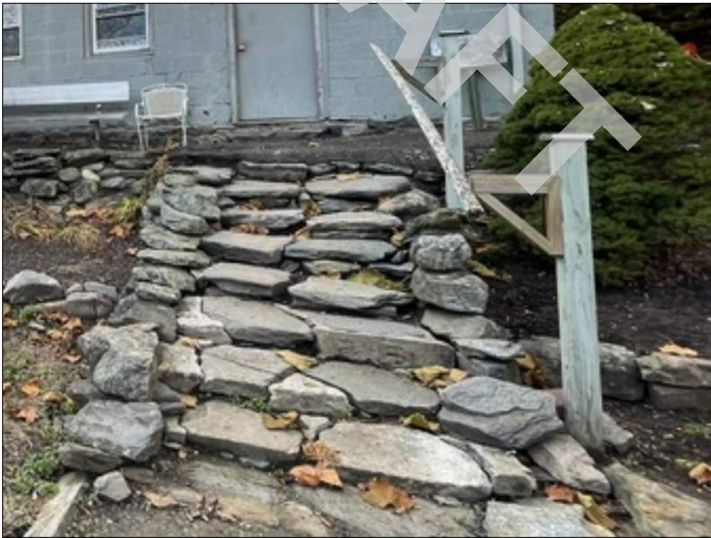
12 - Barn: Rock stair and landing are in poor condition; surfaces are uneven and a second handrail is not provided.
