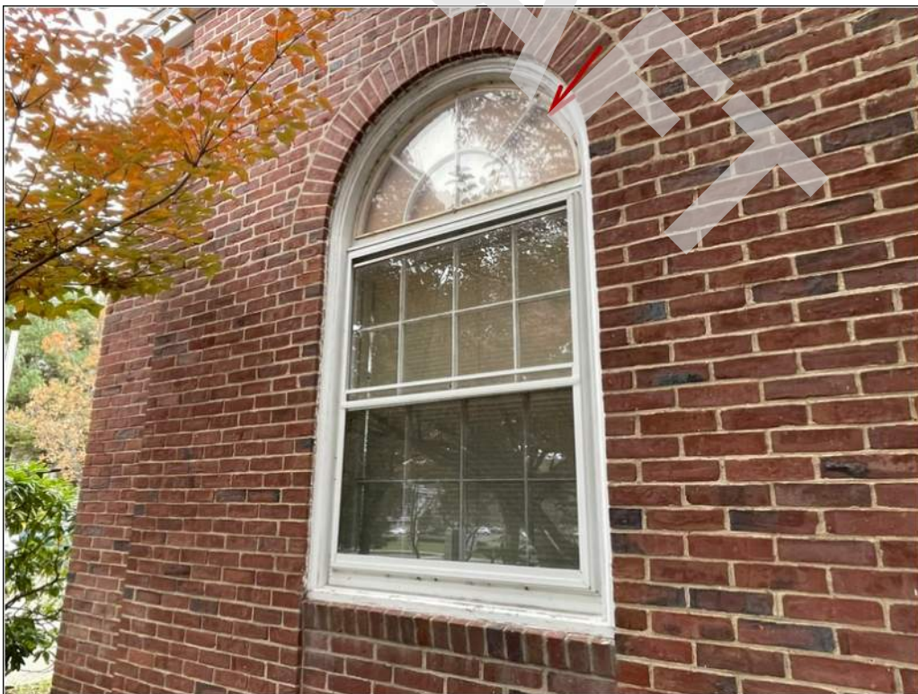
22 - Most of the window units have been covered with a plastic screen on the exterior.
