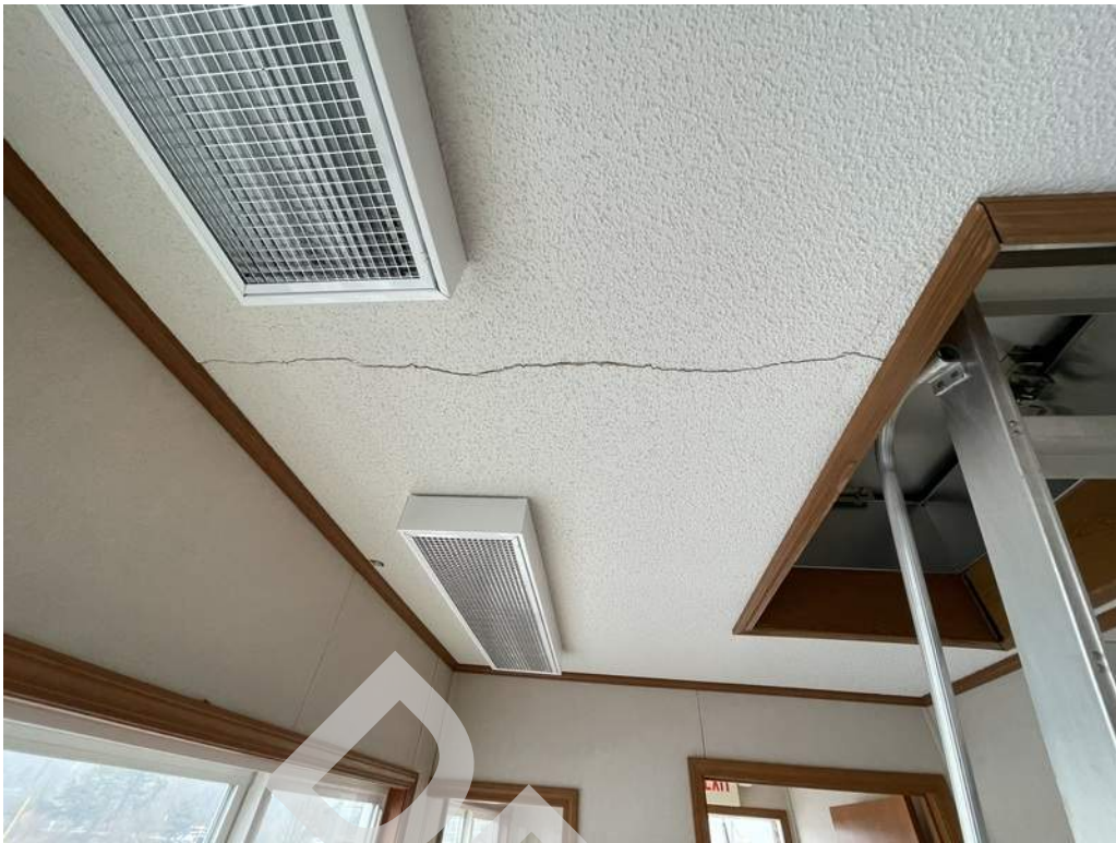
19 - Localized cracks along the press box ceiling have occurred.
