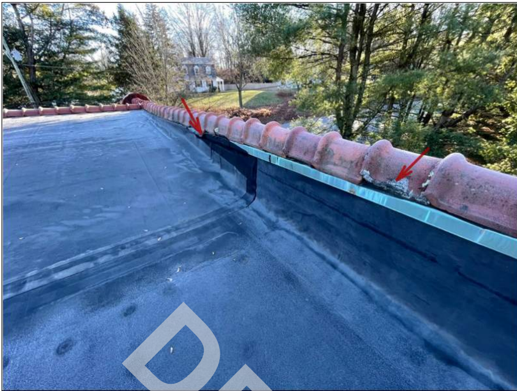
5 - Parapet coping consists of clay roof tiles with EPDM flashing and metal counterflashing. Clay roof tiles are in poor condition, some units are displaced and the EPDM parapet flashing is poorly installed.
