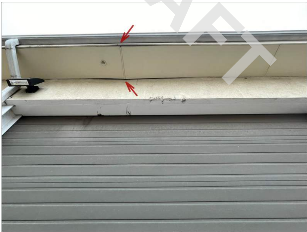
20 - Soffit and fascias are displacing.
