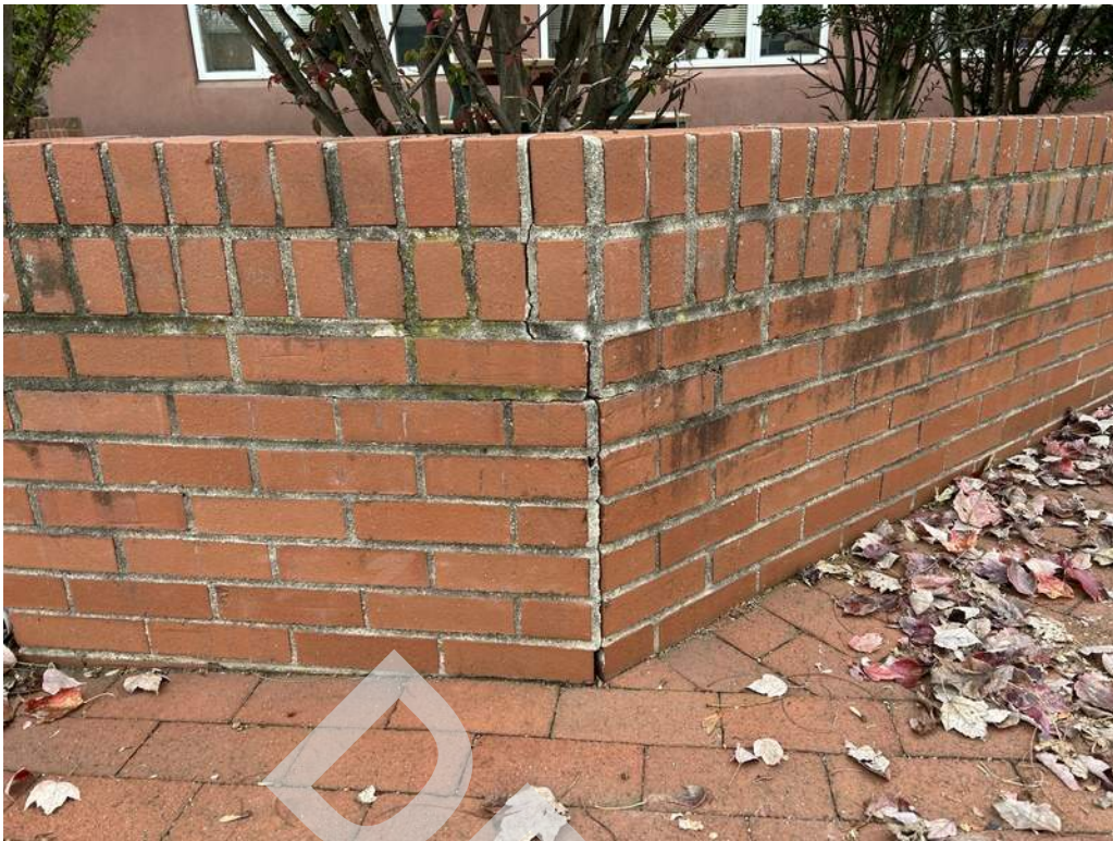
3 - Deteriorated mortar was observed at the brick garden wall, adjacent to the patio.
