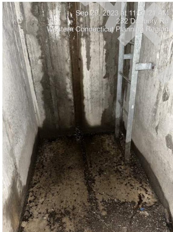
20 - Water intrusion at the bottom of the hatchway.
