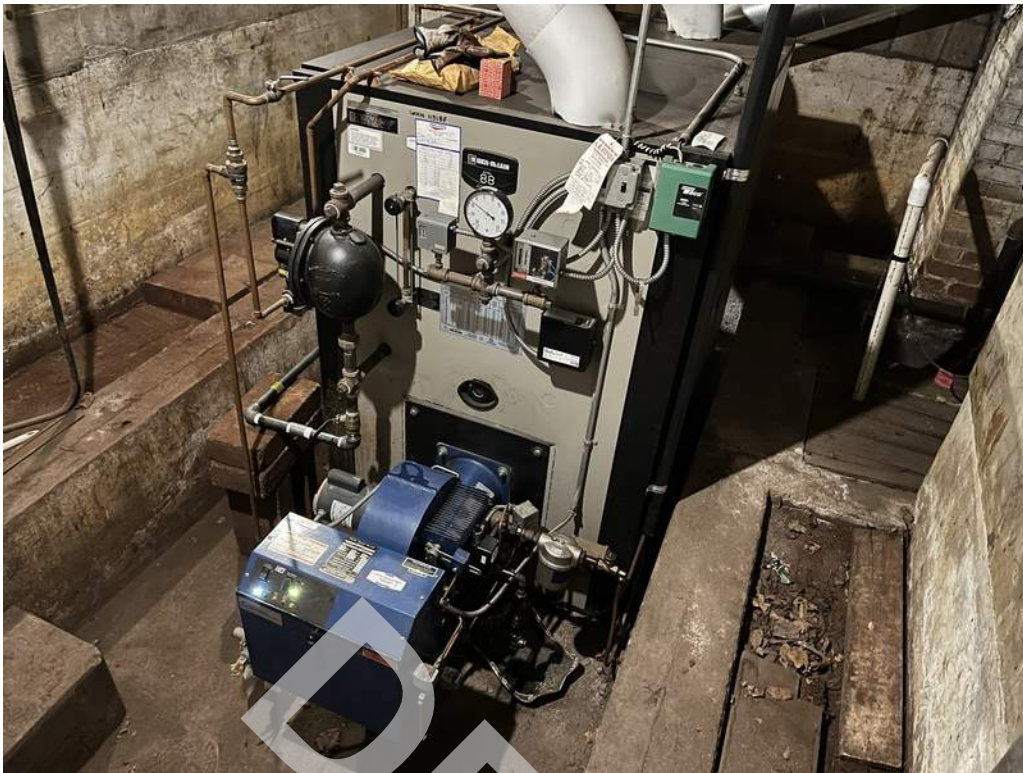
25 - An oil fired boiler located in the basement provides heating and domestic hot water throughout the building.
