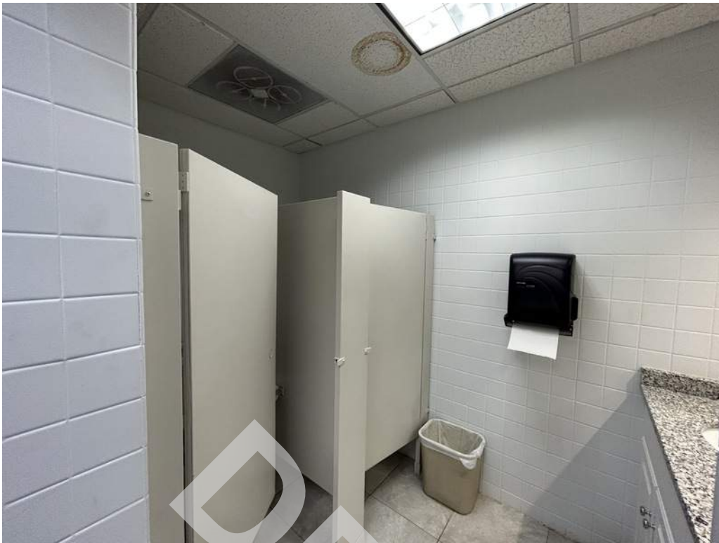
65 - An accessible stall is not provided at the multi-user restroom on the first floor.
