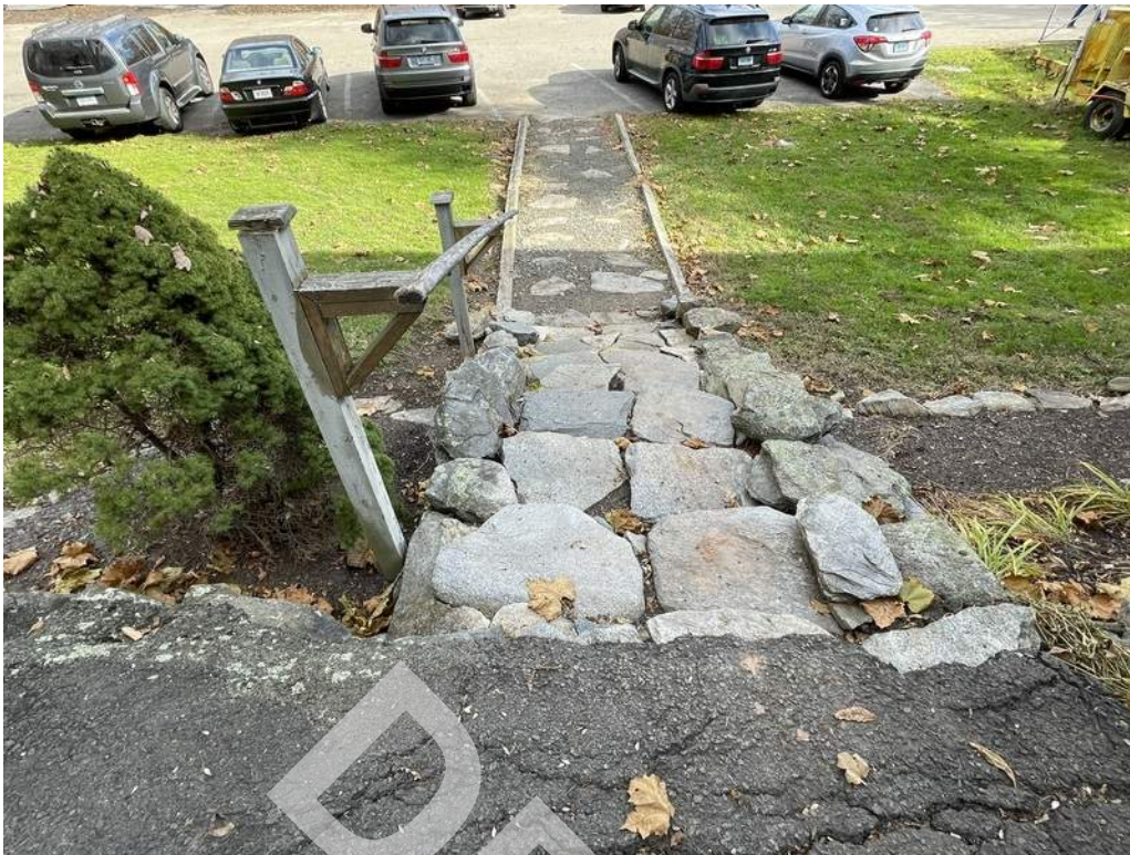
13 - Barn: Rock stair is uneven, and does not have a second handrail.
