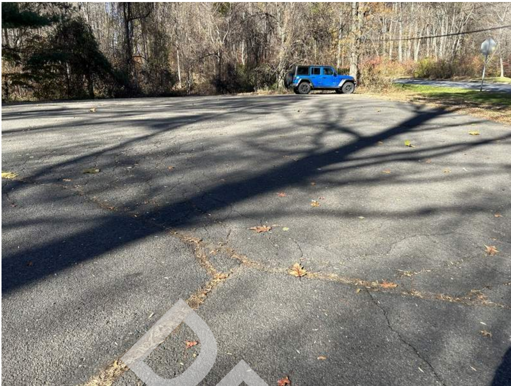
5 - Longitudinal and alligator cracking was observed at the second additional parking lot provided.
