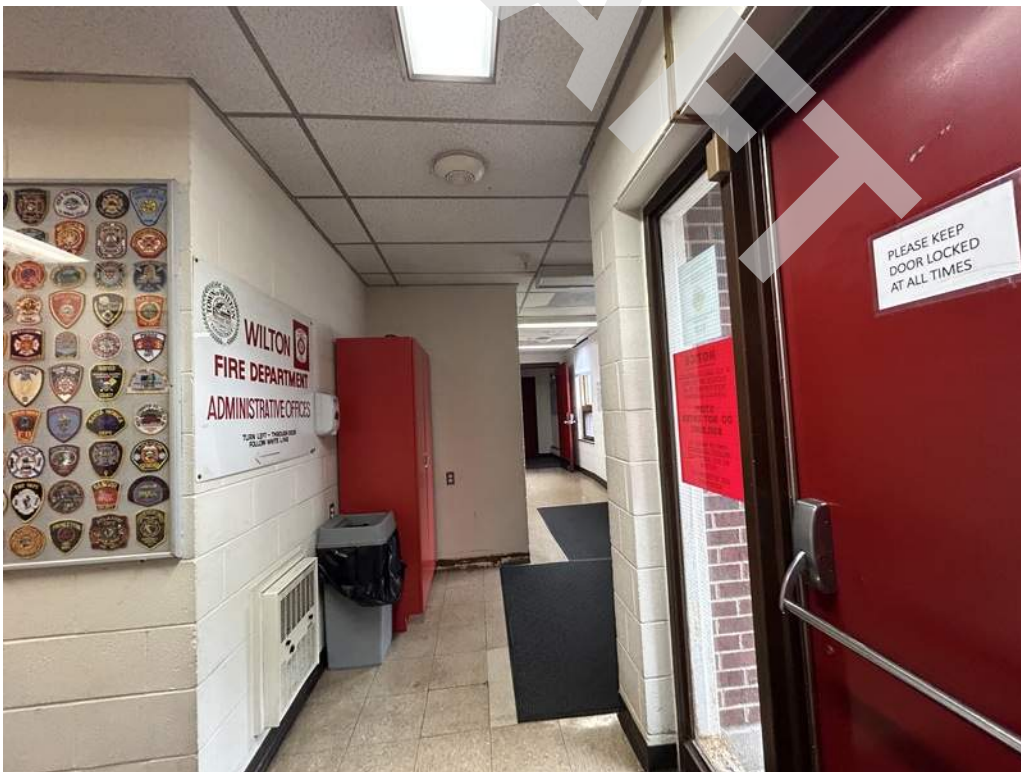
18 - Interior corridor finishes generally consist of painted gypsum walls boards or masonry, suspended ceilings with acoustic tiles, and vinyl composite tile floors. Chipped floor tiles and missing baseboards were observed.
