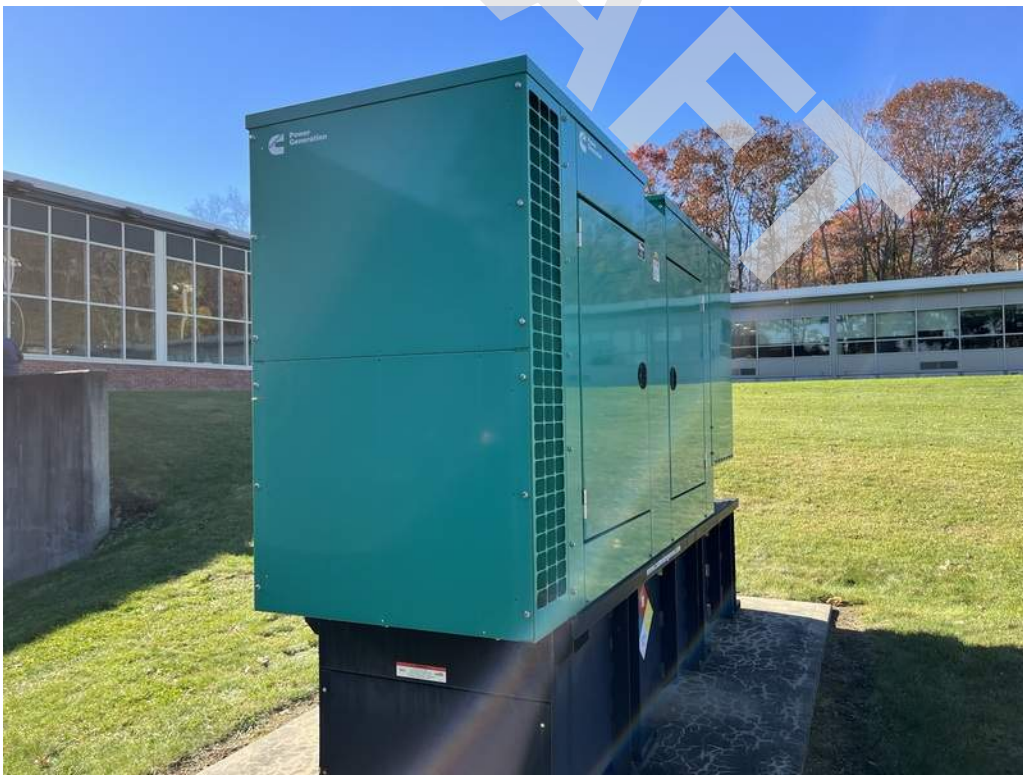
28 - A diesel-fired emergency generator located on the exterior of the building provides emergency power to the building.
