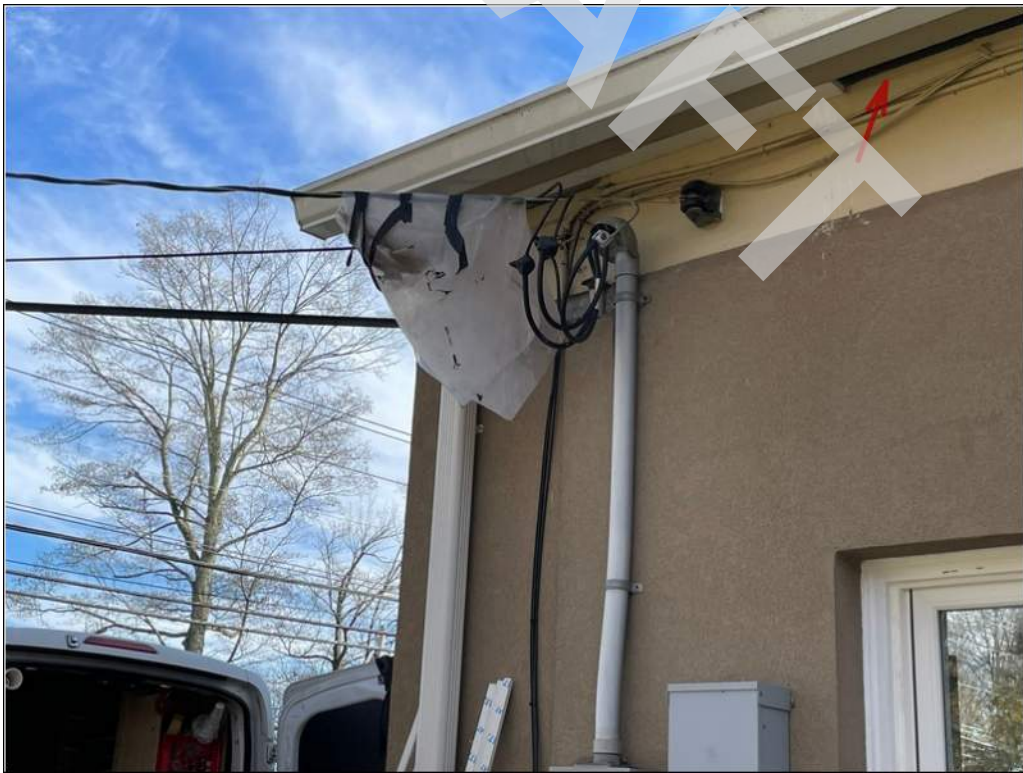
12 - Trim sections along the soffit are missing.
