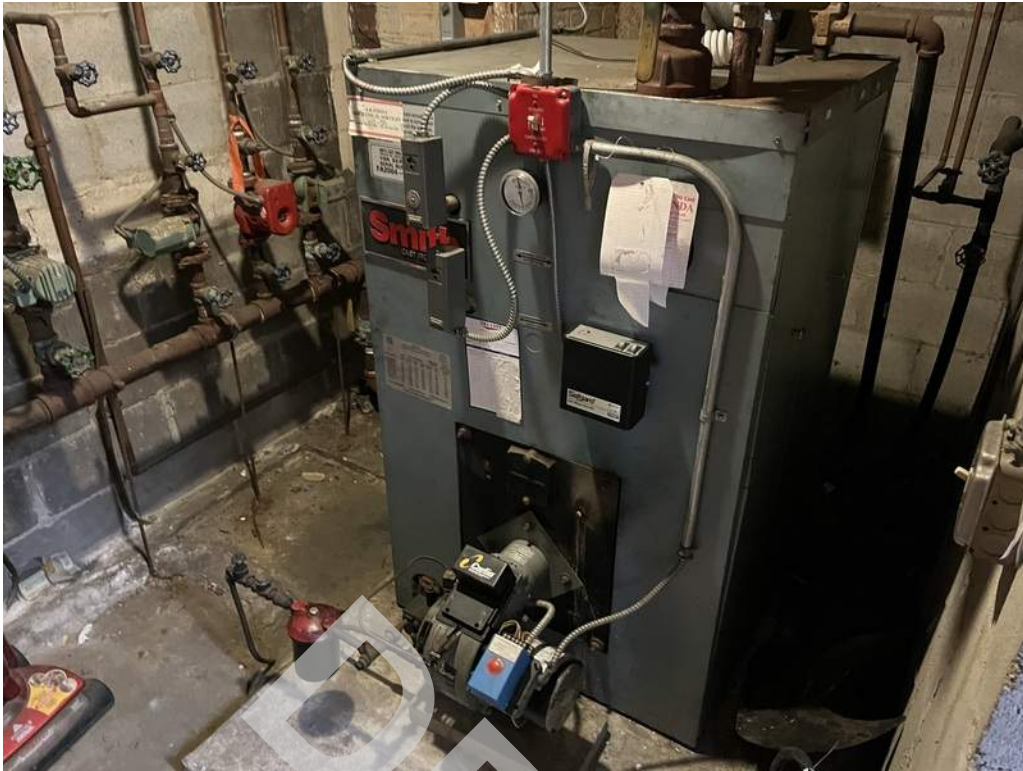
23 - An oil fired boiler located in a mechanical closet provides heating hot water throughout the building.
