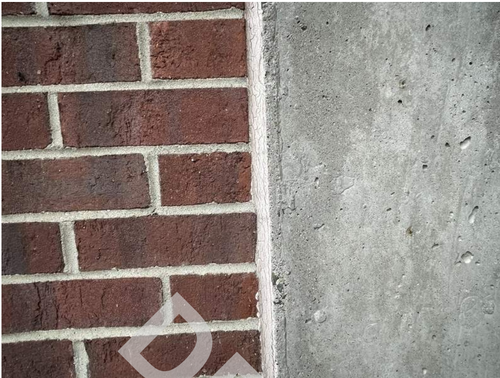
13 - The joint sealant between the brick masonry unit and concrete wall has failed.
