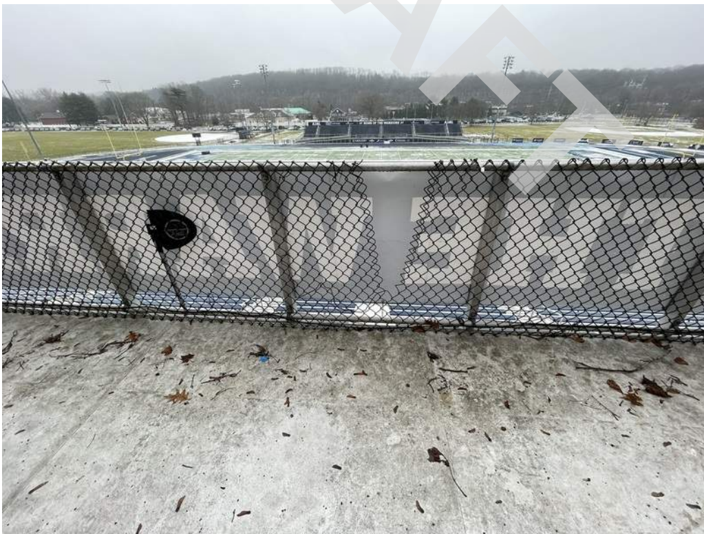
18 - A section of the chain link fence at the press room roof guardrail is broken.
