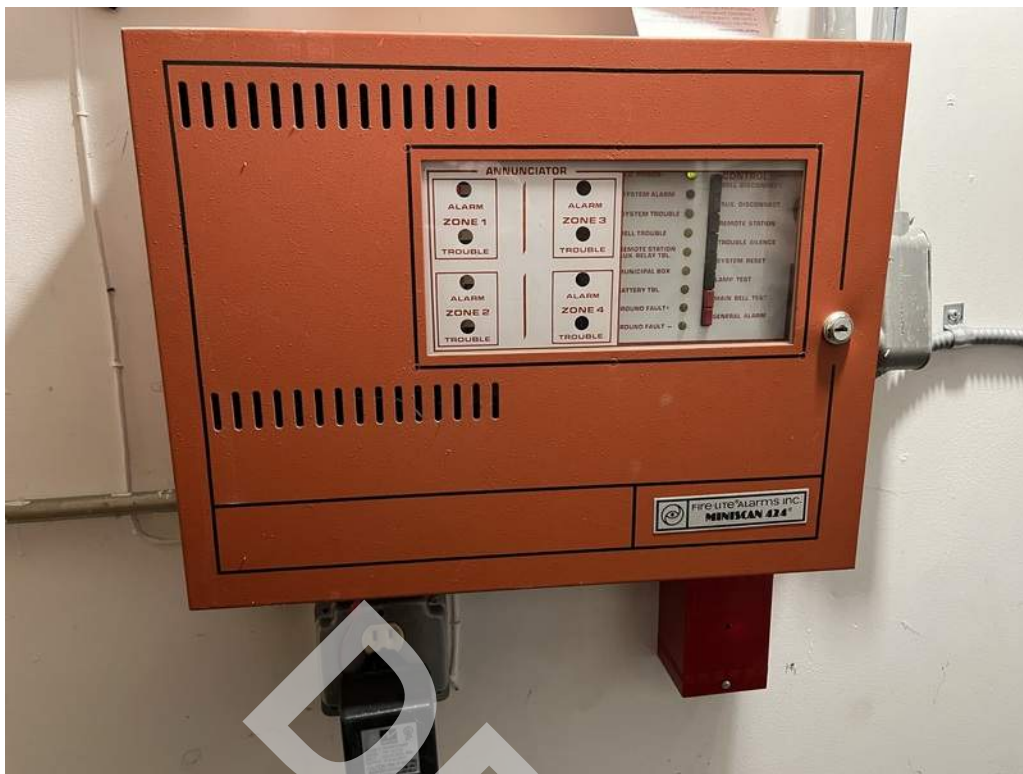
55 - The building is provided with a Miniscan 424 Fire Alarm Panel.
