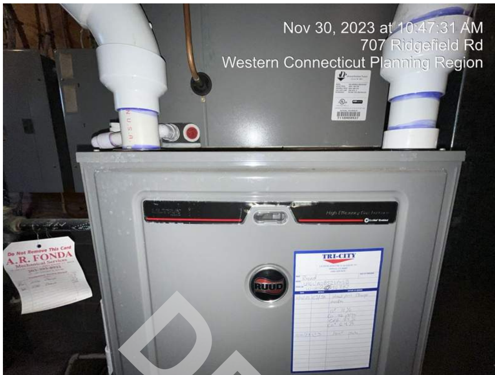
17 - Two propane fired furnaces located in the mechanical room provide heating to the building.
