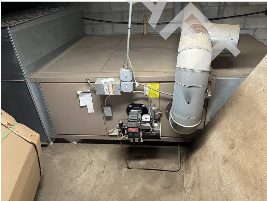
22 - Three oil fired furnaces located throughout the building provide heating throughout the building.
