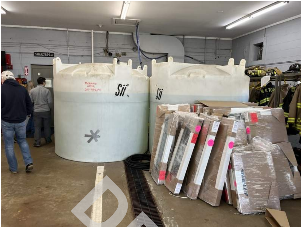
19 - Two water storage tanks located in the garage currently provide the building with domestic water.
