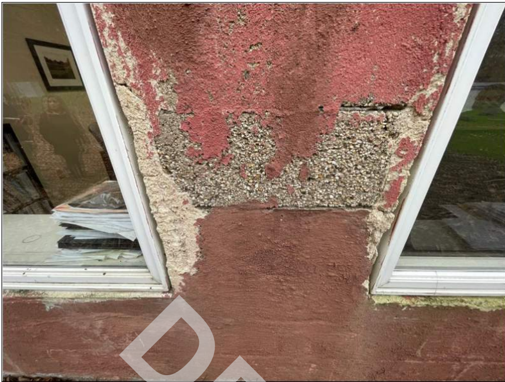
9 - CMU finishes and mortar joints along the facade are deteriorating.
