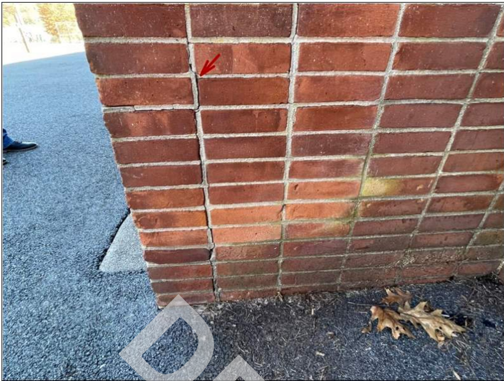
15 - Brick masonry unit mortar joints have cracked.
