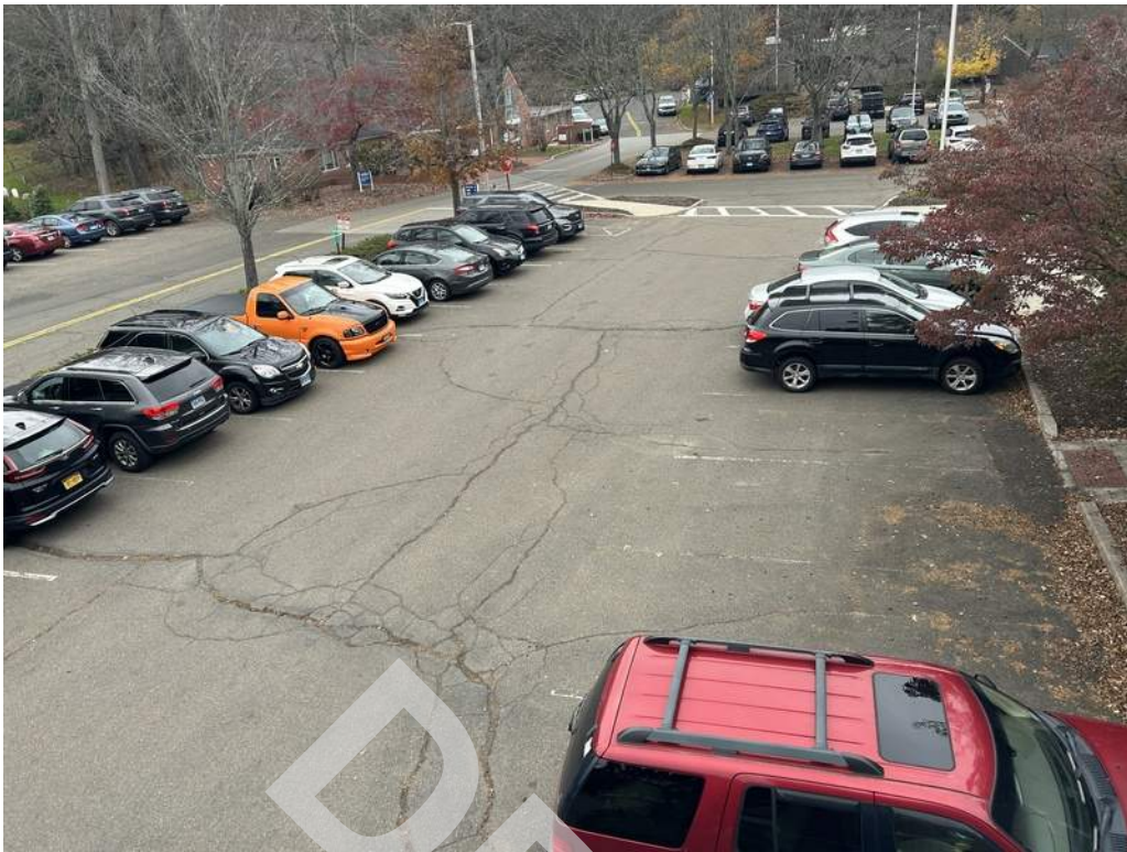
5 - Parking is provided along the north side of the building. Faded striping and alligator and longitudinal cracking was observed throughout the paved parking areas and drive lanes.
