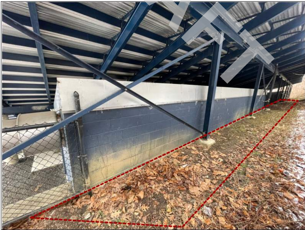
2 - Area adjacent to the building does not slope away from the retaining wall.
