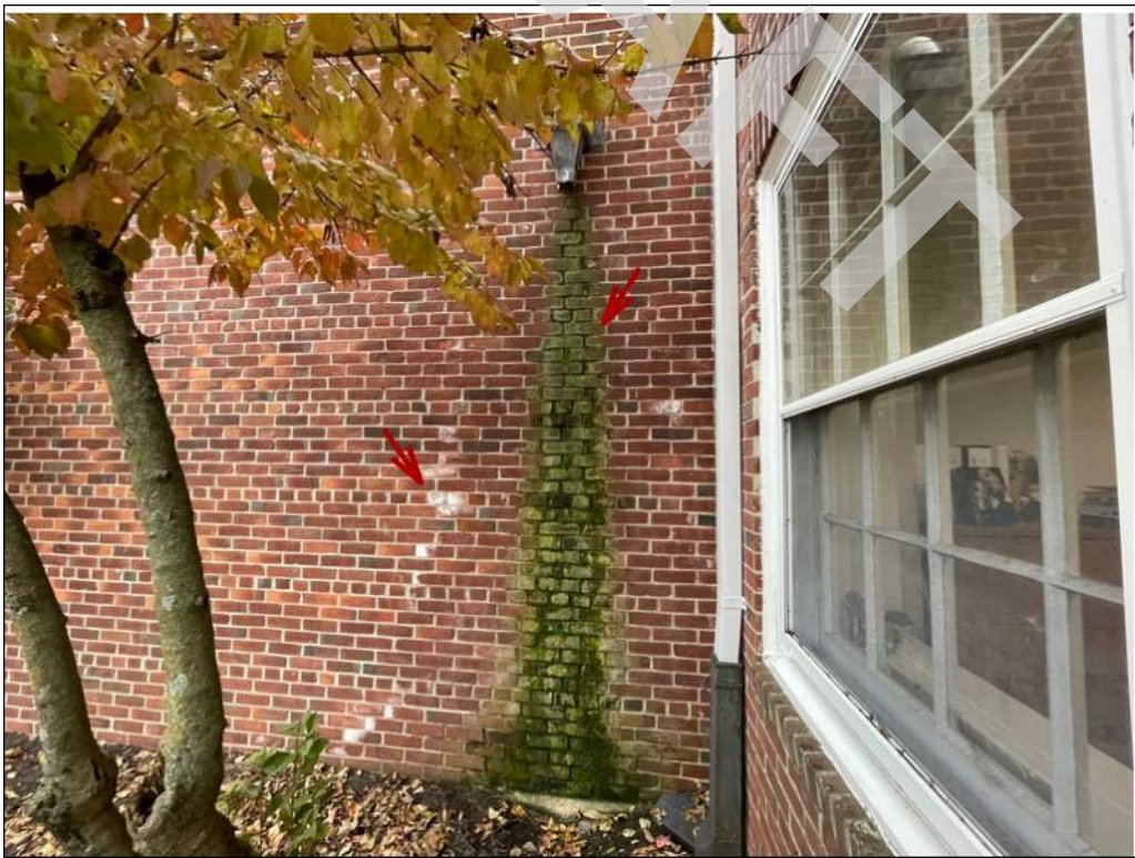
18 - Areas of the brick masonry facade have efflorescence and organic growth. Roof leader is missing.
