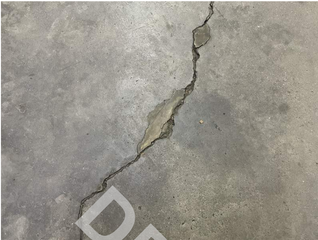
5 - Evidence of previously repaired cracks on the apparatus room slab on grade.
