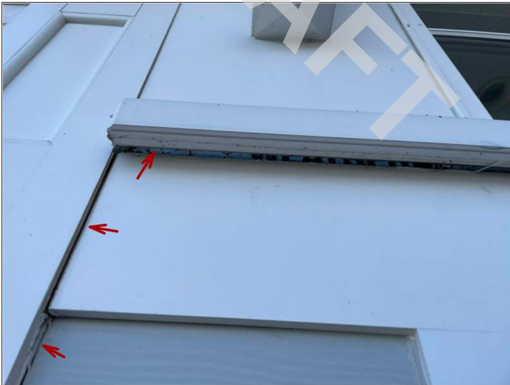
4 - Differential movement noted between fiber cement trim and panels throughout the building enclosure.
