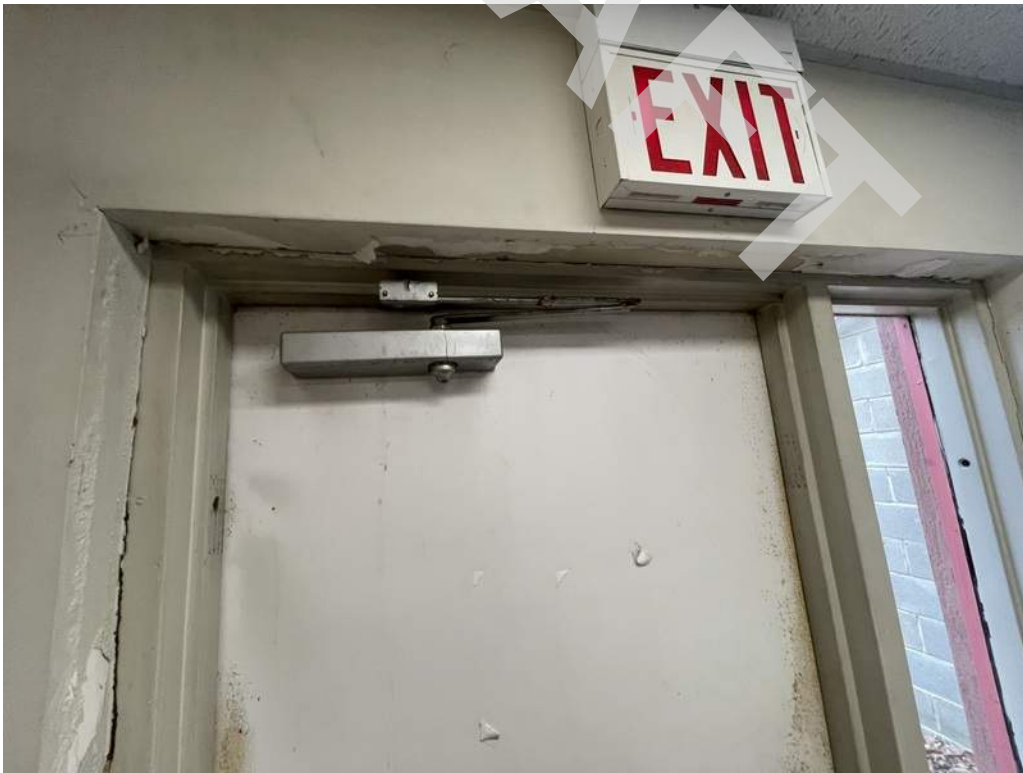
14 - Hollow metal egress door along the north facade is in poor condition.
