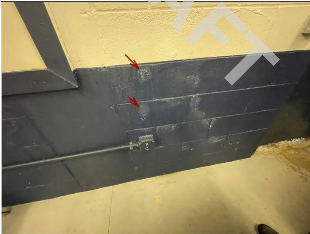
14 - Visible signs of moisture and efflorescence are spreading along the interior surface of the CMU enclosure.
