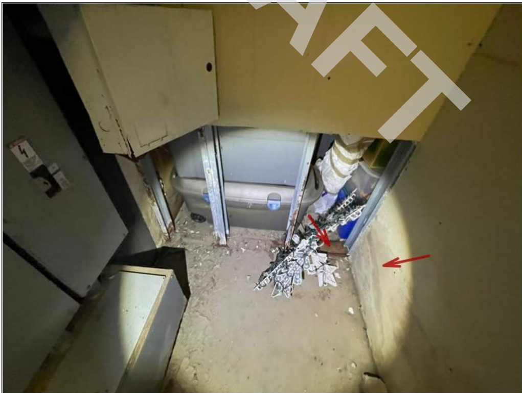
16 - Basement wall surfaces and wall framing metal components have water stains and corrosion due to water intrusion instances.
