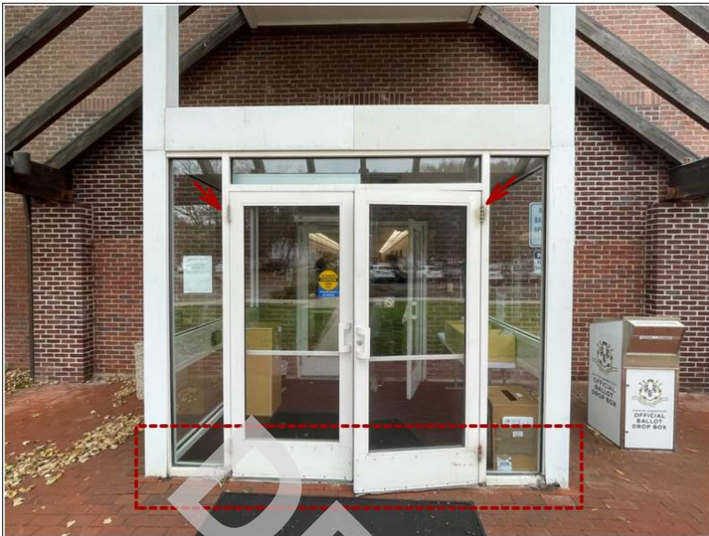
27 - The rear entrance storefront system has deteriorated. Damages include corrosion at the hinges and storefront framing along the base.
