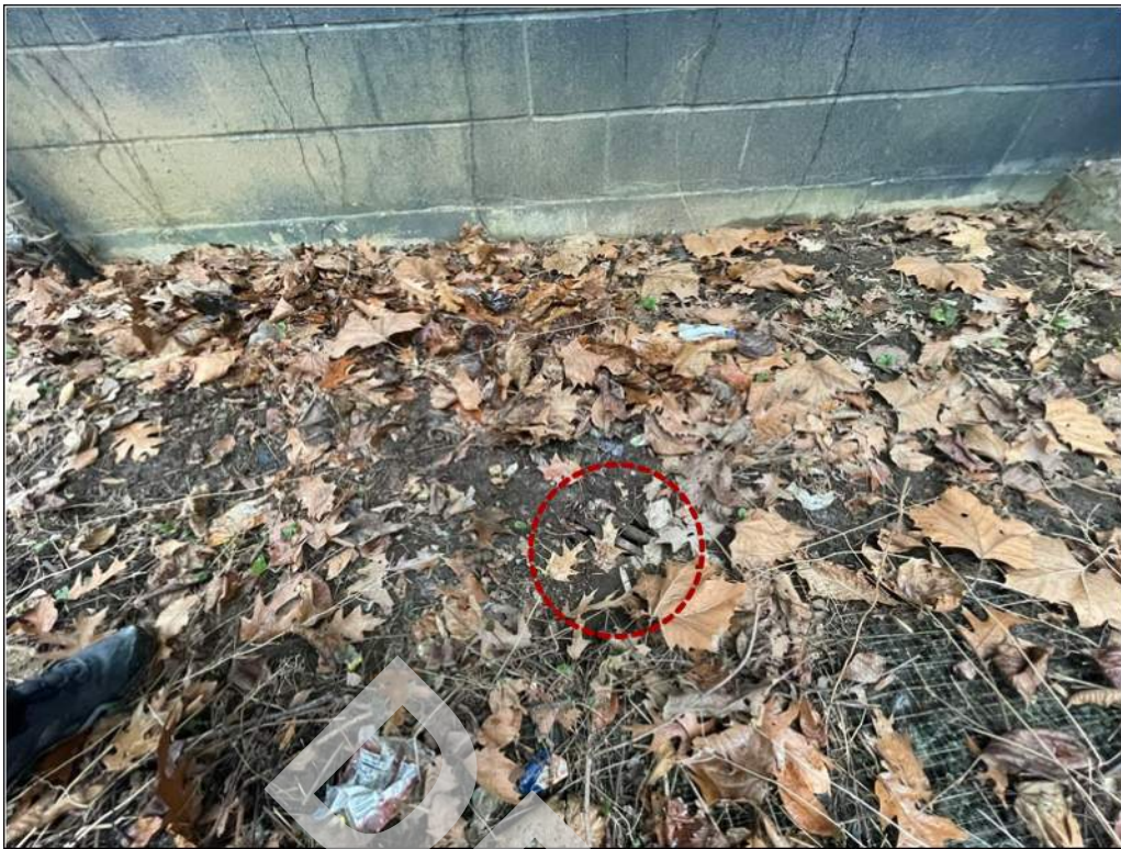
3 - Yard drains along the west wall of the team rooms are not readily accessible, obstructed by soil and debris.
