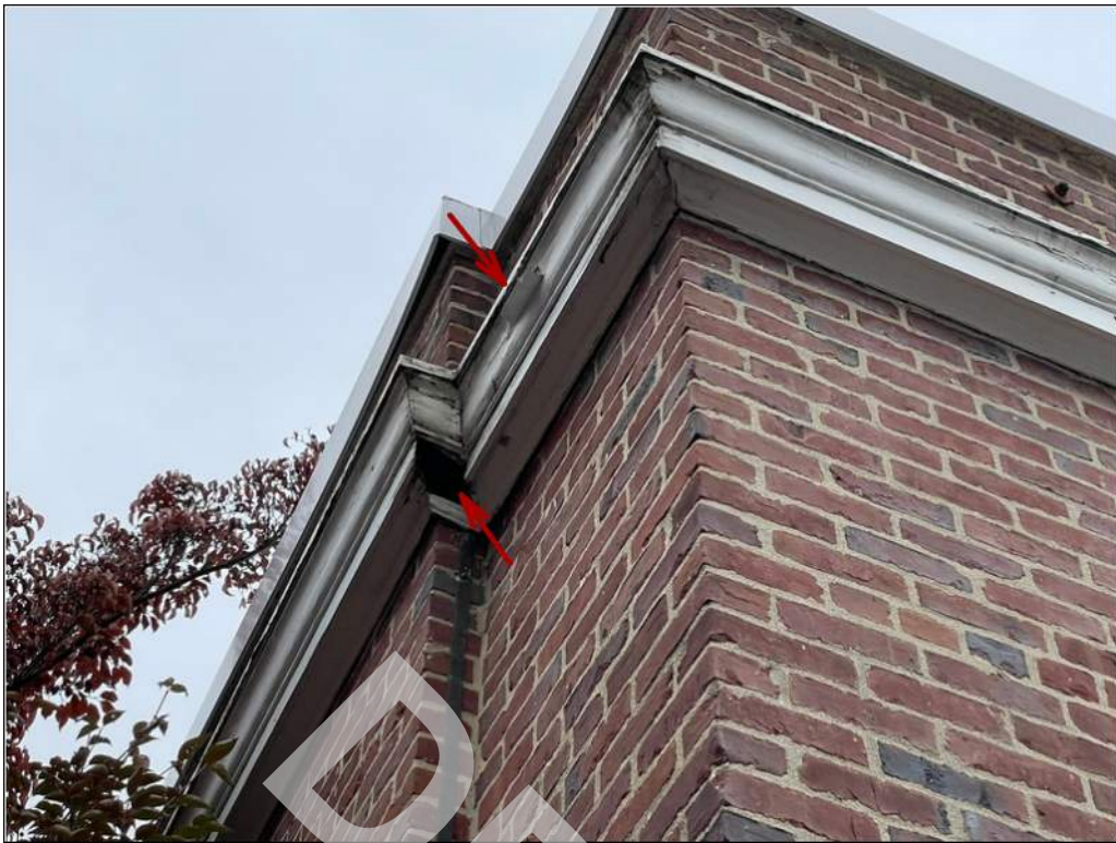
31 - Decorative wood trim cornices have rotted and have peeling finishes.
