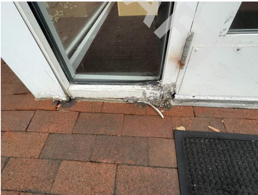
28 - Close up view of the corroded storefront framing components.
