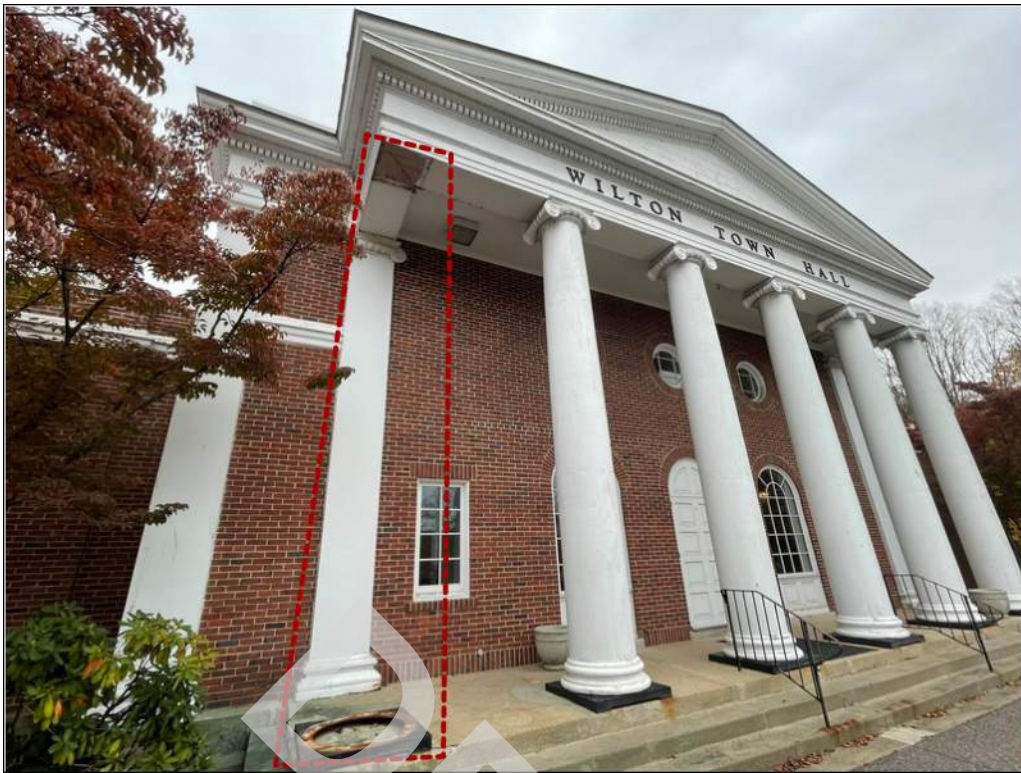
9 - Missing column along the front facade.
