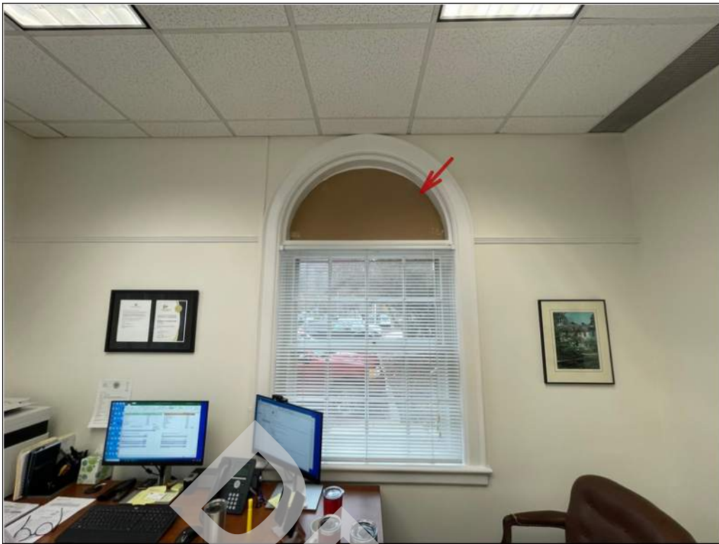
23 - A portion of the window units have been covered with cardboard.
