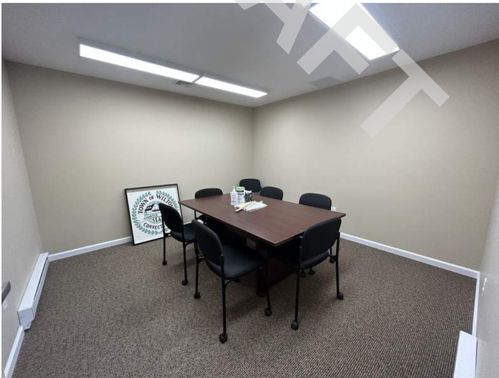
20 - Interior finishes at conference rooms consist of painted gypsum wall and ceiling boards and carpet floors.
