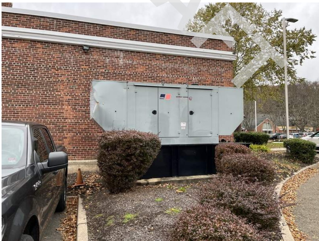
54 - A diesel-fired emergency generator located on the exterior of the building provides emergency power to the Town Hall and Annex buildings.
