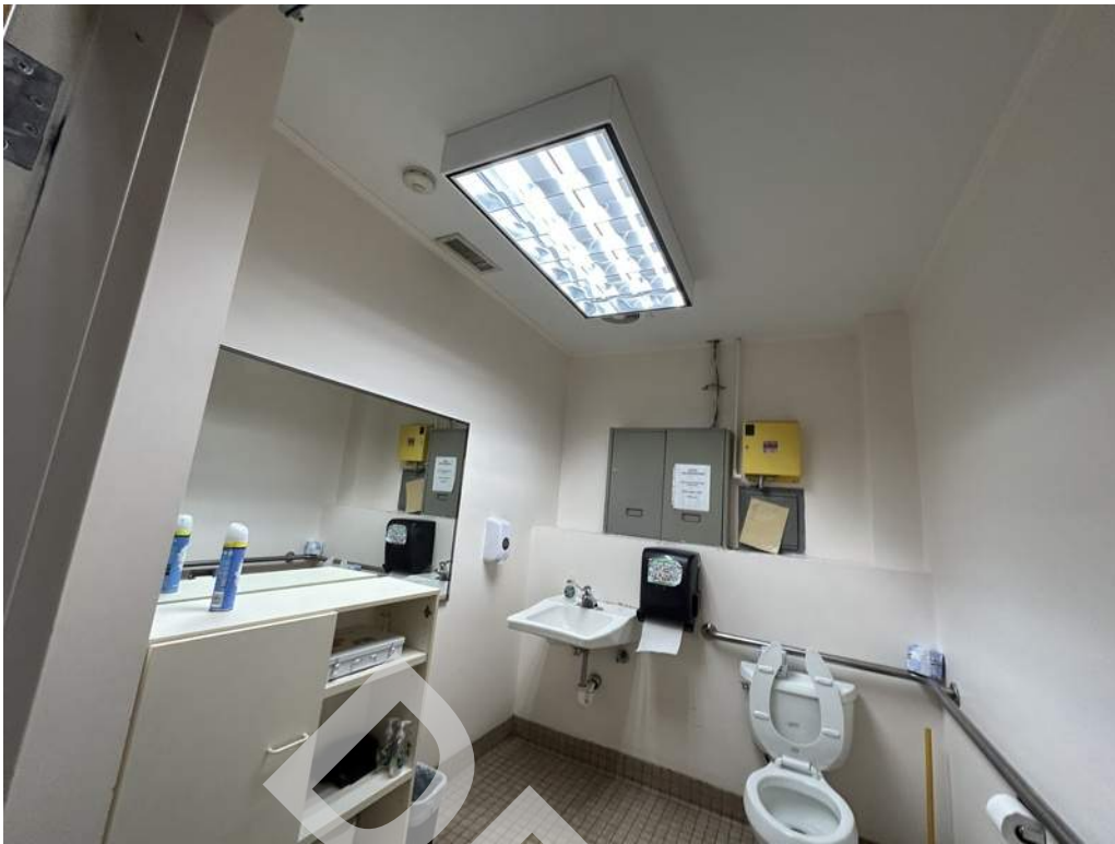
63 - The single user restroom on the ground floor was noted to have various non-compliant items. Items include center of toilet mounted above the the range tolerance from the side wall, inadequate sink depth and clear floor space, and missing scald guard protection beneath the lavatory.
