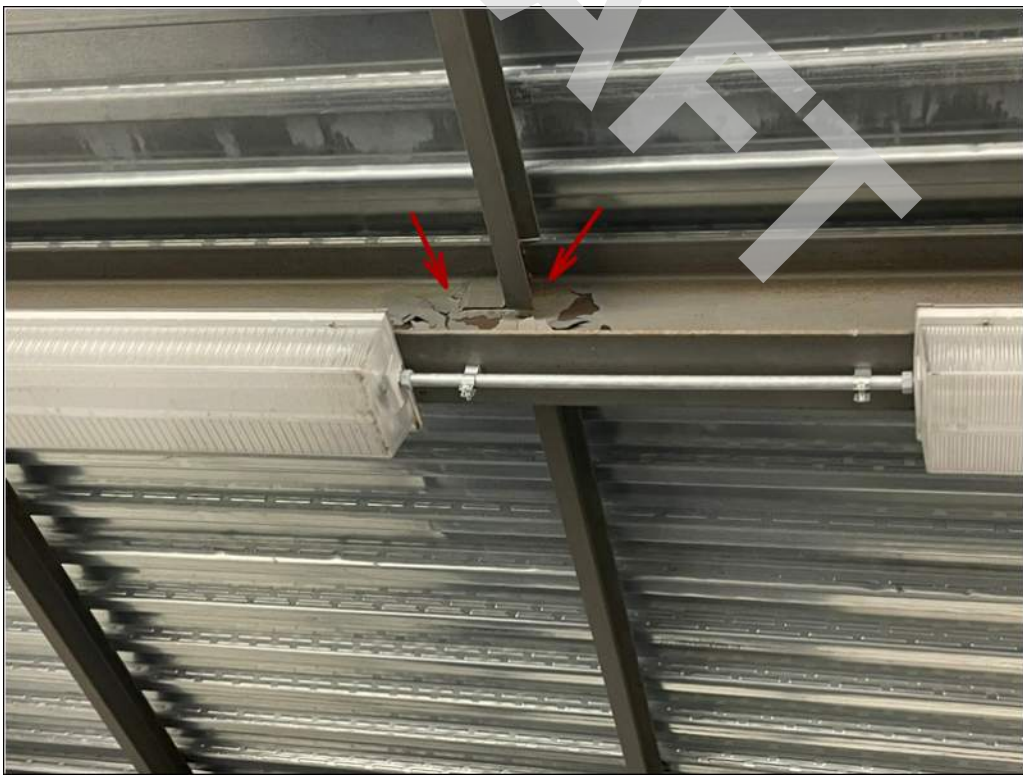
6 - Surface corrosion and peeling coating at the team rooms roof steel framing.
