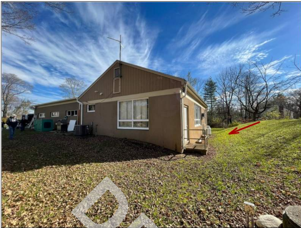
3 - Mound septic system is sloping towards the building's structure.
