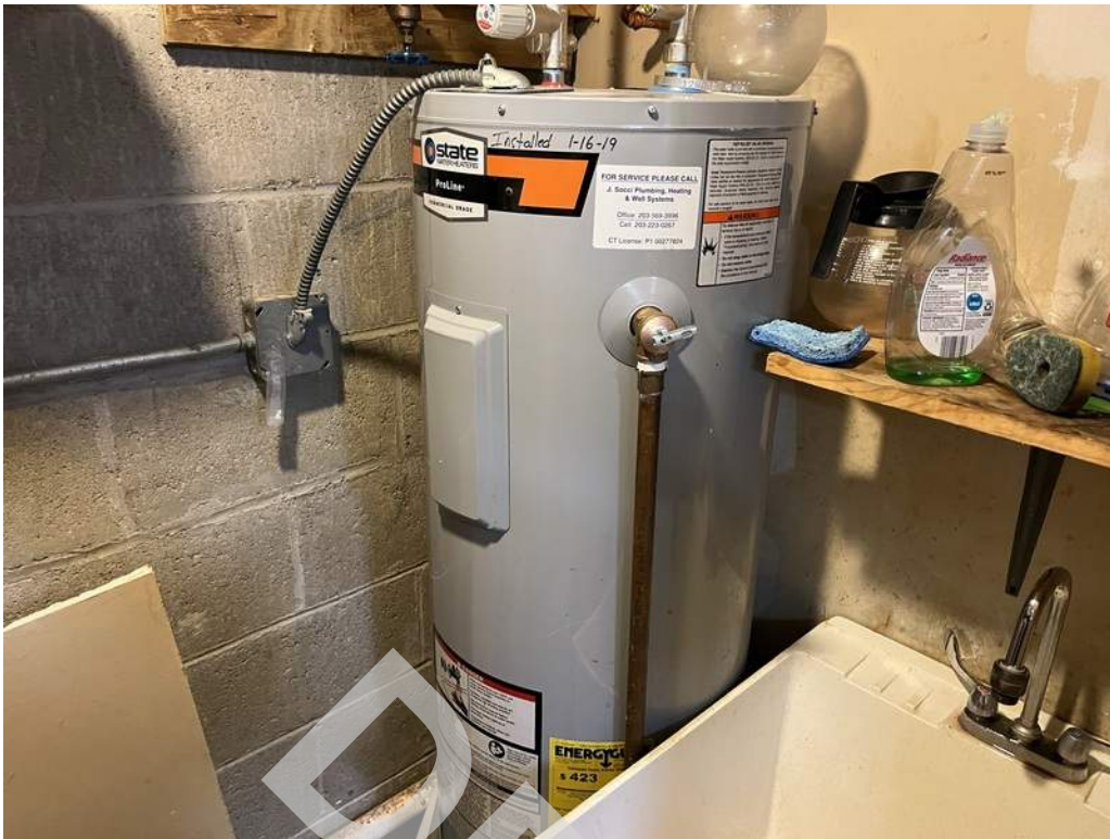
25 - An electric storage-type water heater is located in a closet and provides hot water throughout the building.
