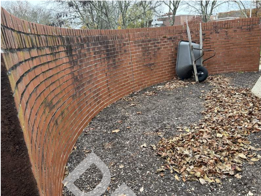
5 - Staining and deteriorated mortar was observed at the brick garden wall along the east façade.
