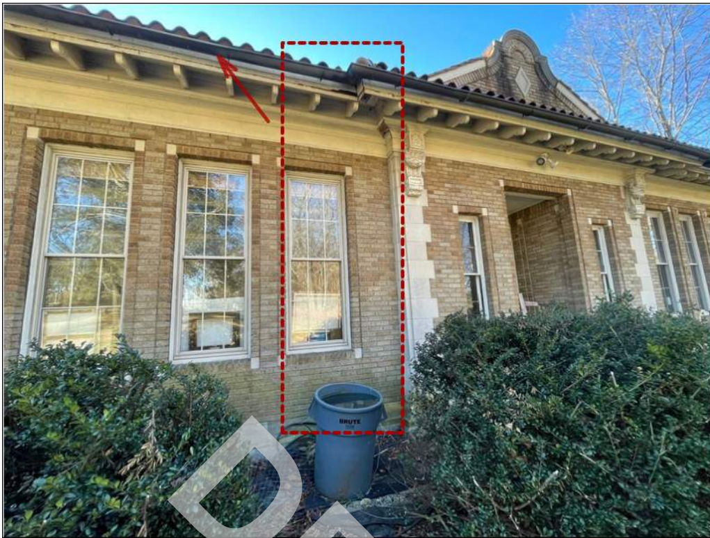
9 - Sections of the roof gutters are in poor condition and appear to be overflowing.
