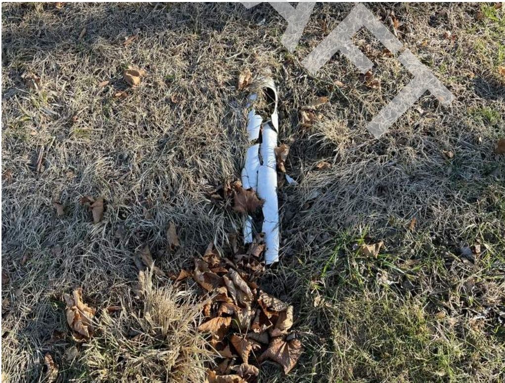
10 - Roof leader drain pipe extensions have failed.
