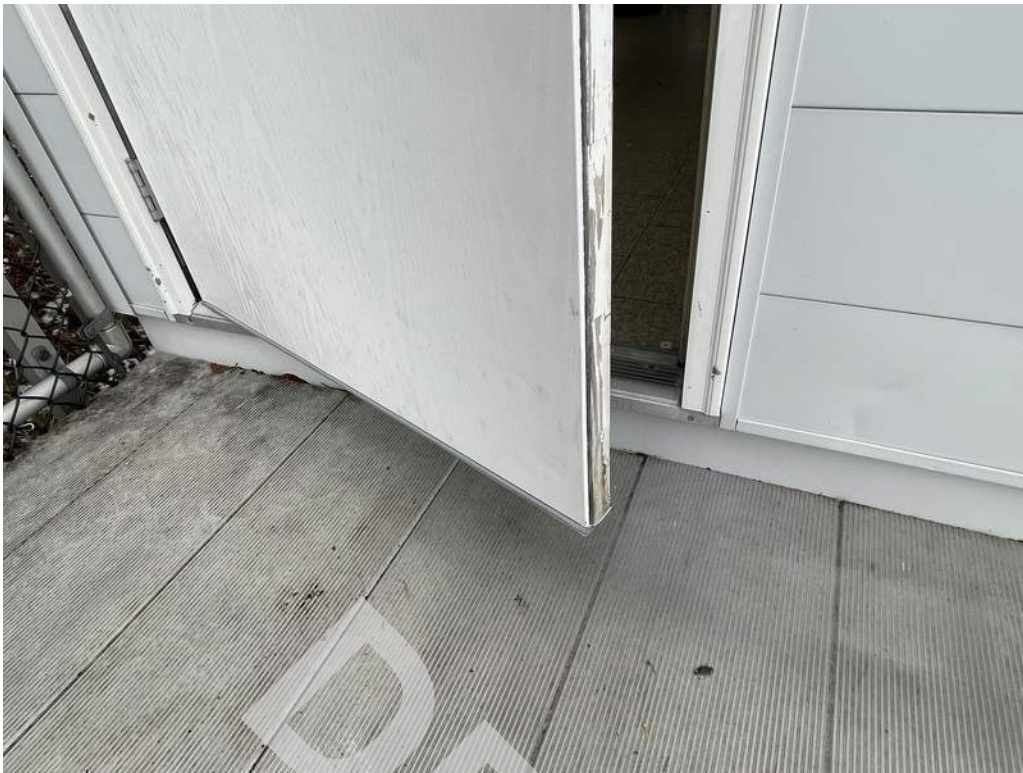
17 - Press box wood door surfaces are deteriorating.
