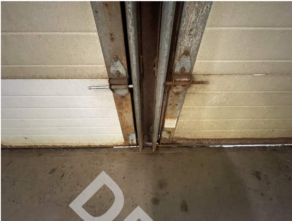
19 - Sectional overhead door metal components have corroded.
