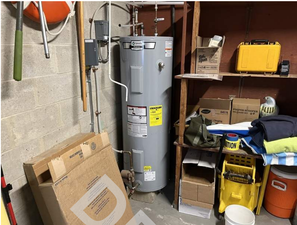
17 - The barn and restroom facility are each provided with an electric storage-type water heater which provides hot water to each building.
