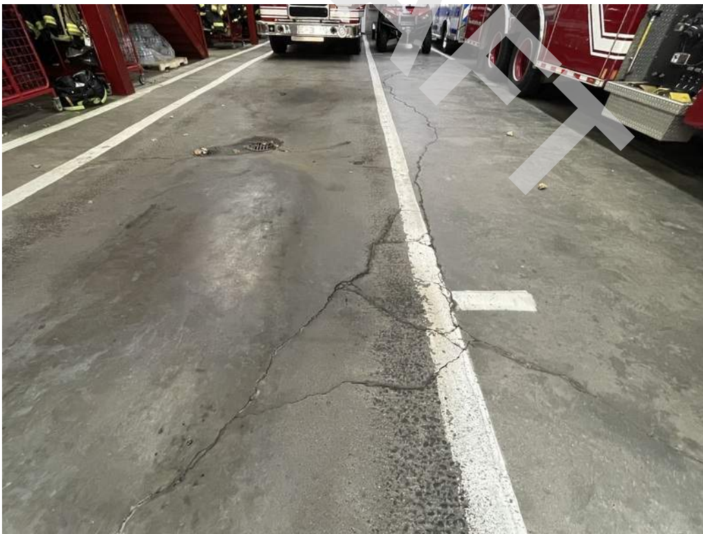
4 - The apparatus room slab on grade is uneven, has spalled, and has continuous cracks.
