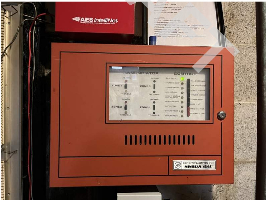
26 - The building is provided with a Miniscan 424 Fire Alarm Panel.
