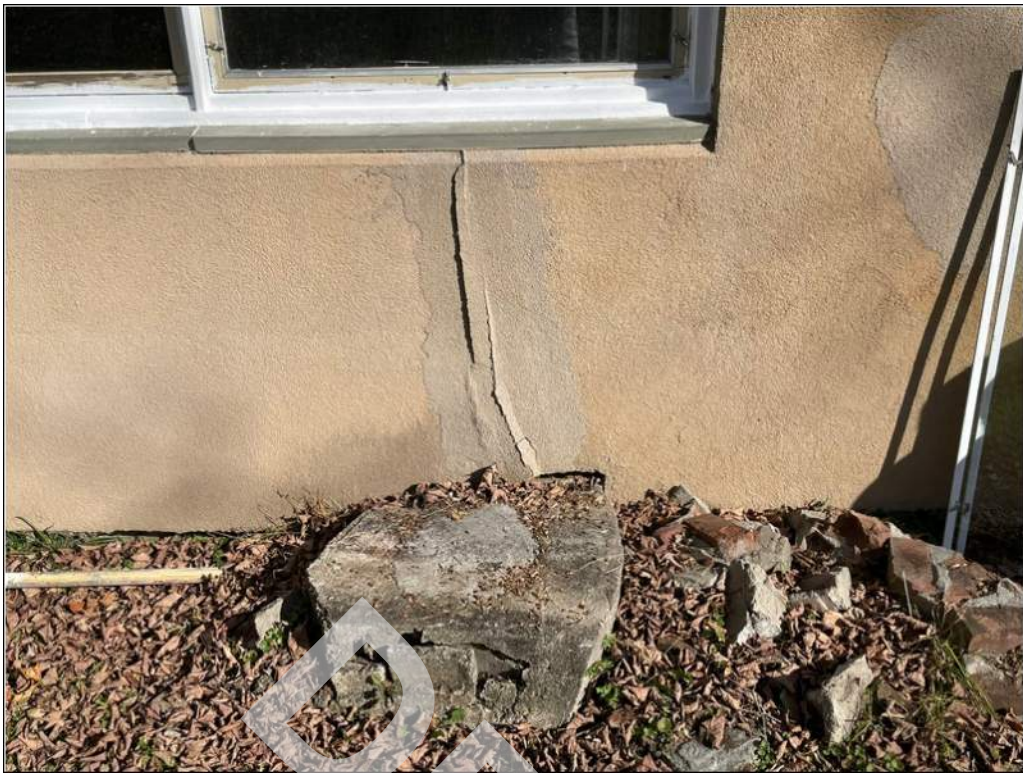
7 - Localized areas of the EIFS have cracked.
