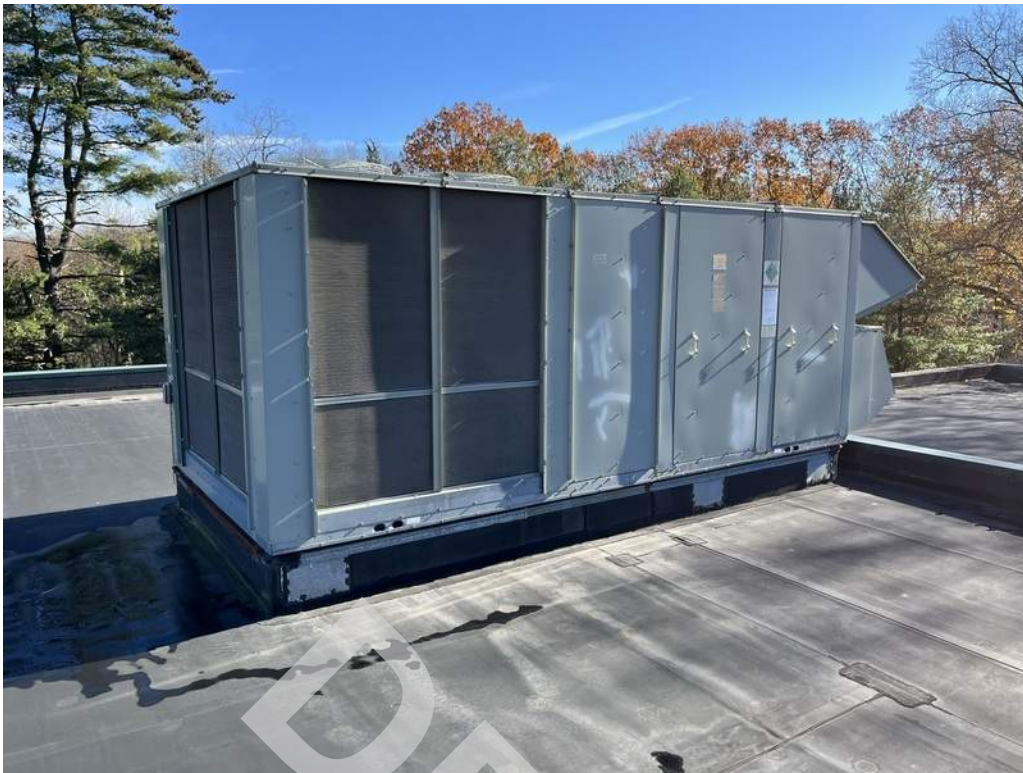
25 - Two rooftop packaged units (RTU) provide heating and cooling to portions of the building. One RTU is natural gas fired and the other is provided with a hot water coil that is fed from the boilers.
