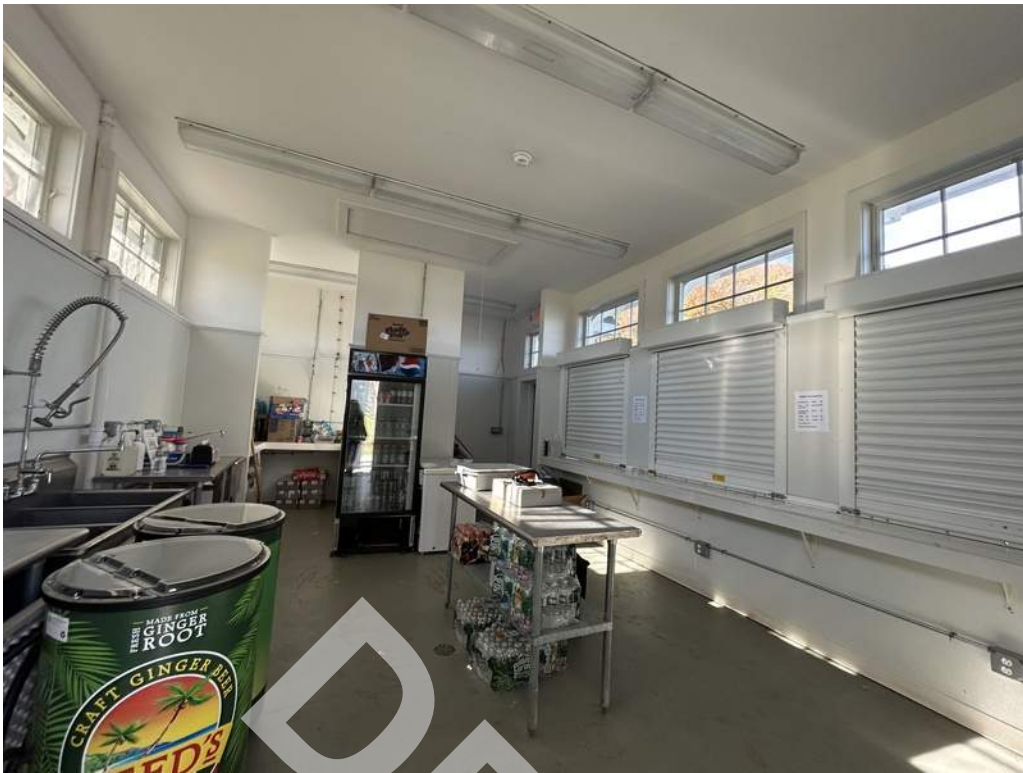
7 - Interior kitchen finishes consist of painted gypsum board ceiling and boards and painted concrete slabs.
