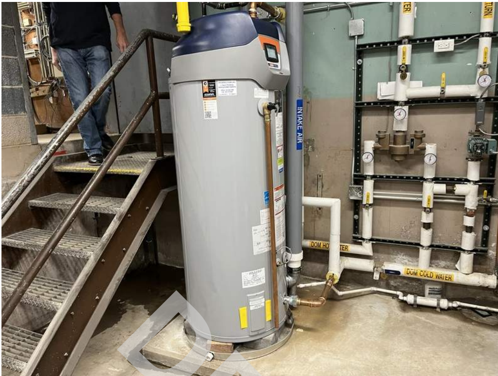
27 - A natural gas fired storage-type water heater is located in the lower level and provides hot water throughout the building.
