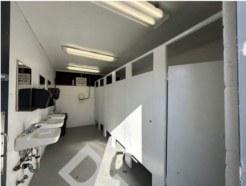
15 - Restrooms: Interior finishes consist of painted masonry walls, painted gypsum ceiling boards, and painted slabs.
