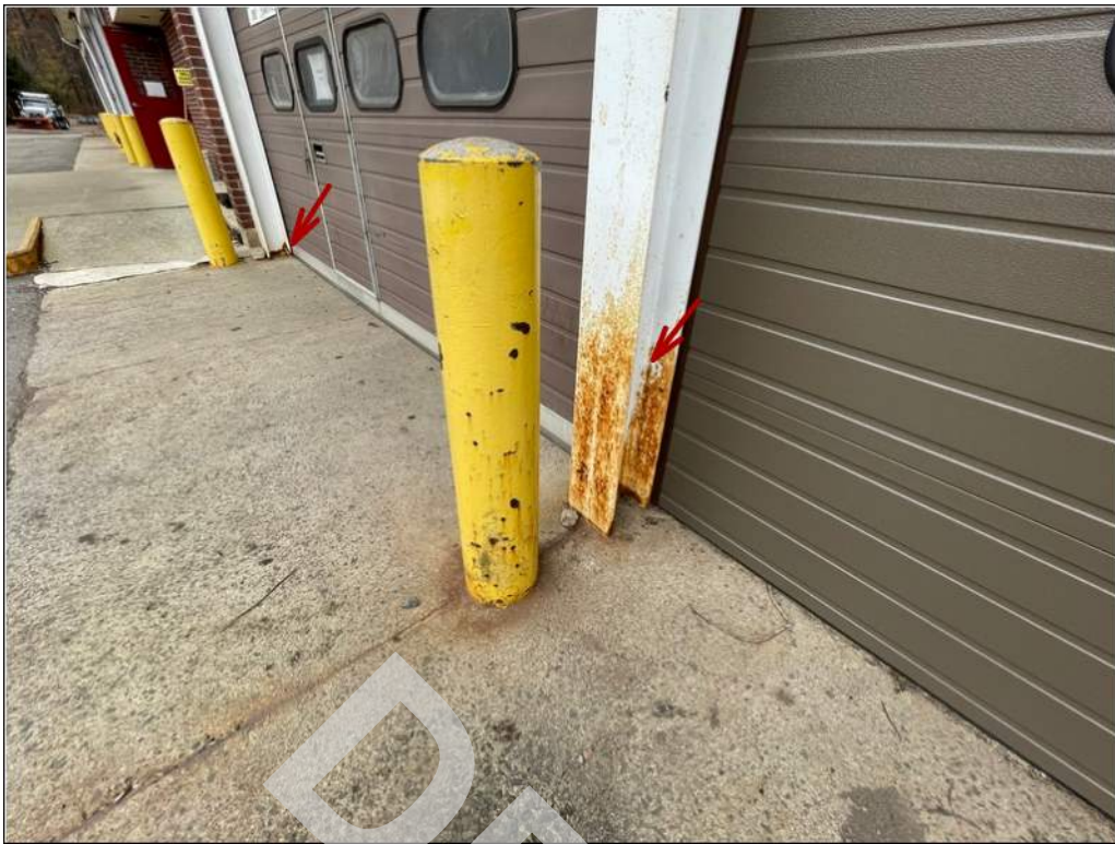
5 - Steel column surfaces have corroded.
