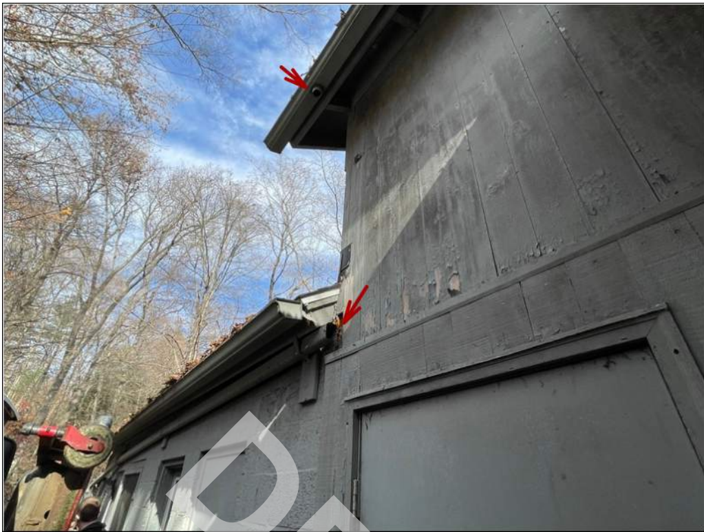
7 - Barn: A roof leader is missing along the west side of the barn.
