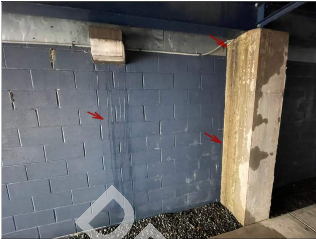
11 - Water from the grandstand is dripping along the team room CMU (Concrete Masonry Walls) and reinforced concrete structure.
