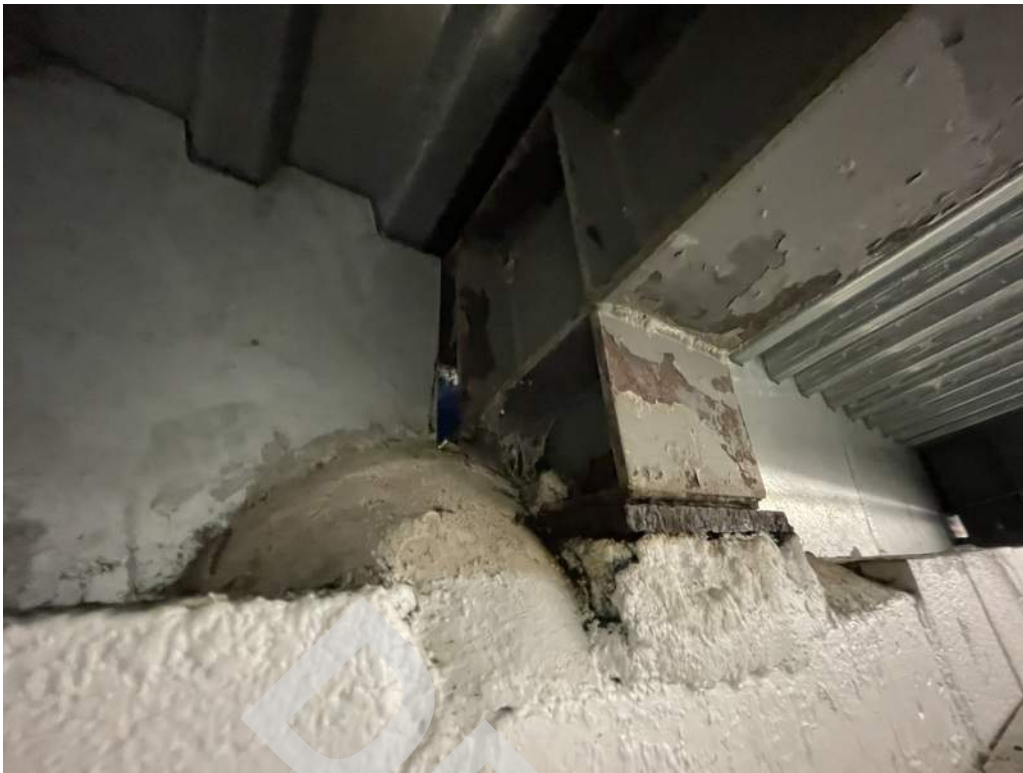
7 - Surface corrosion and peeling coating at the team rooms roof steel framing.
