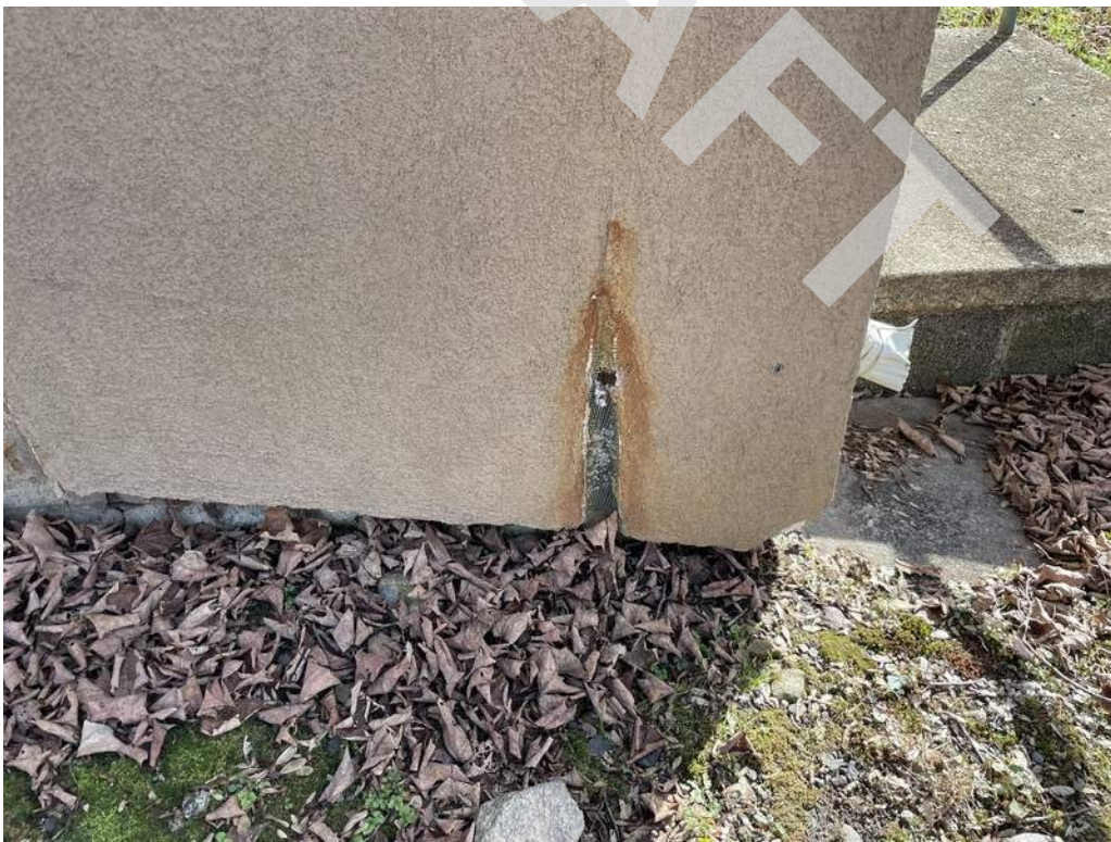
8 - Localized areas of the EIFS have eroded.
