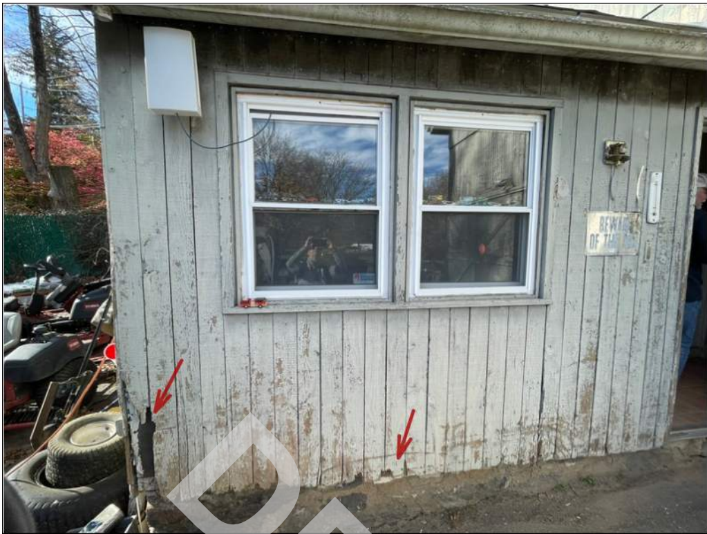
9 - Barn: Wood plank facade is in poor condition, including broken wood planks.
