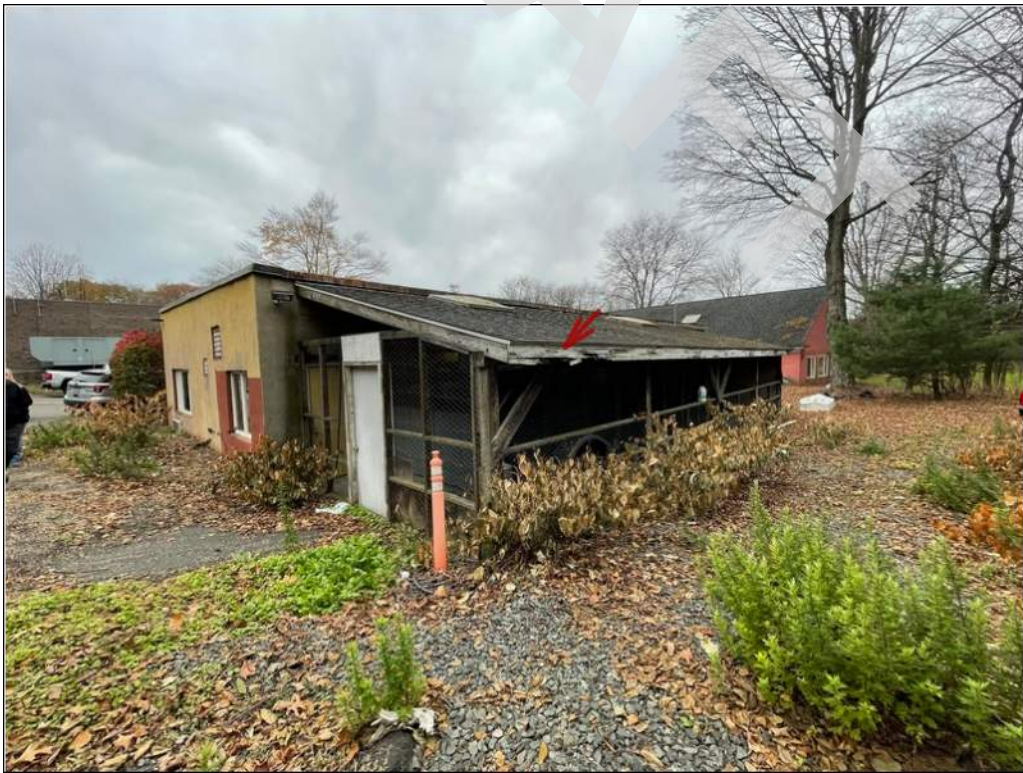
18 - Wood trim around the animal shelter kennel roof has rotted.
