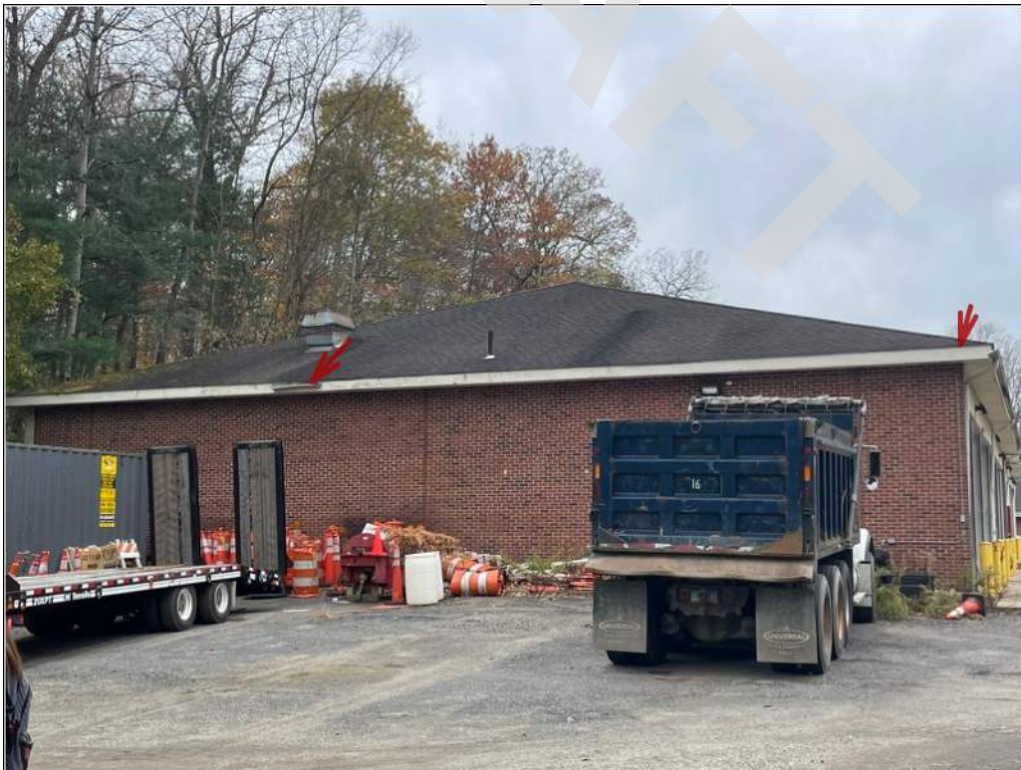
10 - Roof gutter is missing and fascia has damages along the east facade. Roof deficiencies include organic growth and stained asphalt shingles.
