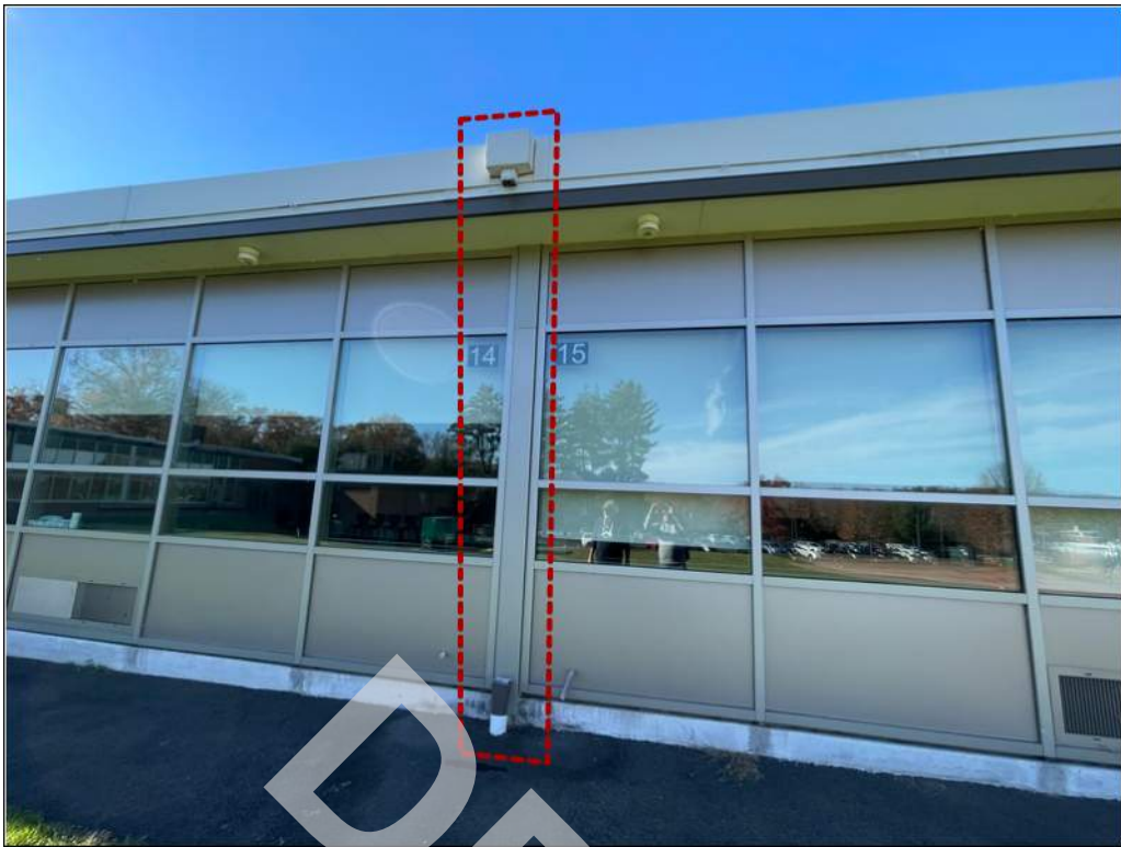
11 - The roof leader is missing.
