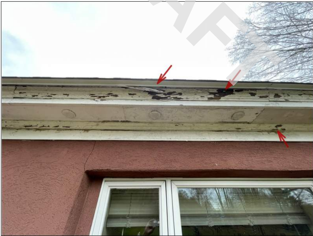
16 - Wooden trim and soffits along the roof perimeter are in poor condition. Wood has rotted and paint finish is peeling.
