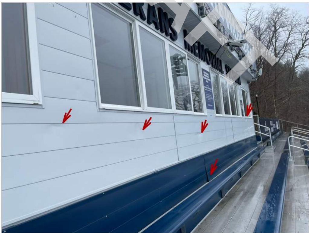
8 - Various metal panels along the Press Box enclosure have dents or have displaced.
