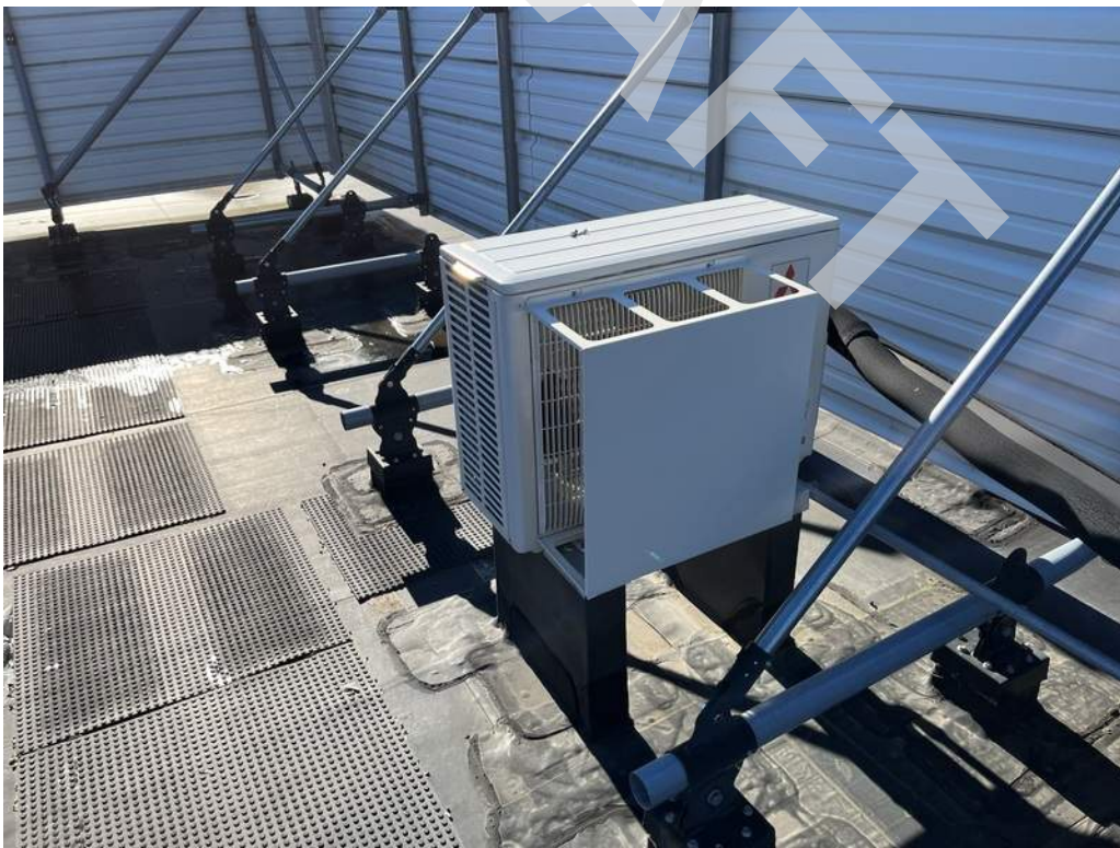
24 - Split system air conditioning units are located on the roof and provide cooling to portions of the building.
