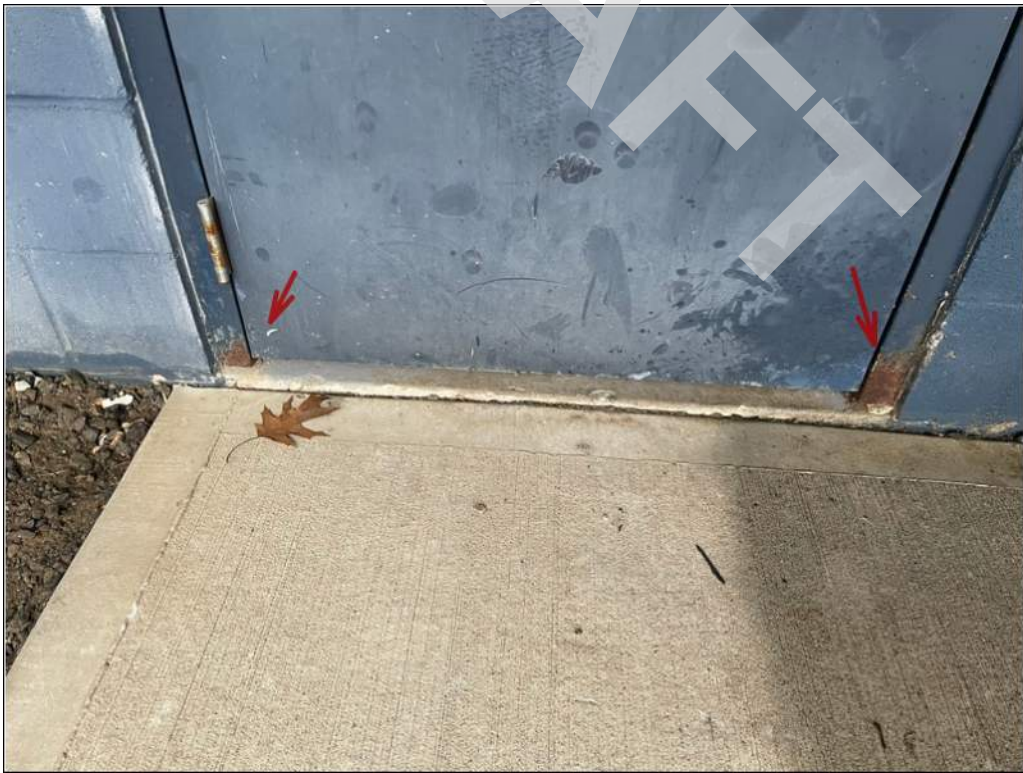
16 - Metal surfaces along the frame and doors at the team rooms are starting to corrode.
