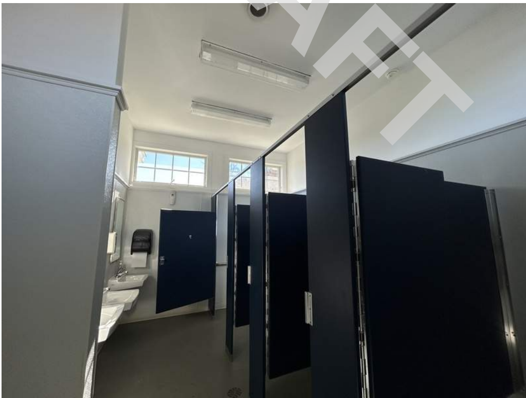
8 - Interior restroom finishes consist of painted gypsum board ceiling and boards and painted concrete slabs.
