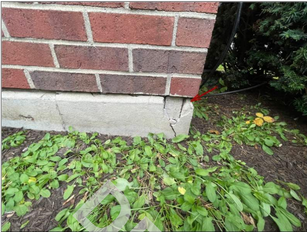
3 - Areas along of the cast-in-place reinforced concrete foundations walls have spalled and appear to have been previously repaired.
