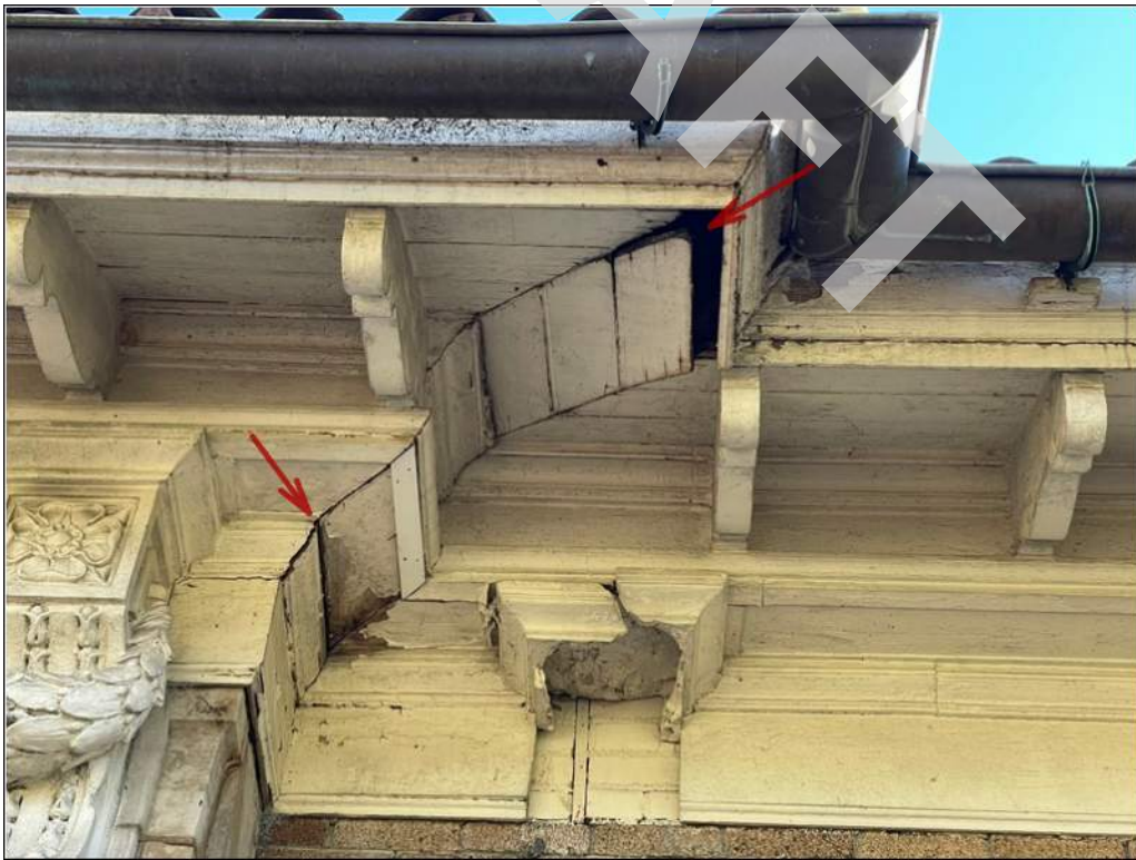
22 - Wood soffits and trim around the roof have displaced and open joints; paint finishes are peeling; wood surfaces are rotting and have missing pieces.
