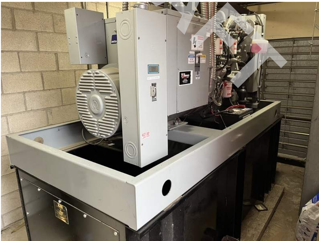
24 - A diesel-fired emergency generator located in a generator room in the Fire Headquarters provides emergency power to the Fire Headquarters and Garage buildings.
