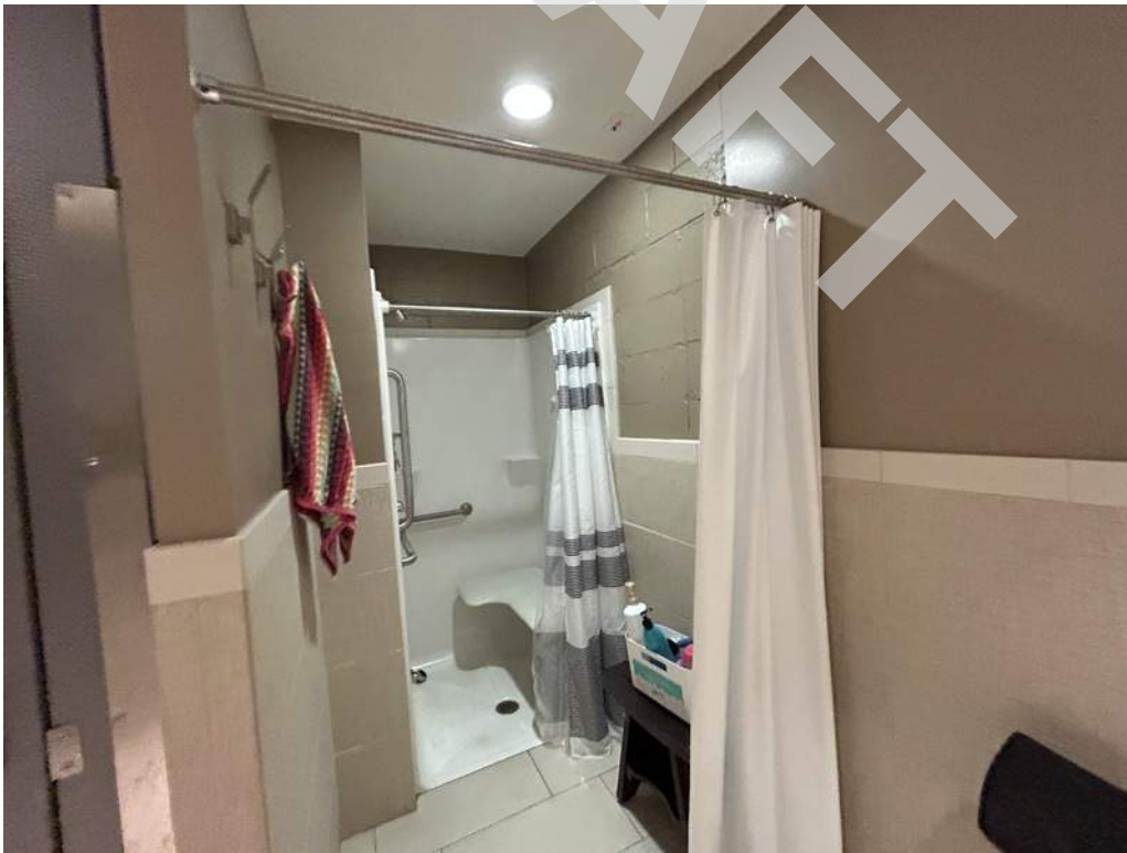
38 - The minimum required clearance measured from the transfer shower control wall is not provided.
