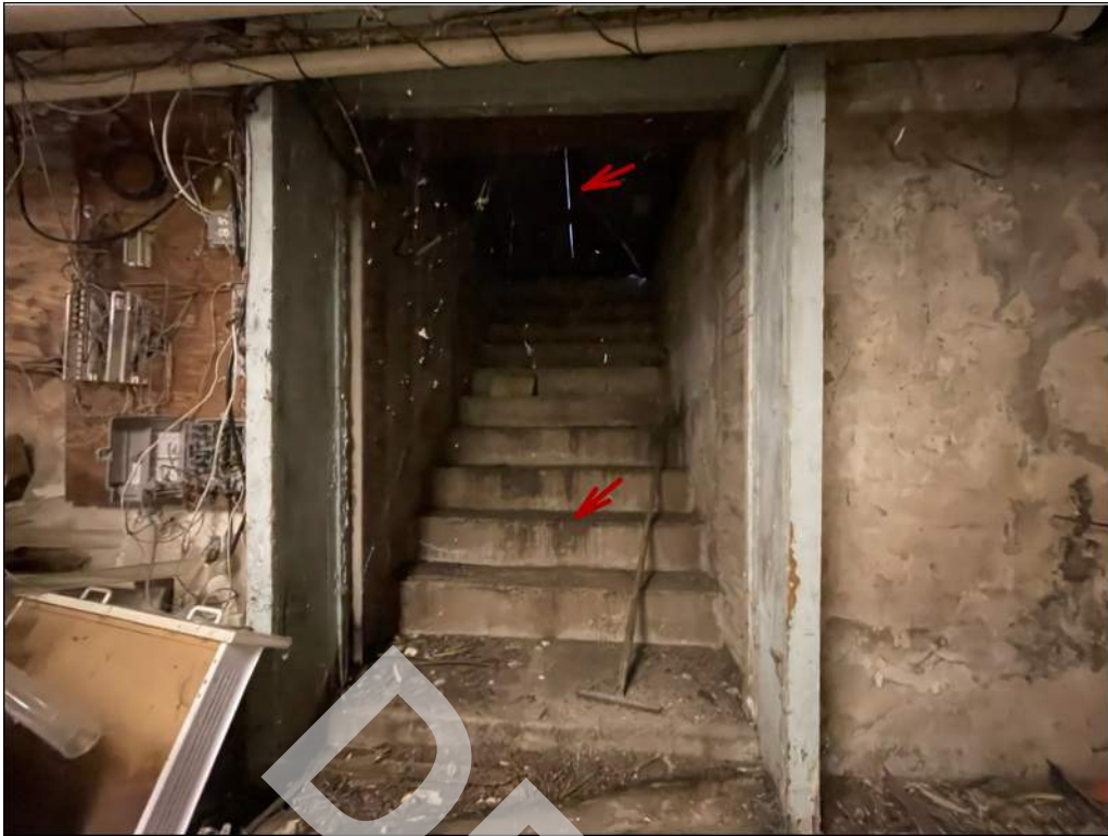
21 - Basement hatch door doesn't close properly and steps have signs of water intrusion.
