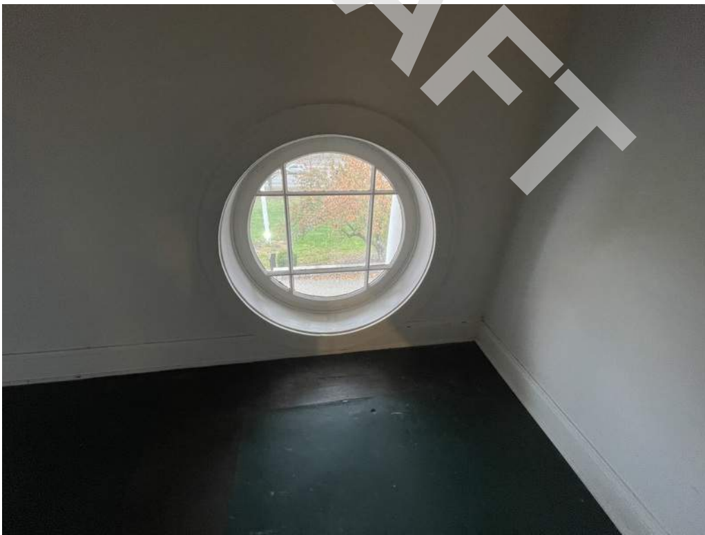
24 - Round windows along the front facade do not appear to include safety glazing.
