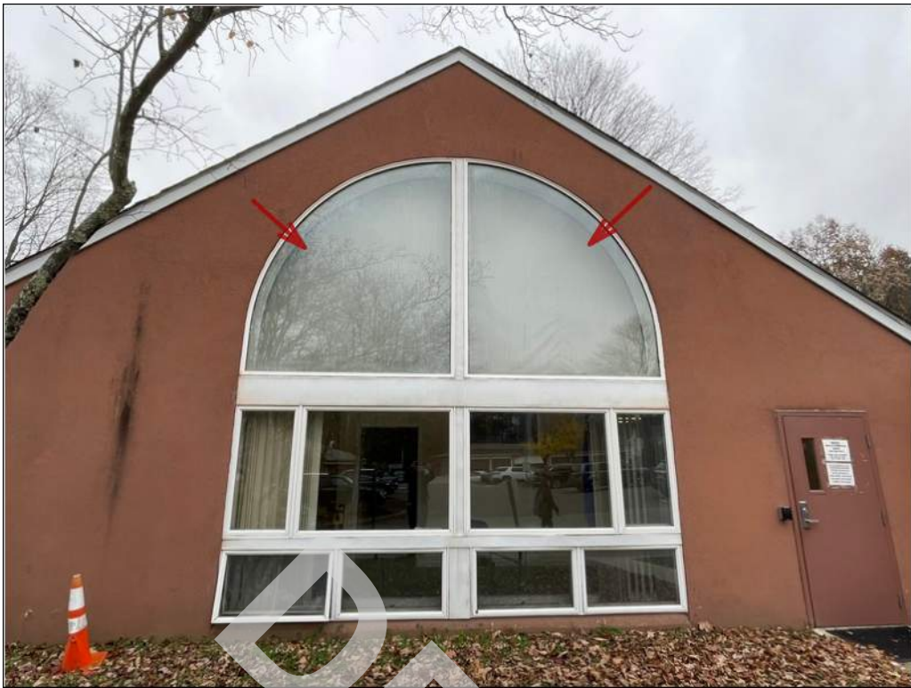
11 - Quarter circle window units along the south facade have failed.
