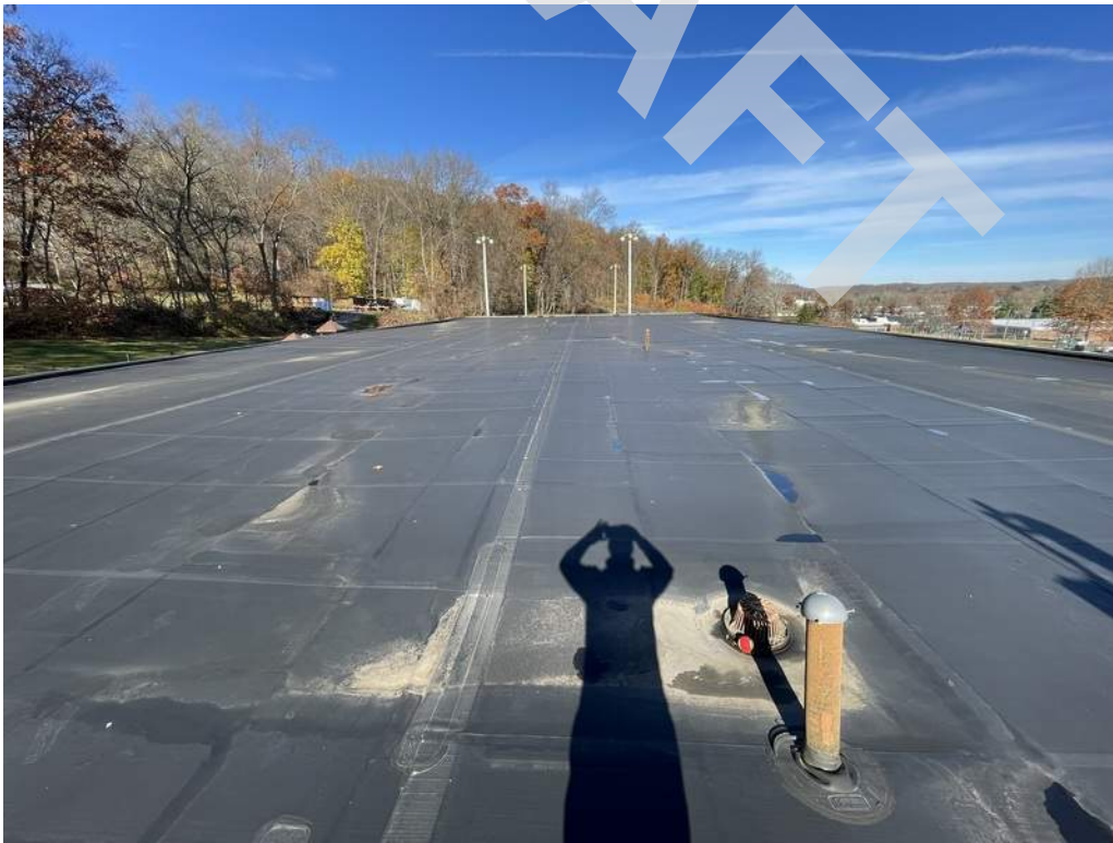
8 - The roofing system consists of an EPDM (ethylene propylene diene terpolymer) membrane.
