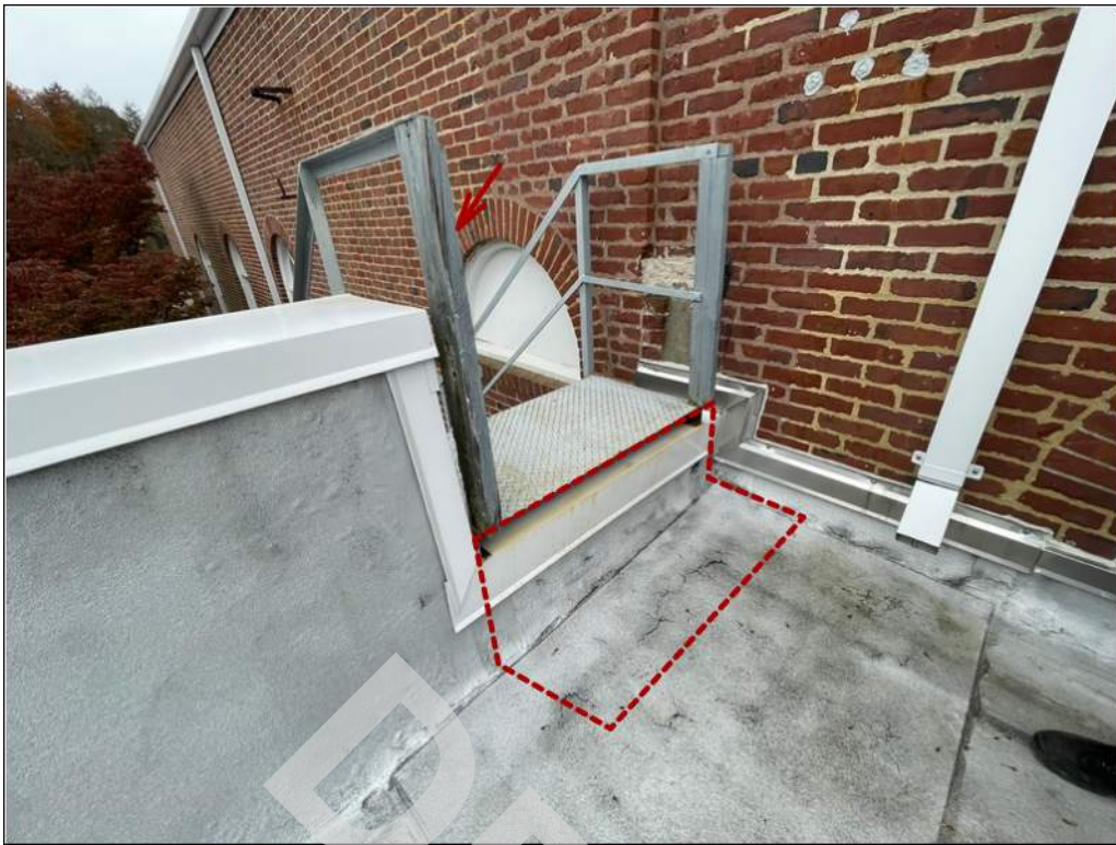
37 - Height of the riser in the path of egress is above the code requirement. Previously repaired handrail support.
