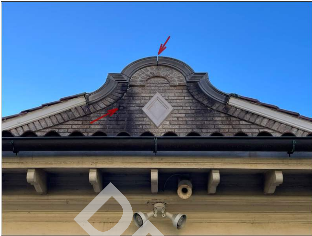
15 - Localized areas of mortar joints are missing or are in poor condition along the masonry brick and stone facades. Areas of the stone and brick masonry have organic growth and debris accumulation.
