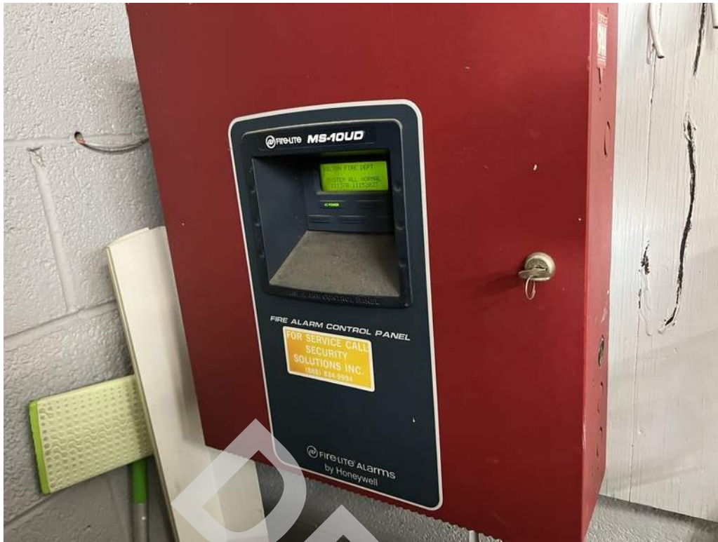
21 - The building is provided with a Fire-Lite MS-10UD fire alarm panel.
