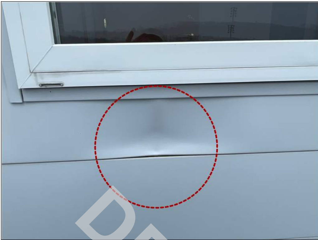
9 - Metal panel dent has opened the joint between panels.
