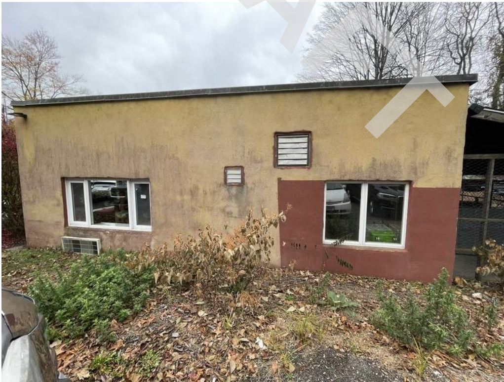
10 - Exterior wall finishes at the animal shelter stucco facade are in poor condition.
