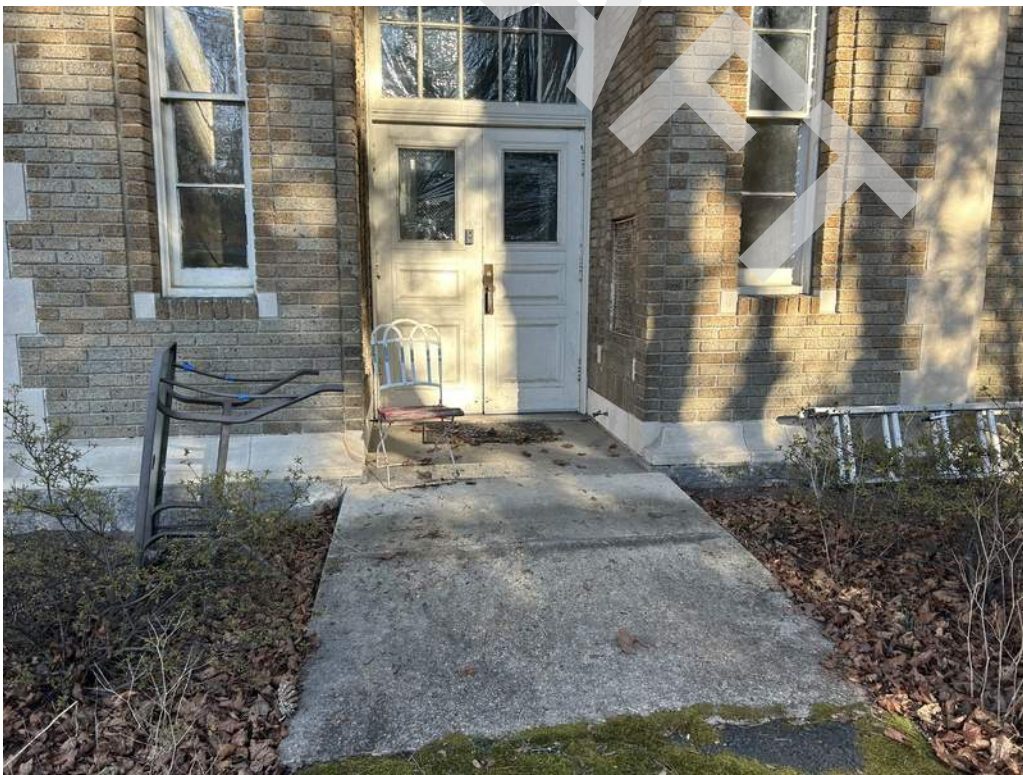
30 - The minimum clear width is not provided at the accessible entrance door.
