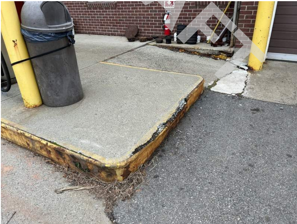
4 - Walkways exhibit concrete spalling and deterioration.
