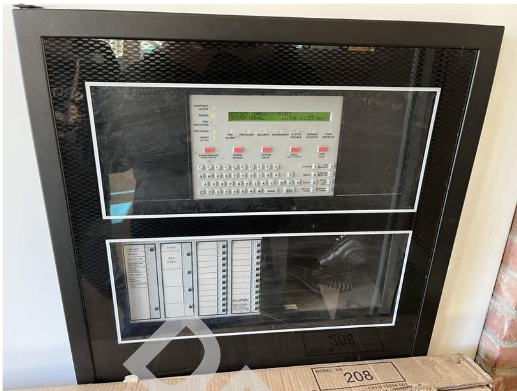
29 - The building is provided with a fire alarm panel which is located in the vestibule of the main entrance.
