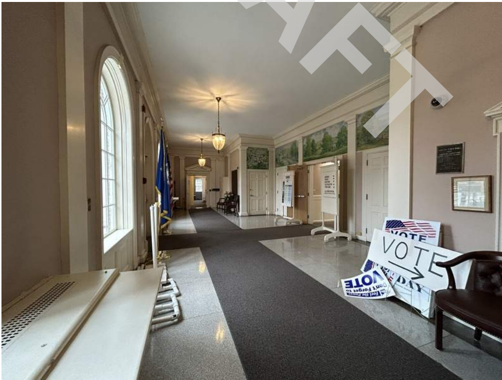
38 - Interior finishes at the lobby consist of painted gypsum ceiling and wall boards and terrazzo floors.
