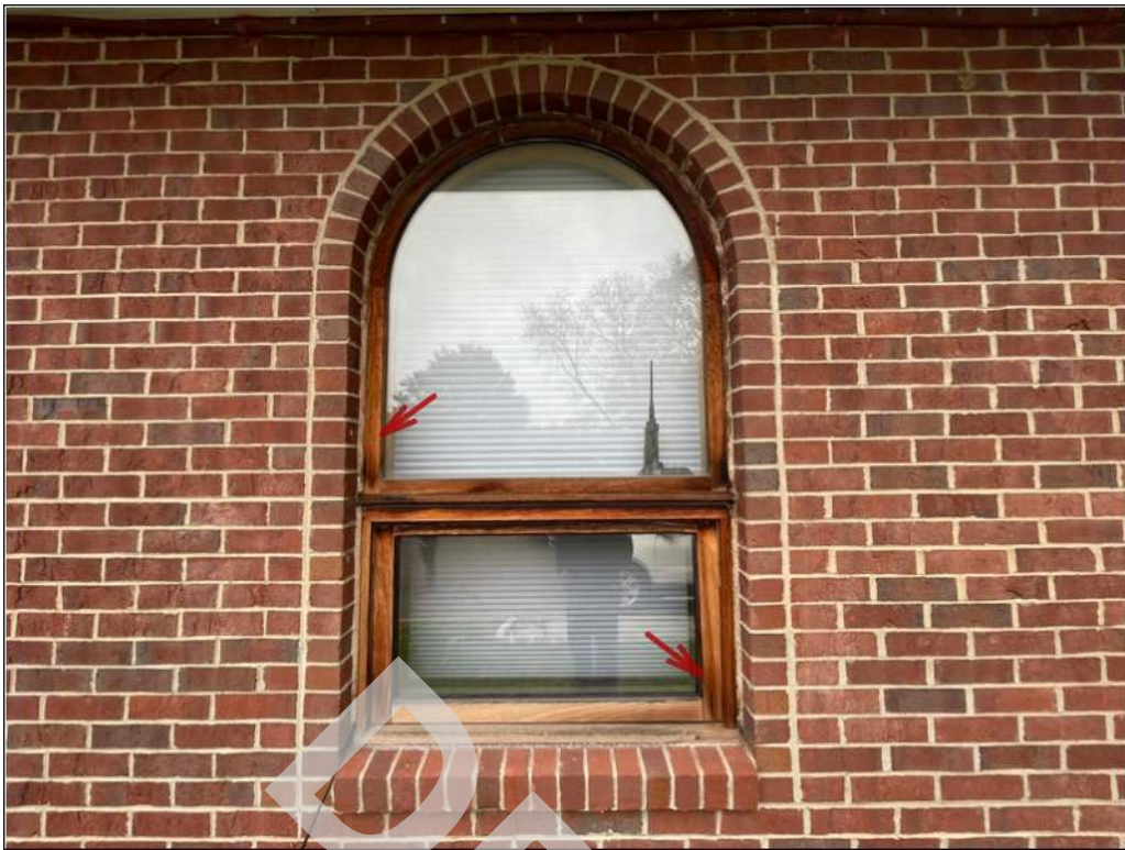
11 - Wood framing surfaces at the operable and fixed windows throughout the building have worn out and are in fair condition.
