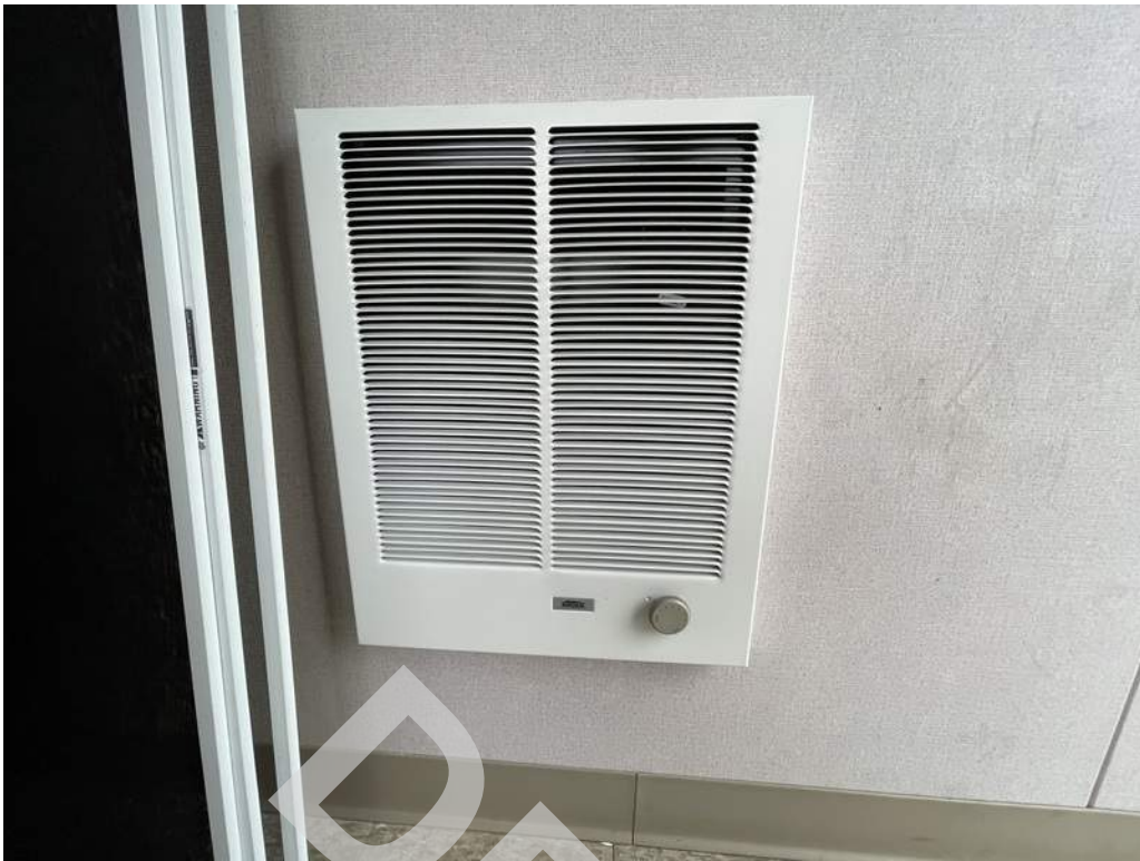
21 - Recessed wall heaters provide heating to the press box.
