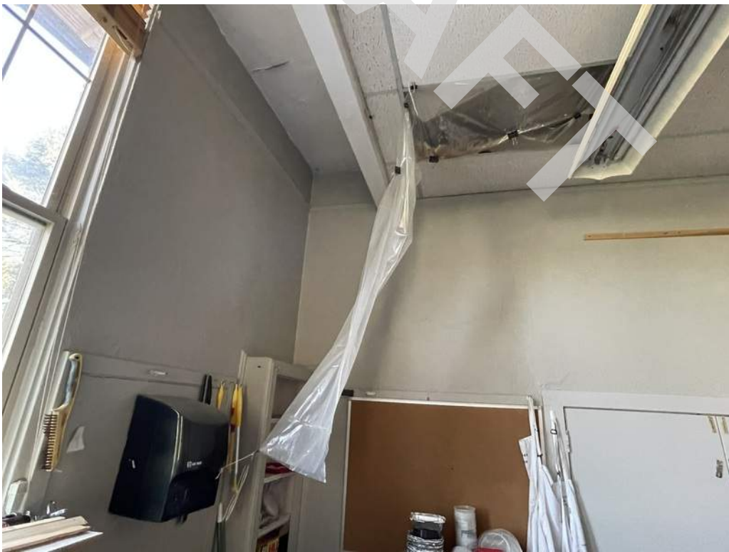
12 - Signs of active roof leaks coming down from the ceiling at one of the art studios.
