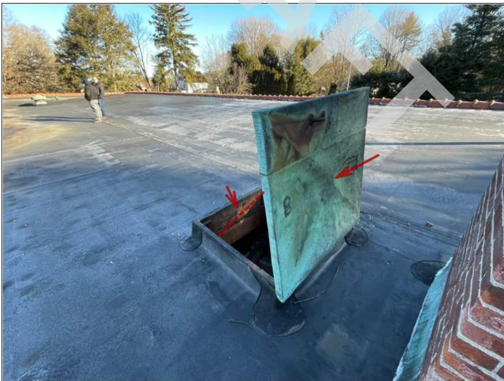
8 - Roof hatch is missing one hold open hardware and is in poor condition.
