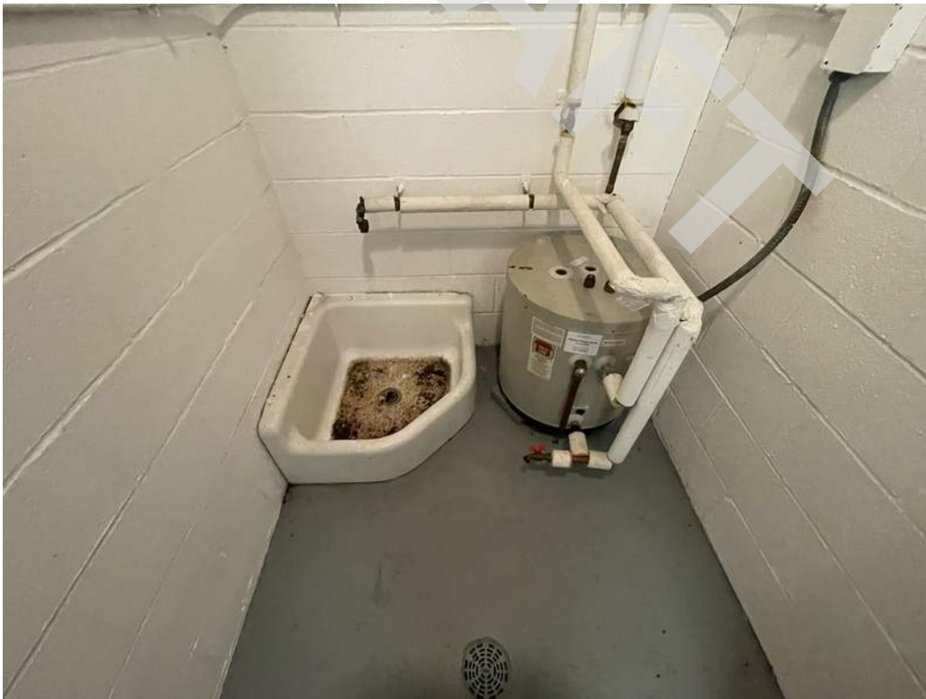
22 - An electric storage type water heater located in the janitor's closet of each team room provides hot water to the building.
