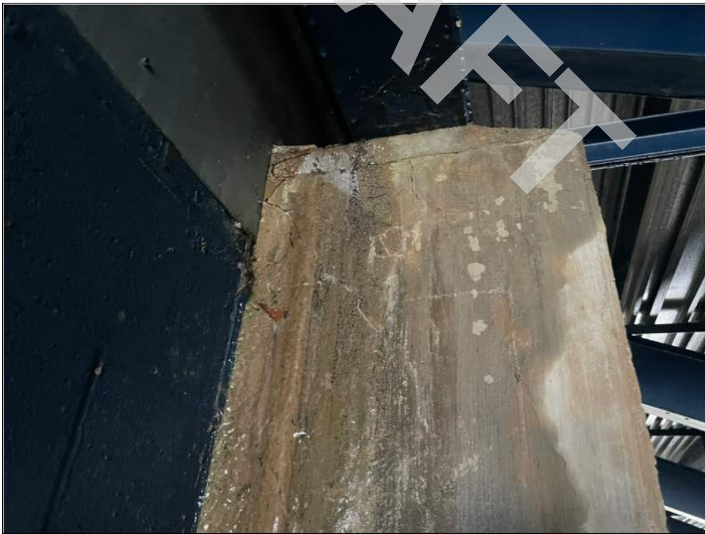
12 - Water dripping from the grandstand is freezing along the concrete column surfaces.
