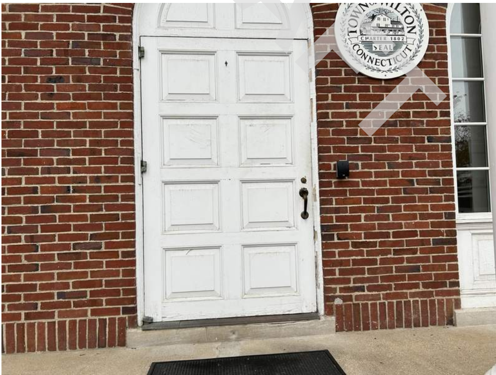
30 - Main entry wood door is in poor condition. Deficiencies include deteriorated door hardware and peeling finish surface.
