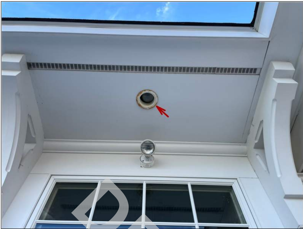
5 - Recessed lighting metal rings have corroded due to water and moisture exposure.
