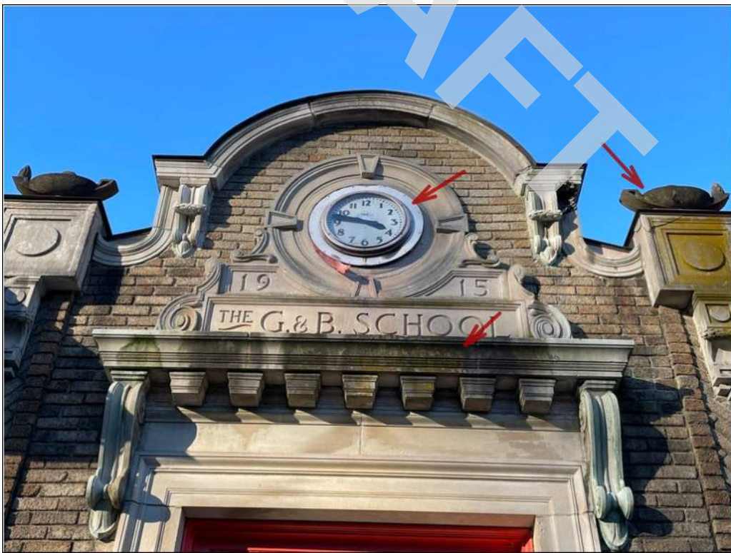
14 - Building clock is not working properly and appear to be in poor condition. Organic growth and build up stains are in the front facade stone.
