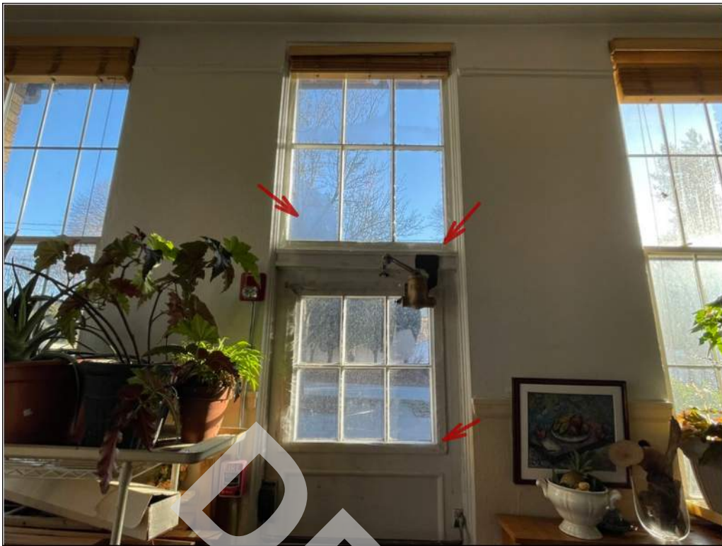
17 - Single pane glass window unit above the door and on the door leaf have condensation and have been covered with window films to reduce draft.
