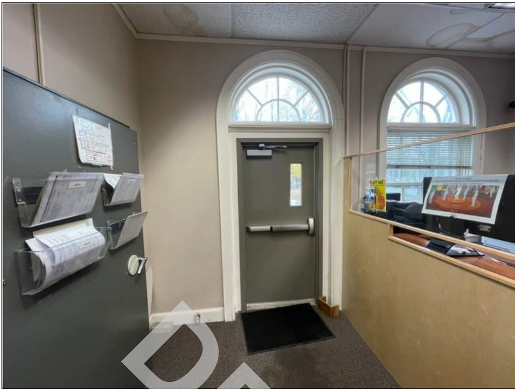
57 - Exit signage and pull alarm are not provided at the egress door.
