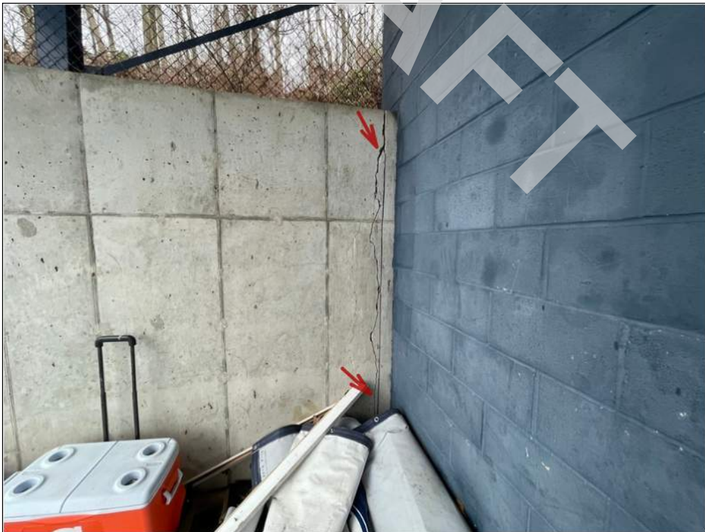
4 - A crack was noted along the entire height of the retaining wall next to the south team room enclosure.
