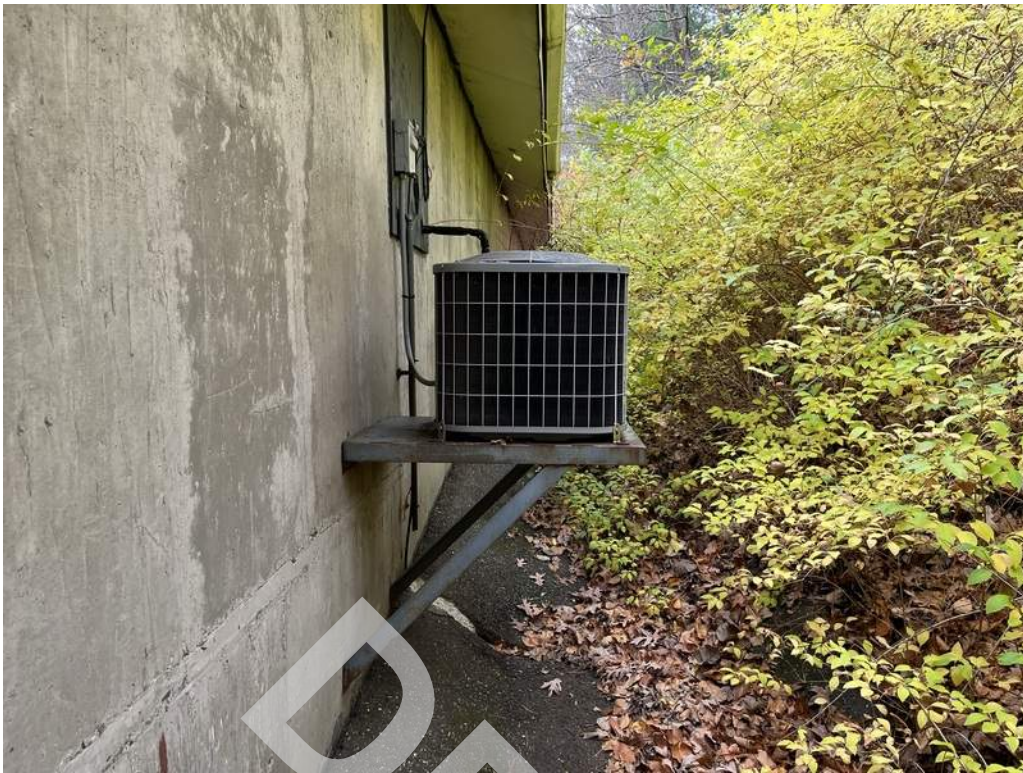
21 - A split system air conditioning unit located on the exterior of the building provides cooling to a portion of the building.
