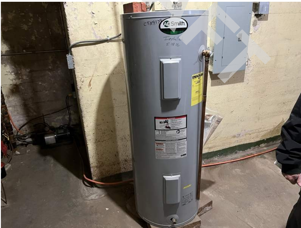
52 - An electric storage-type water heater is located in the basement and provides hot water throughout the building.
