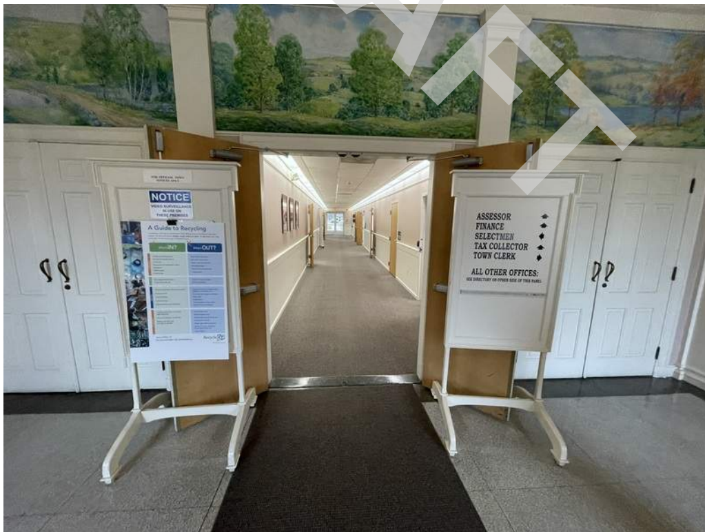
56 - Fire rated doors are held open by signage.
