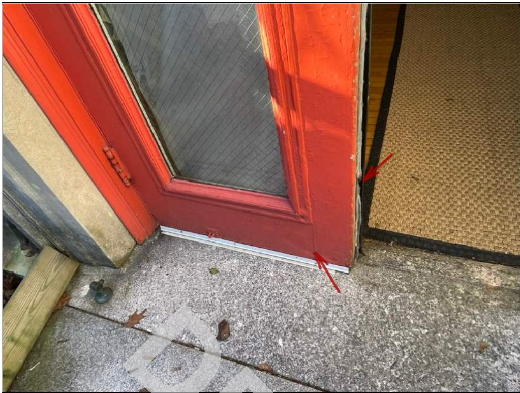
19 - Wood surface and weatherstripping are in poor condition.
