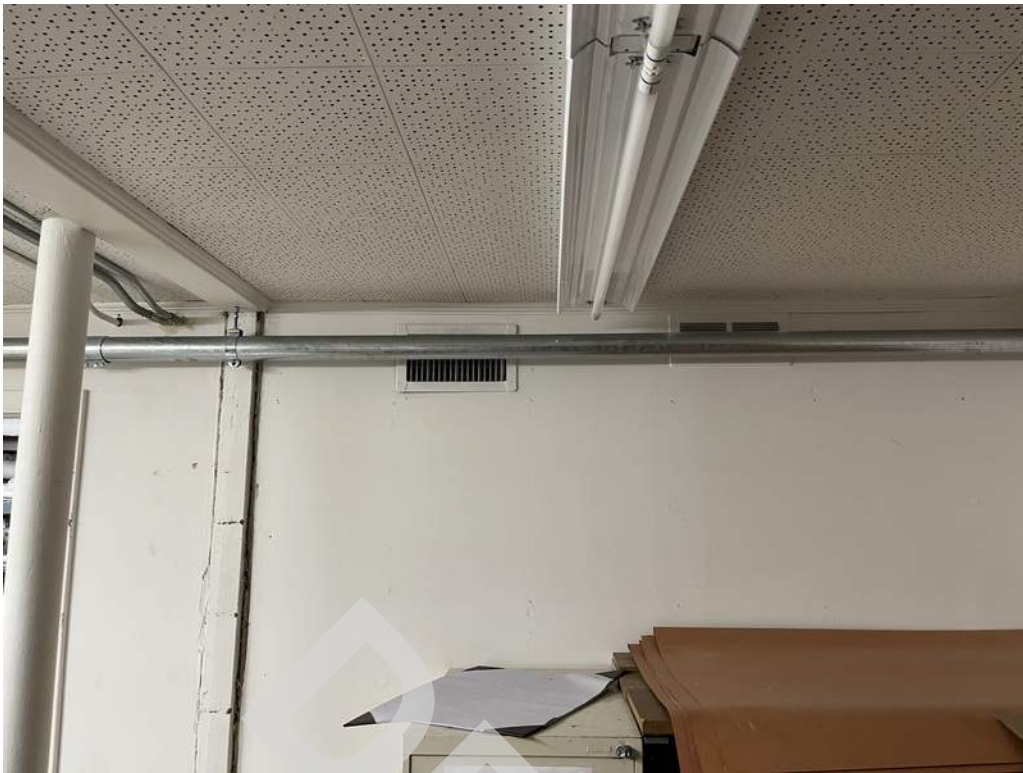
51 - A conduit in the basement is currently partially blocking two wall mounted grilles.
