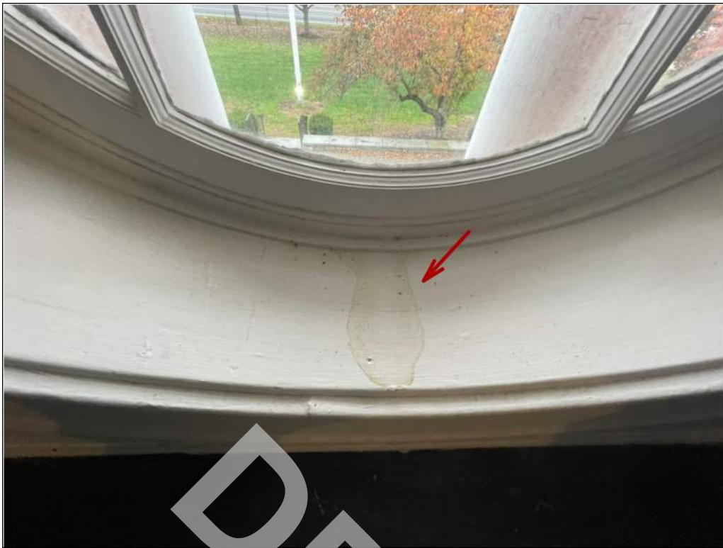
25 - Signs of water intrusion through the round windows along the main facade. Windows are single pane glass units with no safety glazing.
