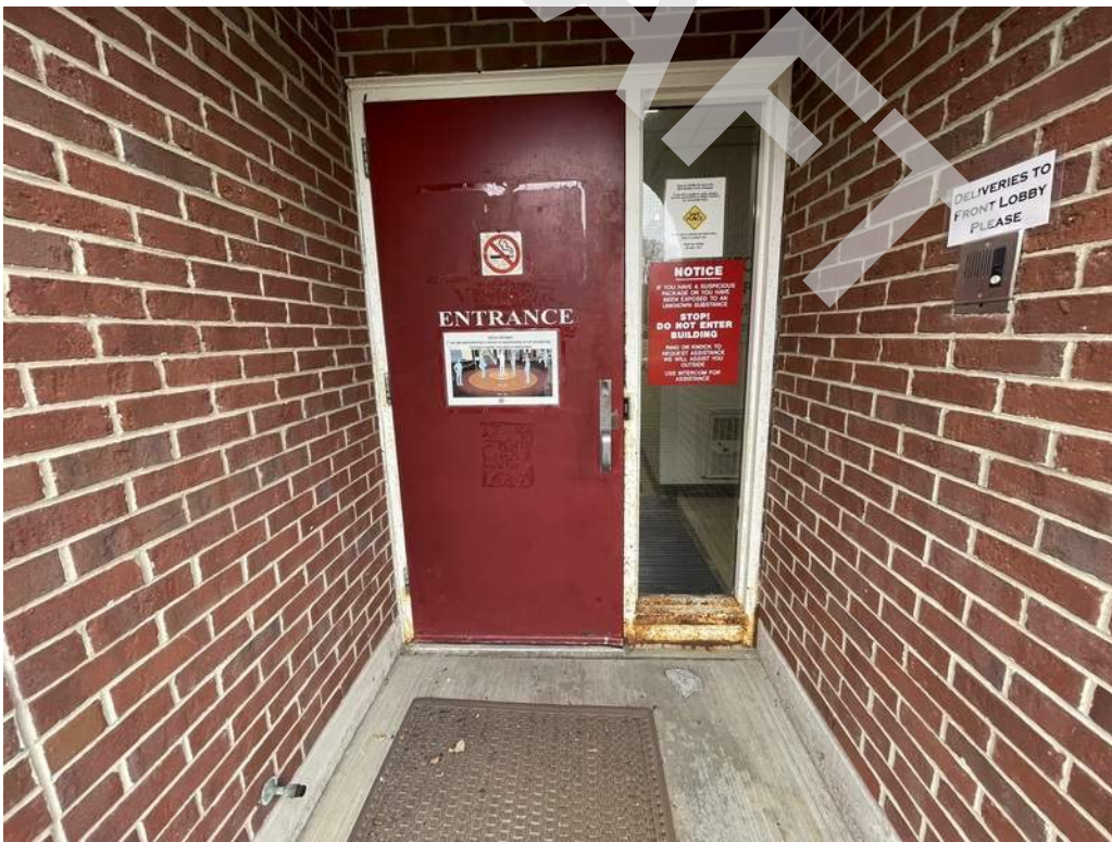
14 - Side light framing has corroded along the bottom. Hollow metal door surfaces are in fair condition.
