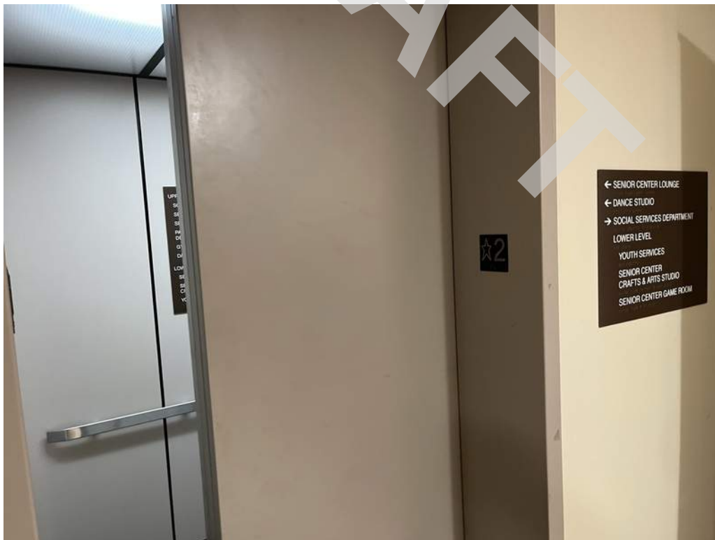
30 - The building is provided with a Kone hydraulic passenger elevator located in the east wing of the building.
