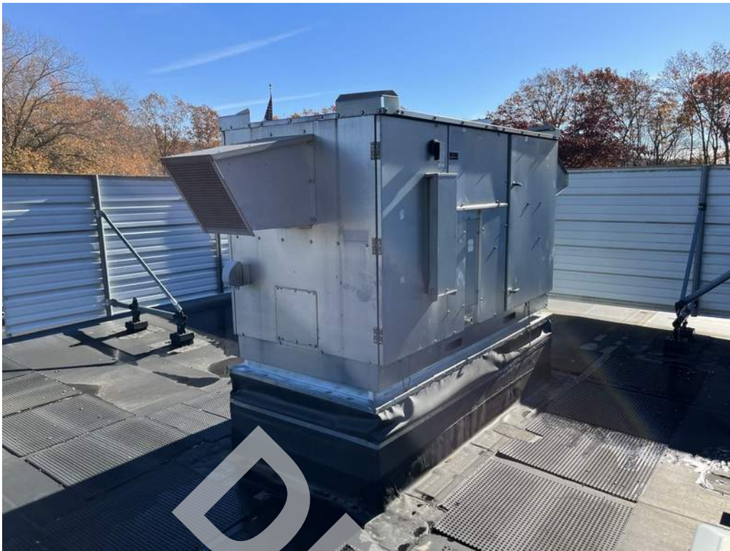
23 - An energy recovery ventilator provides conditioned ventilation air to portions of the building.
