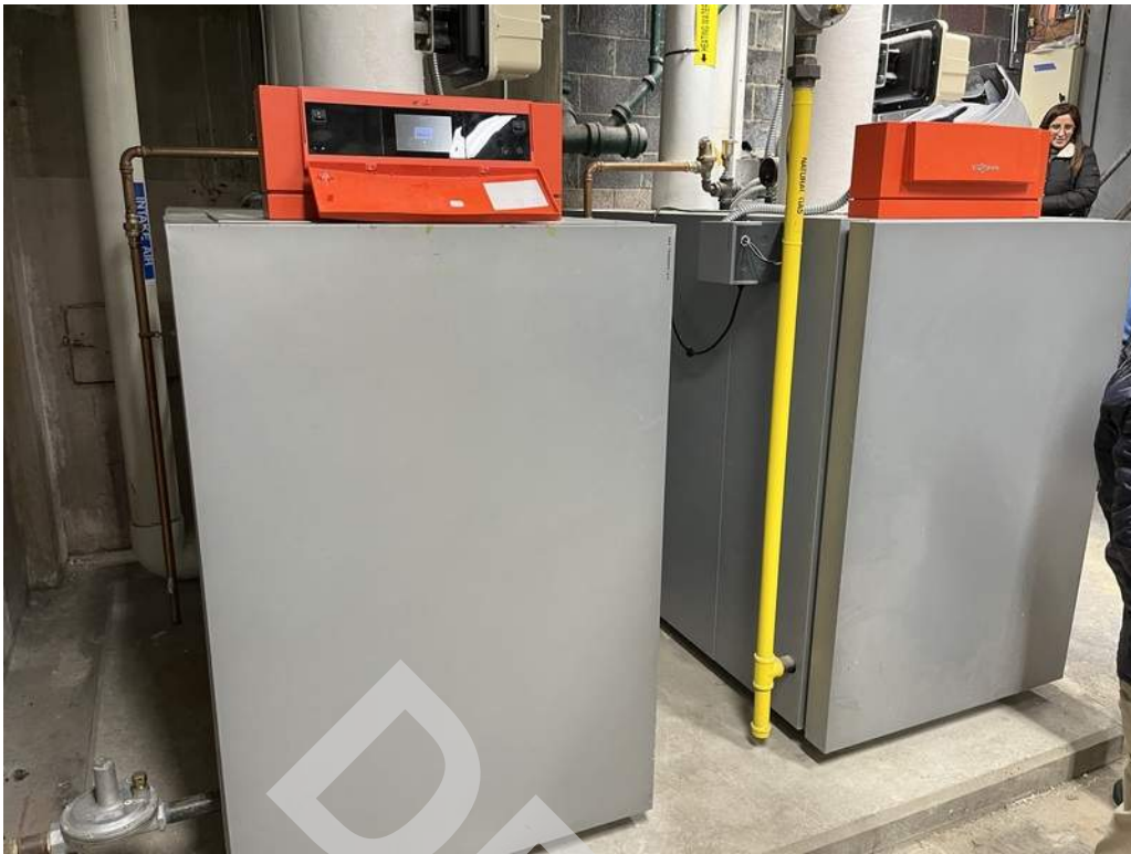
21 - Two natural gas fired boilers located in the lower level provide heating hot water throughout the building.
