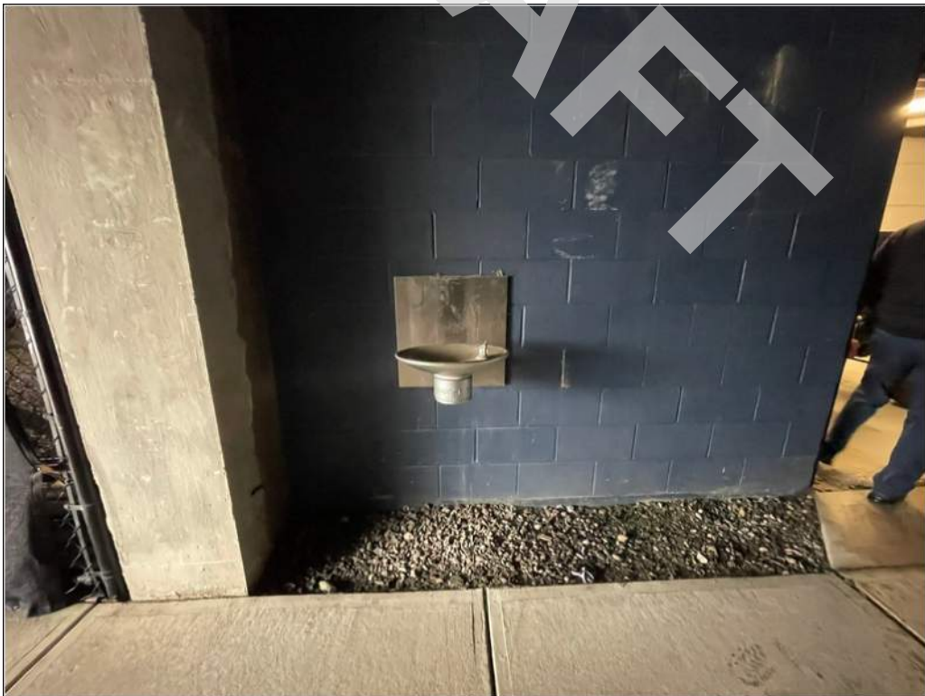
24 - Water fountains are not provided with a firm surface for front approach.
