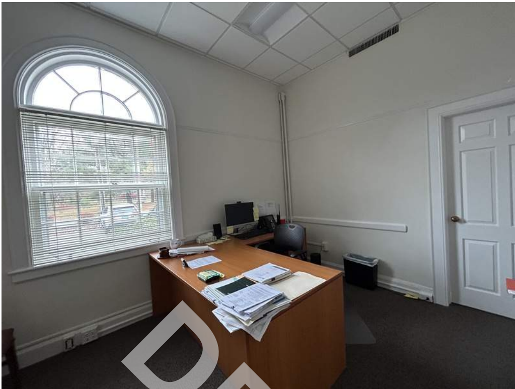
41 - Interior office finishes consist of painted gypsum wall board, suspended grid ceilings with acoustic tiles, and carpet floors.
