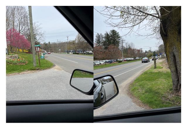
The picture on the left shows the new sightline to the north if the stop bar is moved forward (10 Ft). The picture on the right shows the new sightline to the south if the stop bar on Own Home is moved forward (10 Ft). The tree on the right side of the picture should be removed.
