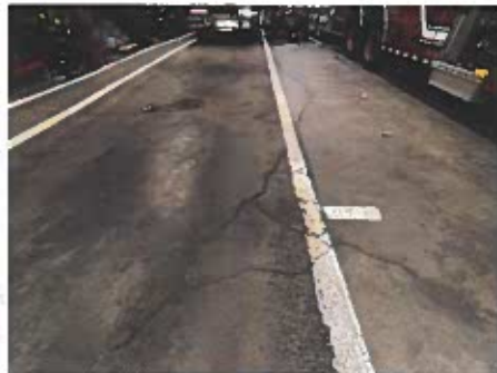
Cracked apparatus room slab
