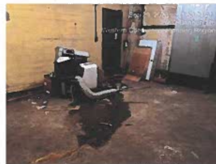
Water intrusion at the basement
