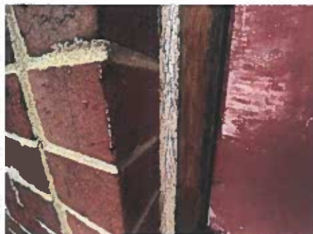
Failed sealant
