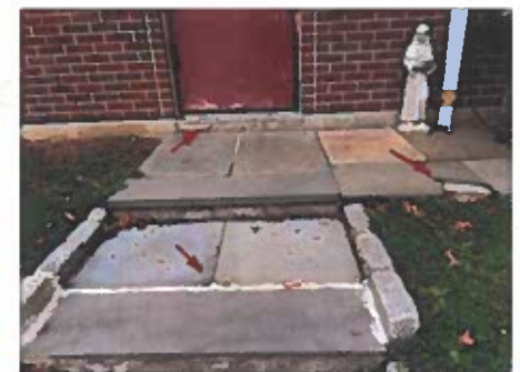
Cracked and spalled landing and steps
