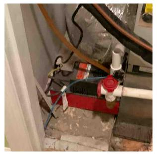
9.5.2 There is corrosion in the attic air handler overflow drain pan indicating a past or current leak. Recommend HVAC evaluation for proper operation prior to air conditioning season to prevent overflow, secondary damage or loss of function.
