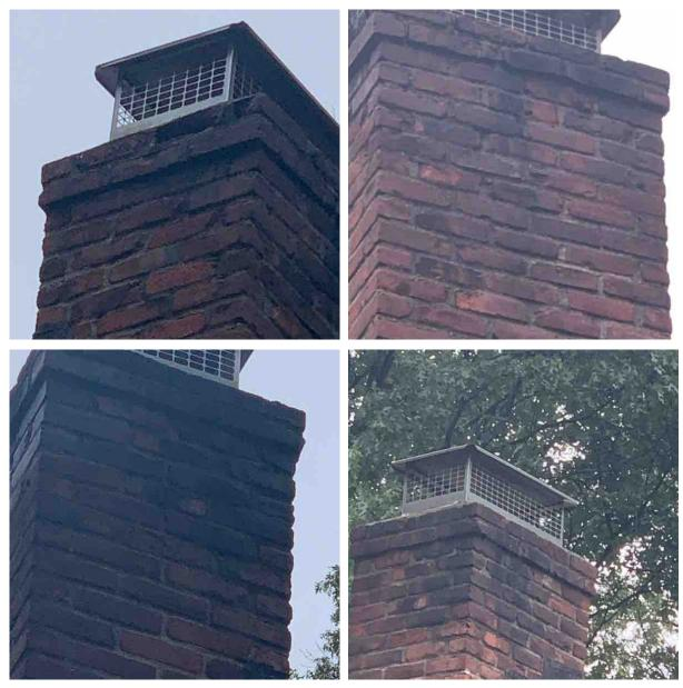
4.6.3 Vintage chimneys are subject to concealed defects from decades of daily wear and exposure to acids produced by combustion gases. While a section of the flue liner may or may not be visible at the roof top, the middle sections of the flue are concealed and often deteriorated.
