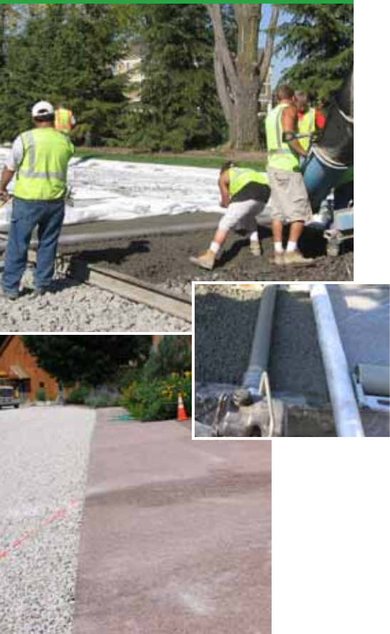
Pervious concrete is a top performer with respect to water quality treatment and volume reduction, however care must be taken in areas where deicing chemicals will be used.
