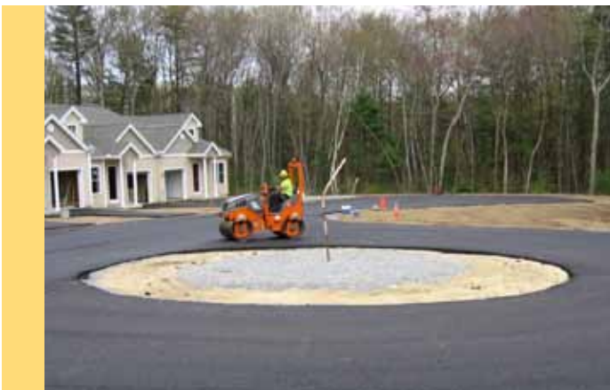
Final rolling of a new porous asphalt roadway installation in a residential subdivision in NH.
