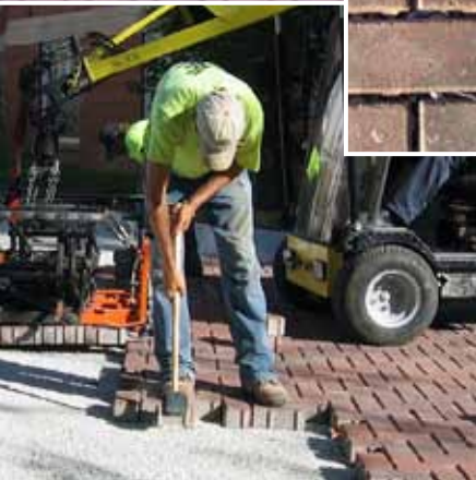
PICP is a high durability and logical choice for effective stormwater management. PICP provides remarkable runoff volume reductions while providing an enhanced aesthetic appeal.
