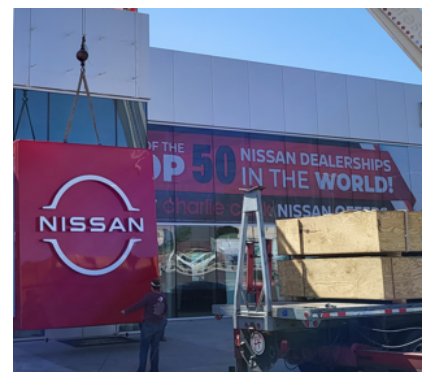
Step 5: Clear pathway and arrange crew for installation to the facade. Use tag lines to assist with guidance.
