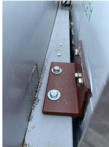
Step 7: Secure all 4 tablet mounting angles with 2 bolts each. Ensure that the tablet is level with the parapet and centered over the doors.
