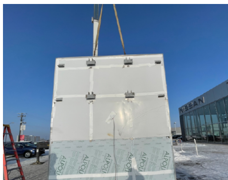
Step 4: Lift upright. Using crane, unbolt shipping stand from tablet frame (remove hardware and set aside). Add tag lines to left and right side of tablet.
