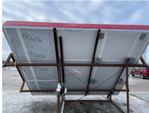
Step 2: While still supported by the crane, detach the angled ship stand assembly and save hardware.
