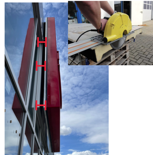
Step 8: Measure at least 4-5 points on each side of the tablet to ensure the cut will be clean and accurate to cover the gap. Cut each side of tablet's ACM trim.
