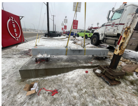
Step 5: Level washer/nuts on anchor bolts. Install torque tube.
