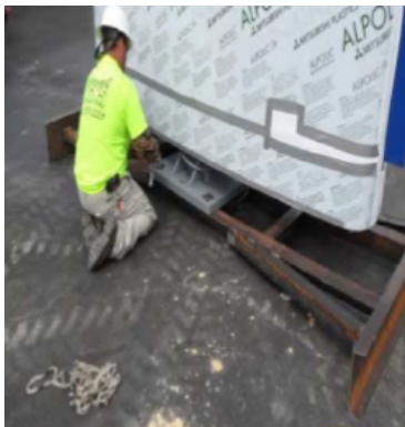
Step 4: Remove bottom shipping stand while sign is still rigged to crane.
