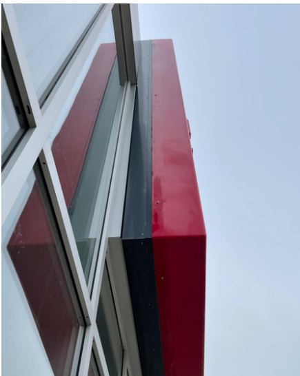
Step 9: Install ACM trim cap using painted tek screws.
