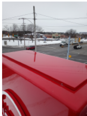
Step 8: Remove top shipping stand and lifting eyes. Attached fiberglass top cap with screws.
