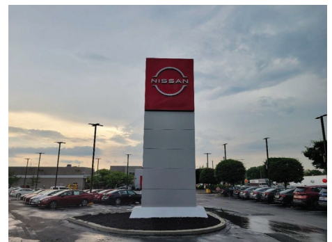
Step 9 : Remove protective wrap , make final electrical connection and install base cover (must be flush with grade and bottom of sign). Ensure access panels open and close properly
