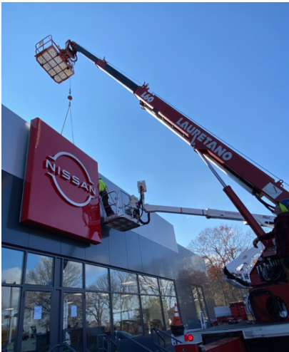
Step 6: Lift and carefully bring tablet to facade and make the electrical connection prior to setting onto the installed template. Crew members use taglines to guide.
