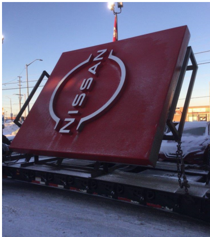
Step 1: Off load tablet from truck and set onto parking lot using 30' lifting straps.
