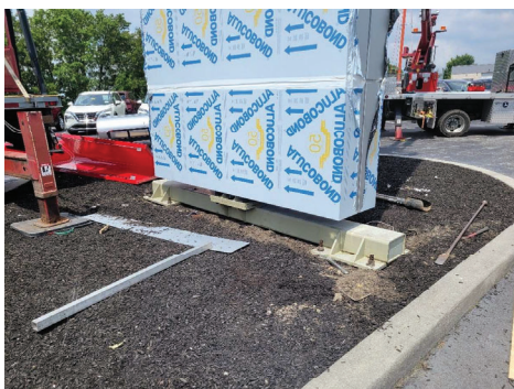
Step 7: Install, level sign and tighten nuts.
