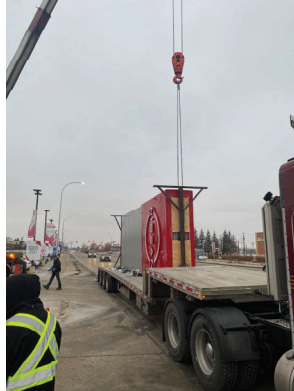
Step 2 : Lift pylon sign off of truck and set onto parking lot. At least 30 ft. long straps must be used.
