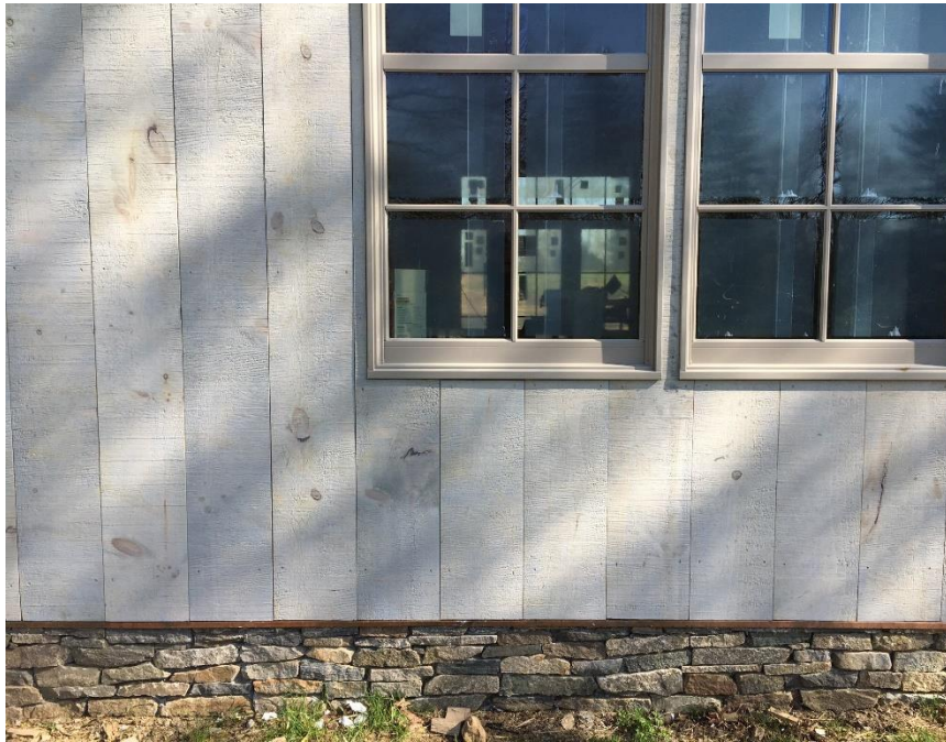
DETAIL: FIELDSTONE FOUNDATION VENEER, STAINED PINE SIDING (FINISHED COLOR), WINDOW SASH AND TRIM (FINISHED COLOR). GALVALUME STANDING SEAM ROOFING- WEATHERED ZINC
