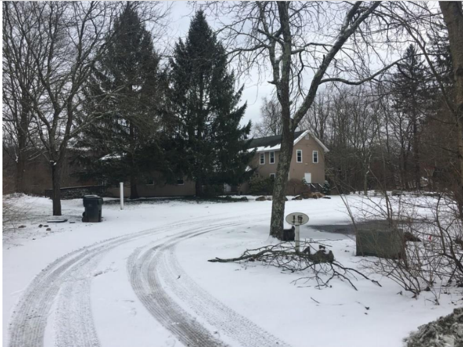
View from common driveway
