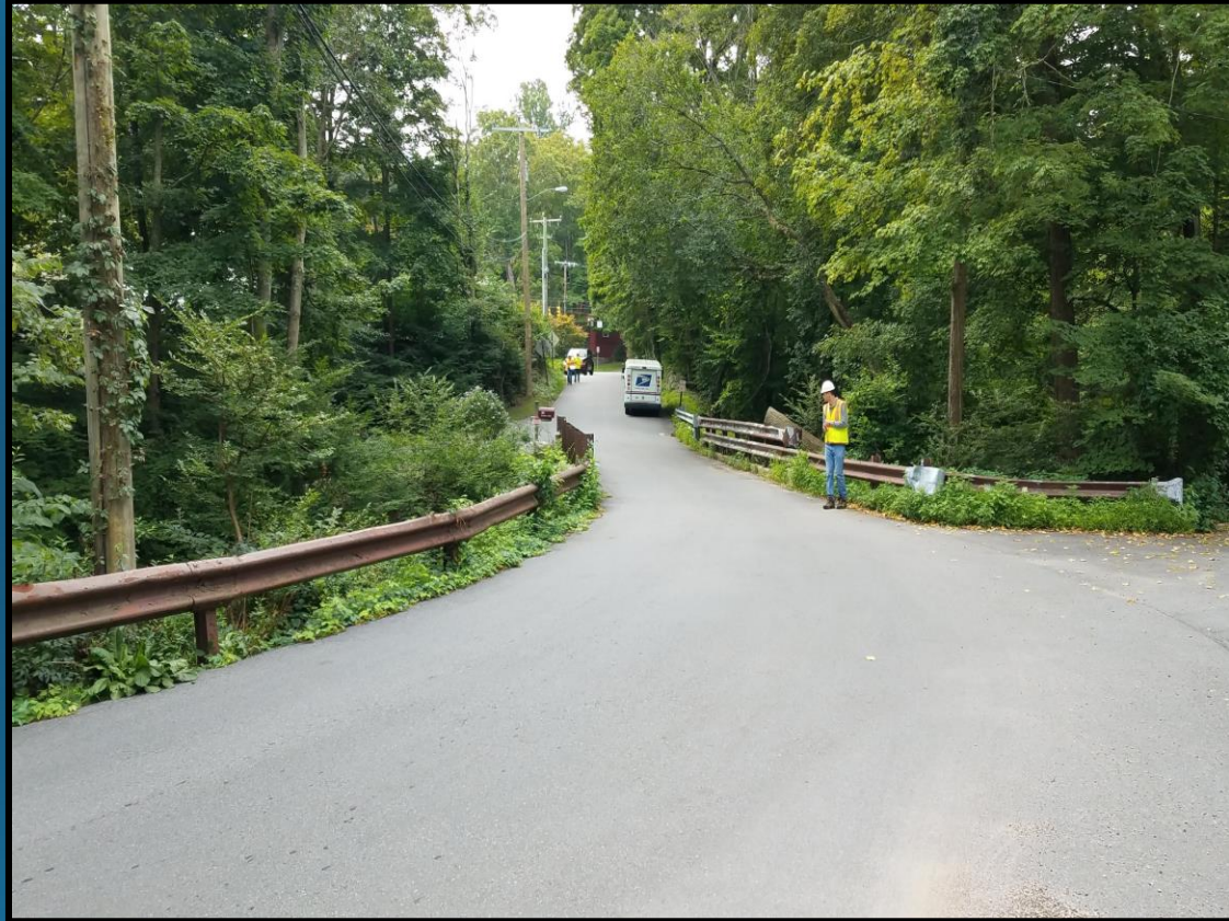
North Approach (Looking South)
