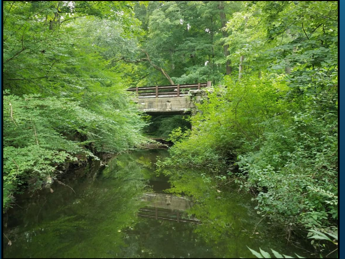
Downstream Face of Bridge
