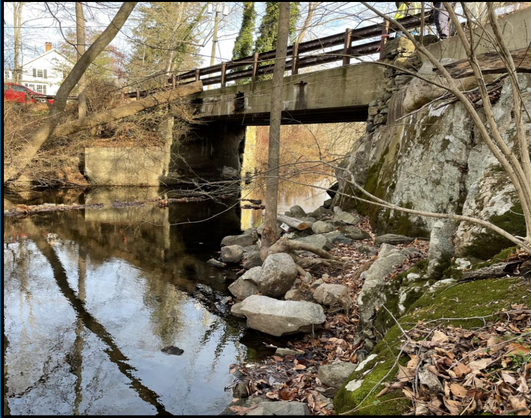
Upstream Face of Bridge
