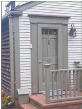
Figure 4. Exterior storm door
