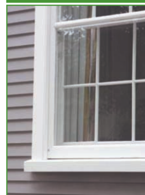
Figure 3. Exterior Storm window
