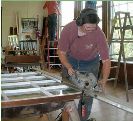
Rebuilding windows in Thetford, VT.
