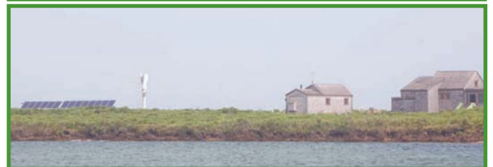
Figure 12. Vertical WECS and photovoltaic array
