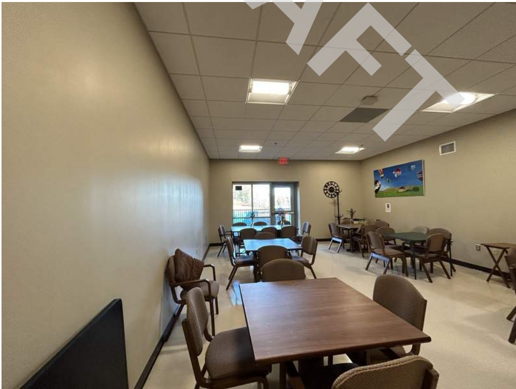
32 - Tables do not provided knee and toe clearance and inadequate clear floor space to the patio was observed at the Senior Center Café.
