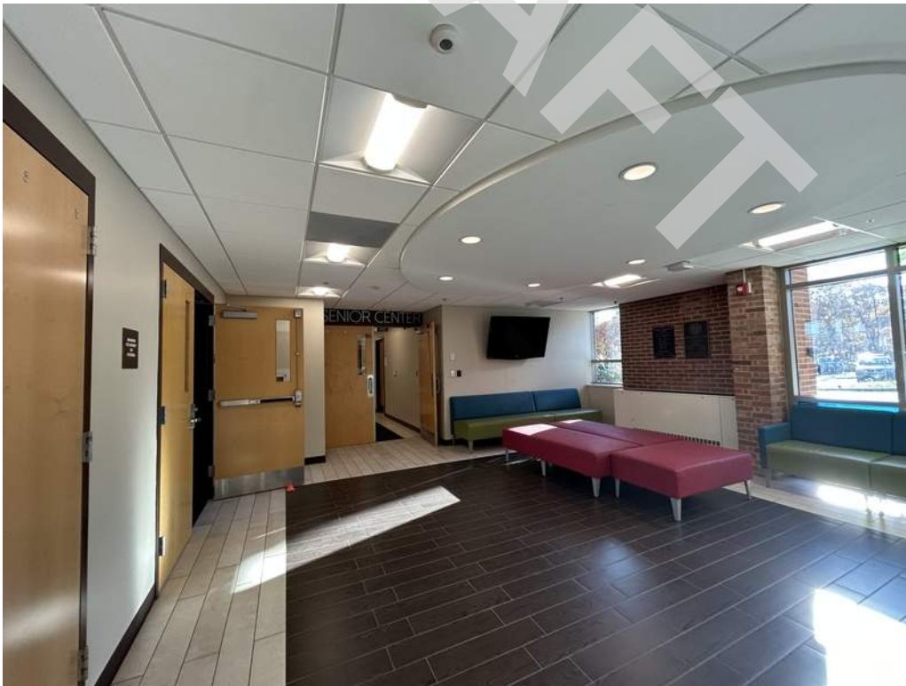
18 - Interior lobby finishes consist of painted gypsum wall boards and instances of brick, suspended ceilings with acoustic tiles, and tile floors.
