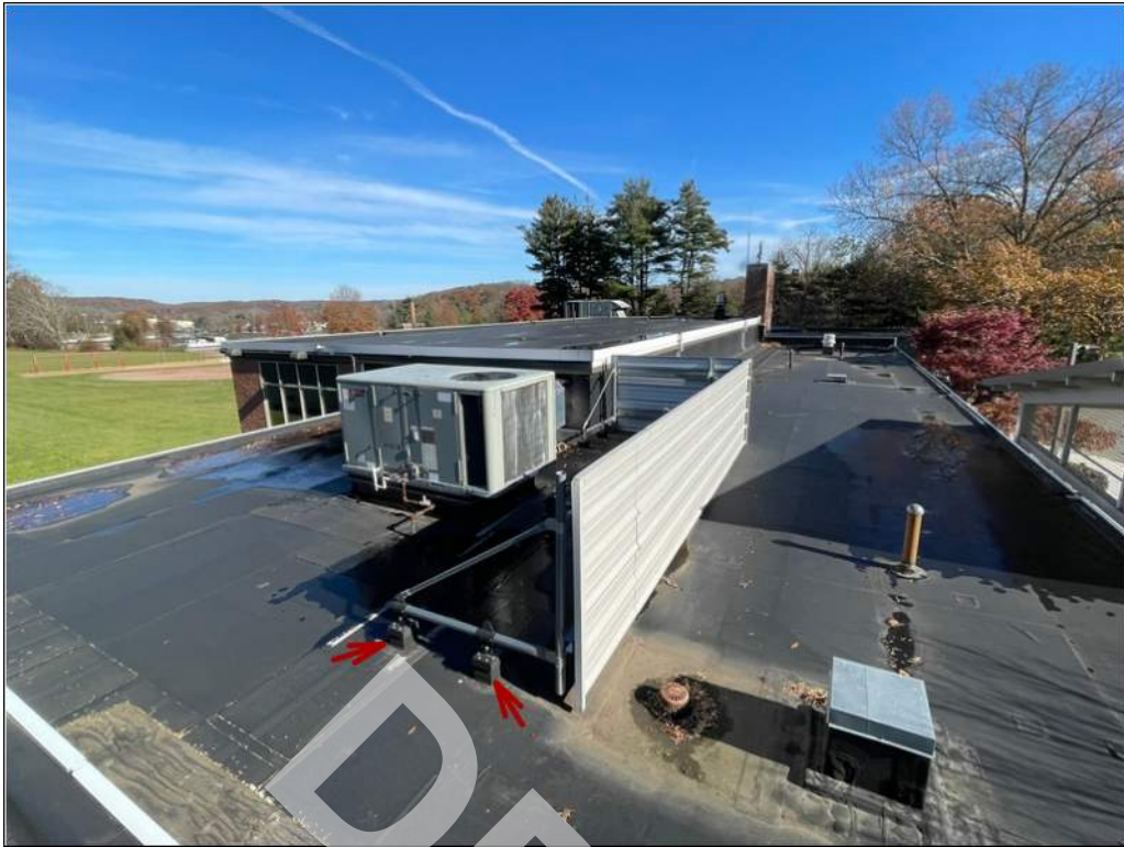
9 - Mechanical screen and supporting structure over the roofing system.
