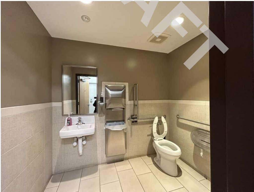
36 - Typical accessible single-user restroom.
