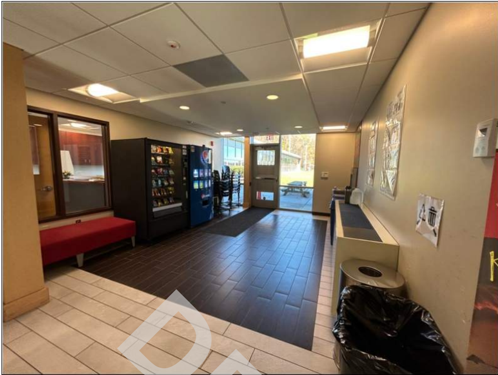
37 - The snack vending machine provided is not complaint as the operable parts are above the reach range.
