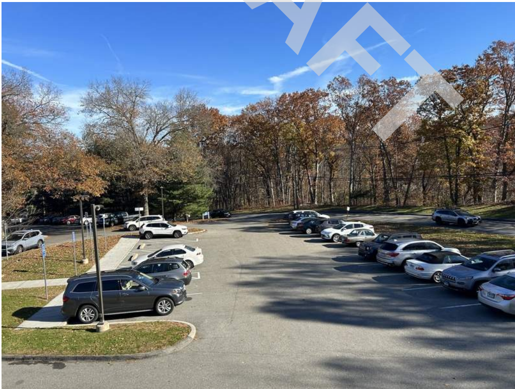
2 - Asphalt paved parking is provided at the front of the building.
