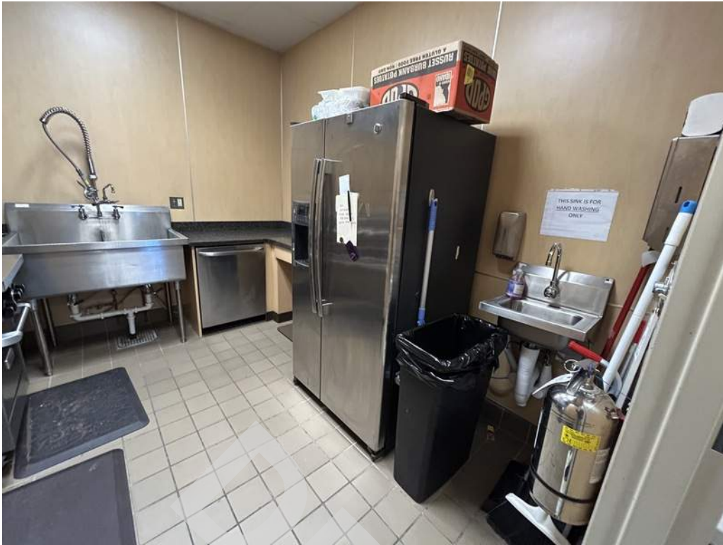
33 - Adequate clear floor space is not provided at the kitchen sink in the Senior Center Café.
