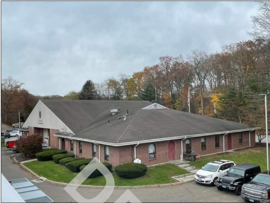
7 - Roof consists of asphalt shingles.
