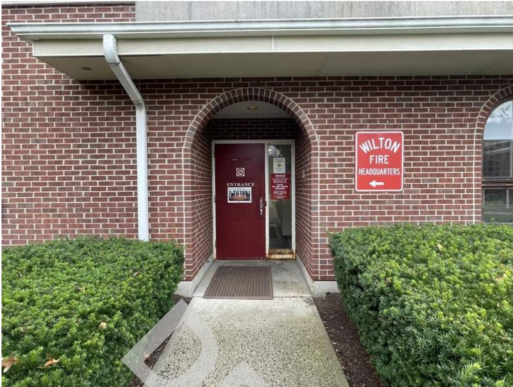
9 - Roof gutter and leaders are provided throughout the roof perimeter.
