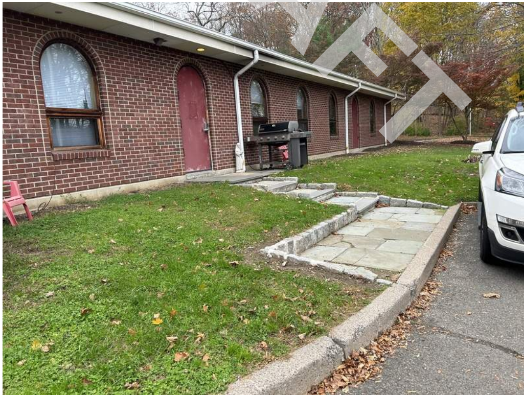
16 - Stone paver landing and steps are provided outside the volunteer meeting room exit door.
