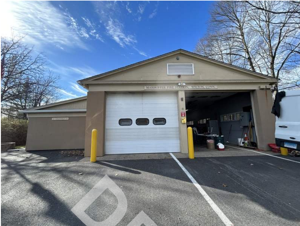
1 - Fire Station No. 2 front entrance.
