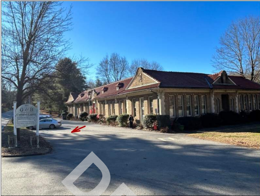
3 - Parking spaces in front of the building are not striped.
