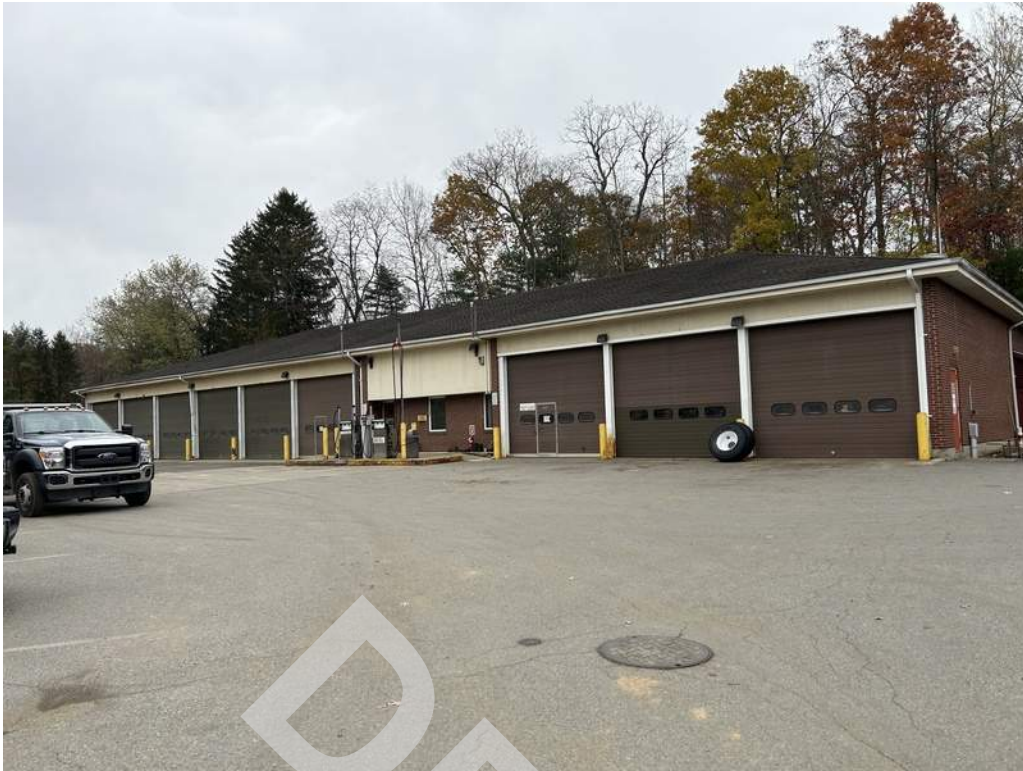
1 - Overview of the garage building.
