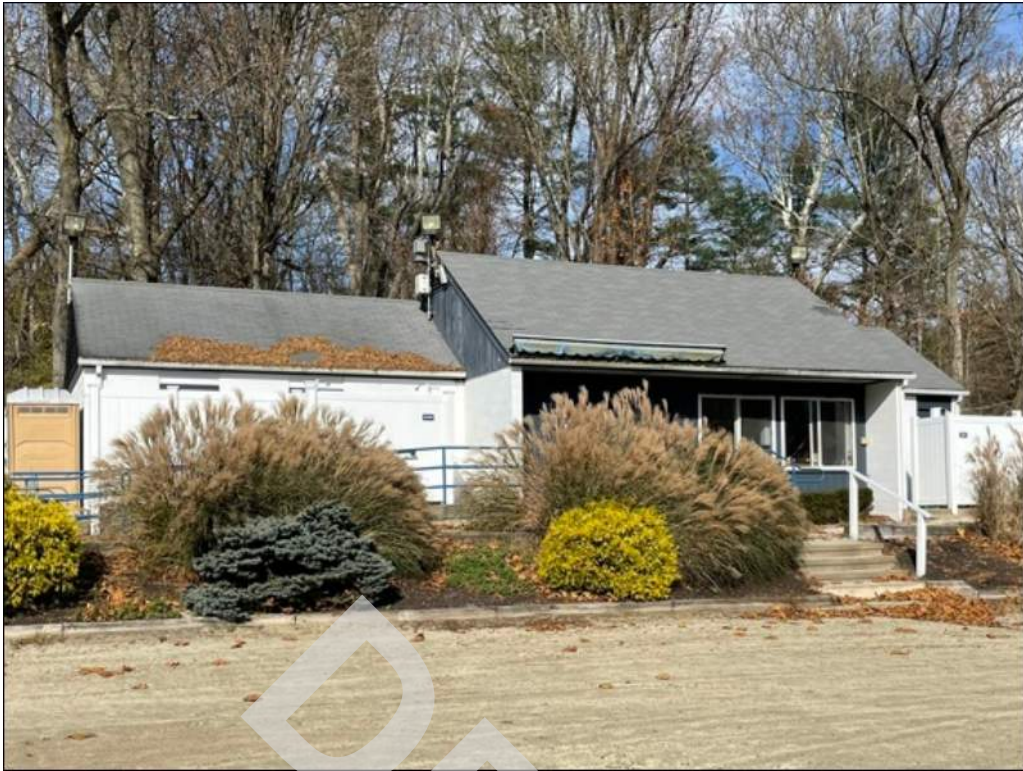
5 - Restrooms: Roof over the restrooms consists of asphalt shingles, walls consist of painted concrete masonry units and wood cladding.
