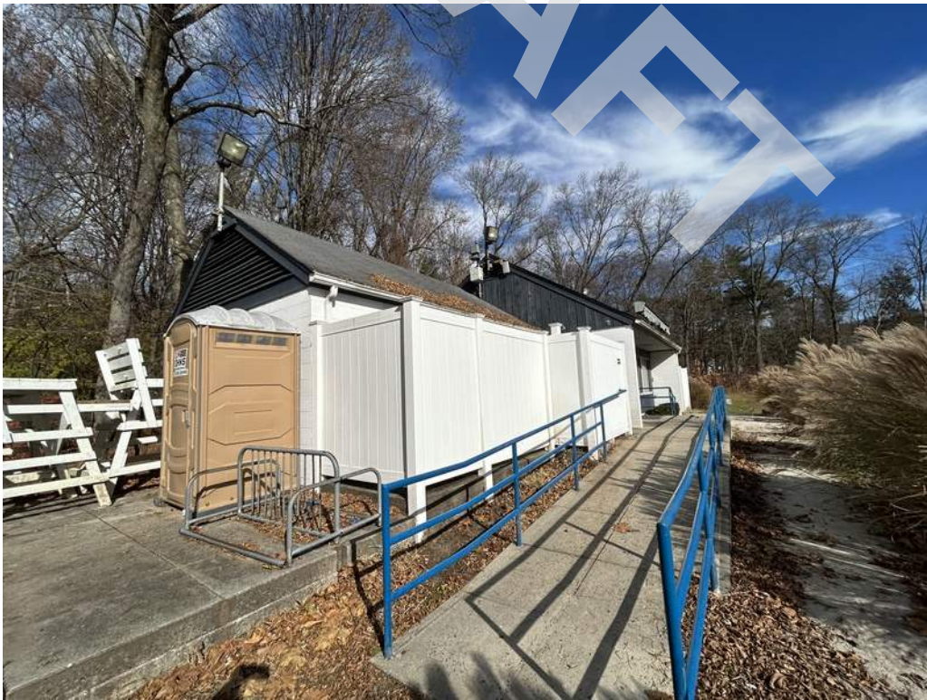
2 - Lifeguard office and restroom facility.
