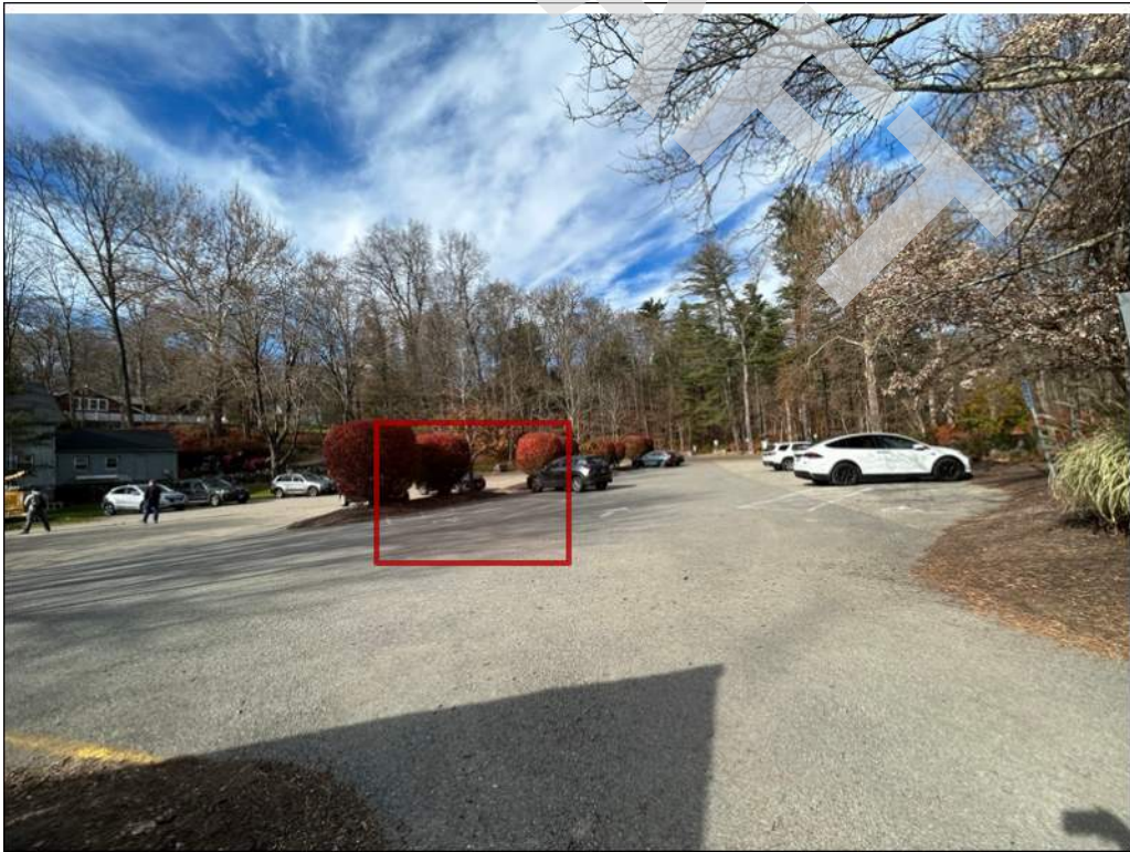
20 - Missing signage was observed at the accessible parking space.
