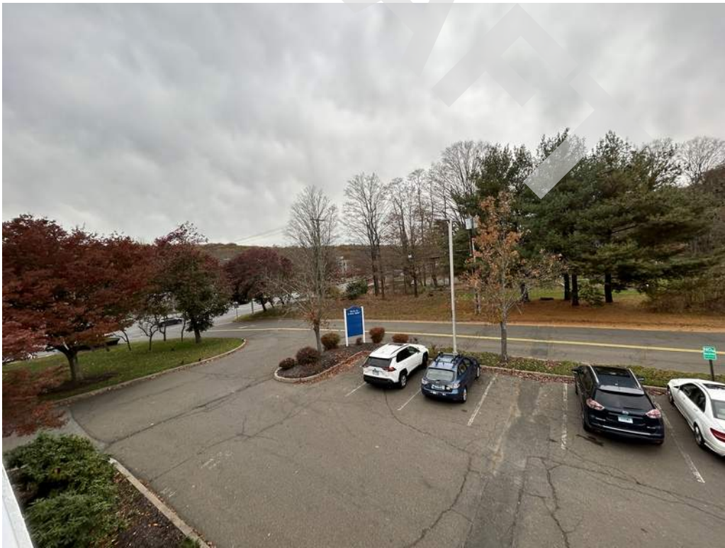
4 - Main vehicular access to the site is provided via a two-way curb cut off Danbury Road. Wayfinding signage is provided along the main drive lane. Site improvements consist of asphalt paved drive lanes and parking areas and landscaping.
