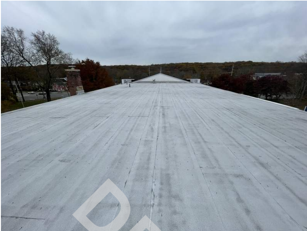
13 - Main roof consist of a modified bitumen roofing system.
