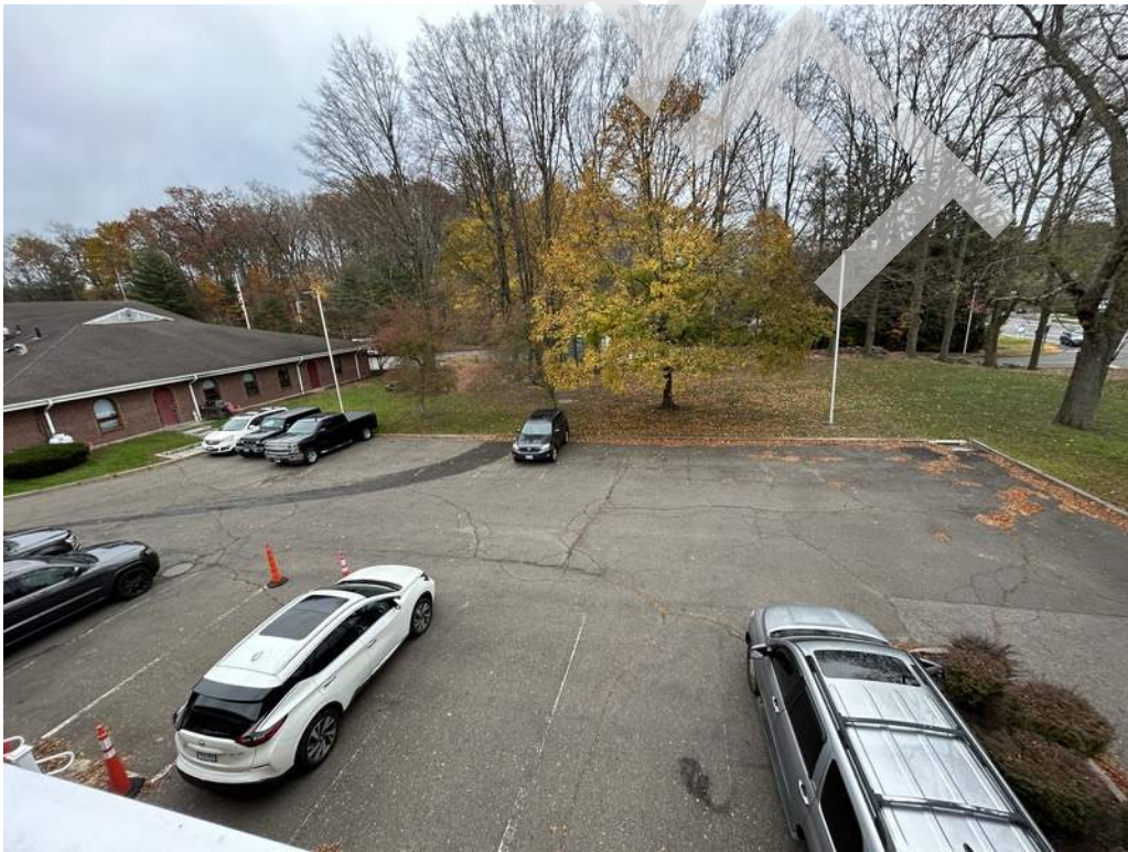
6 - Additional asphalt paved parking is provided on the south side of the building.
