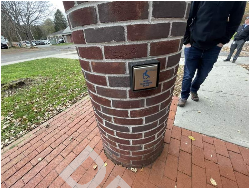
25 - Operated door push plate is located approximately 12' away from the door.
