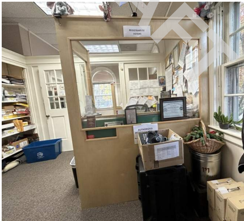
60 - A lowered counter area is not provided at the Registrants of Voters office.
