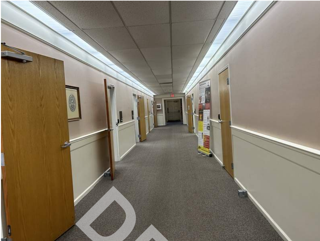
35 - Interior finishes at the corridors on the first floor typically consist of painted gypsum wall boards, suspended grid ceilings with acoustic tiles, and carpet floors.
