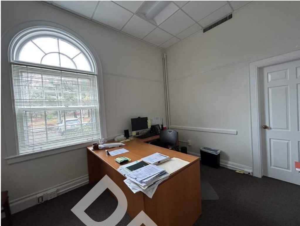
37 - Interior office finishes consist of painted gypsum wall board, suspended grid ceilings with acoustic tiles, and carpet floors.
