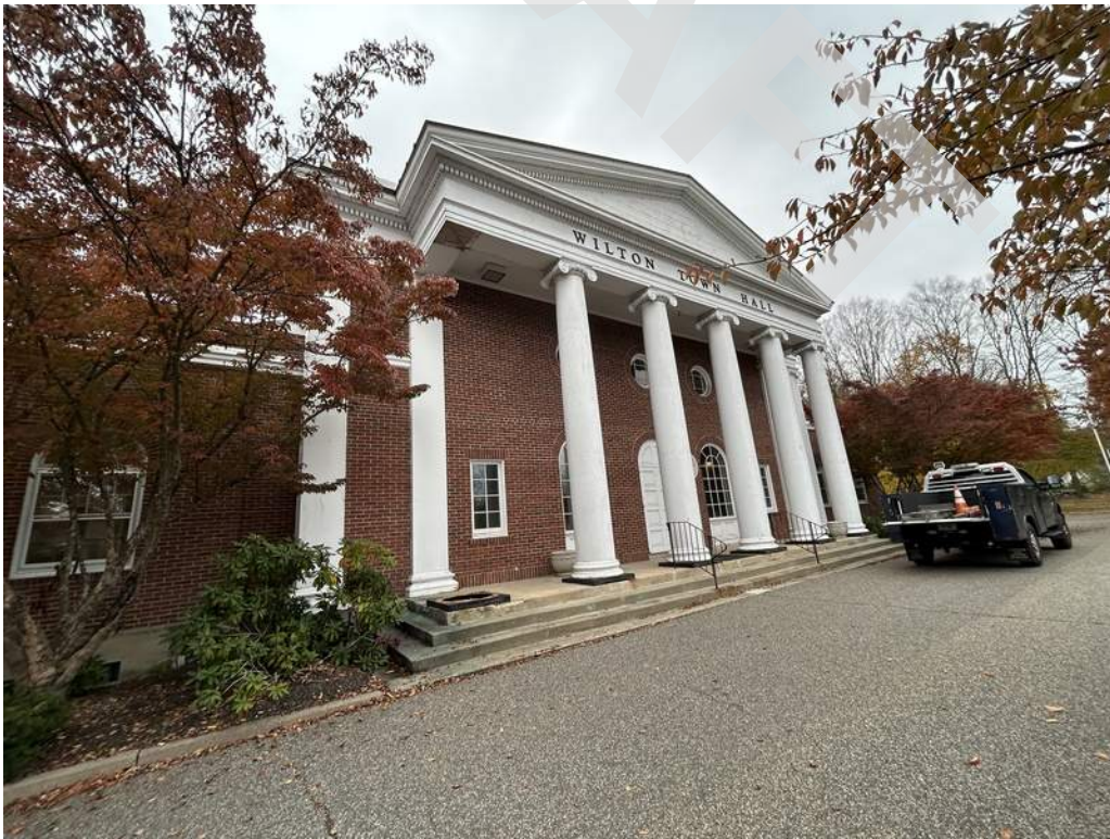
2 - Main entrance into the building is provided on the west side.
