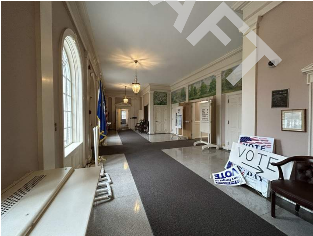
34 - Interior finishes at the lobby consist of painted gypsum ceiling and wall boards and terrazzo floors.
