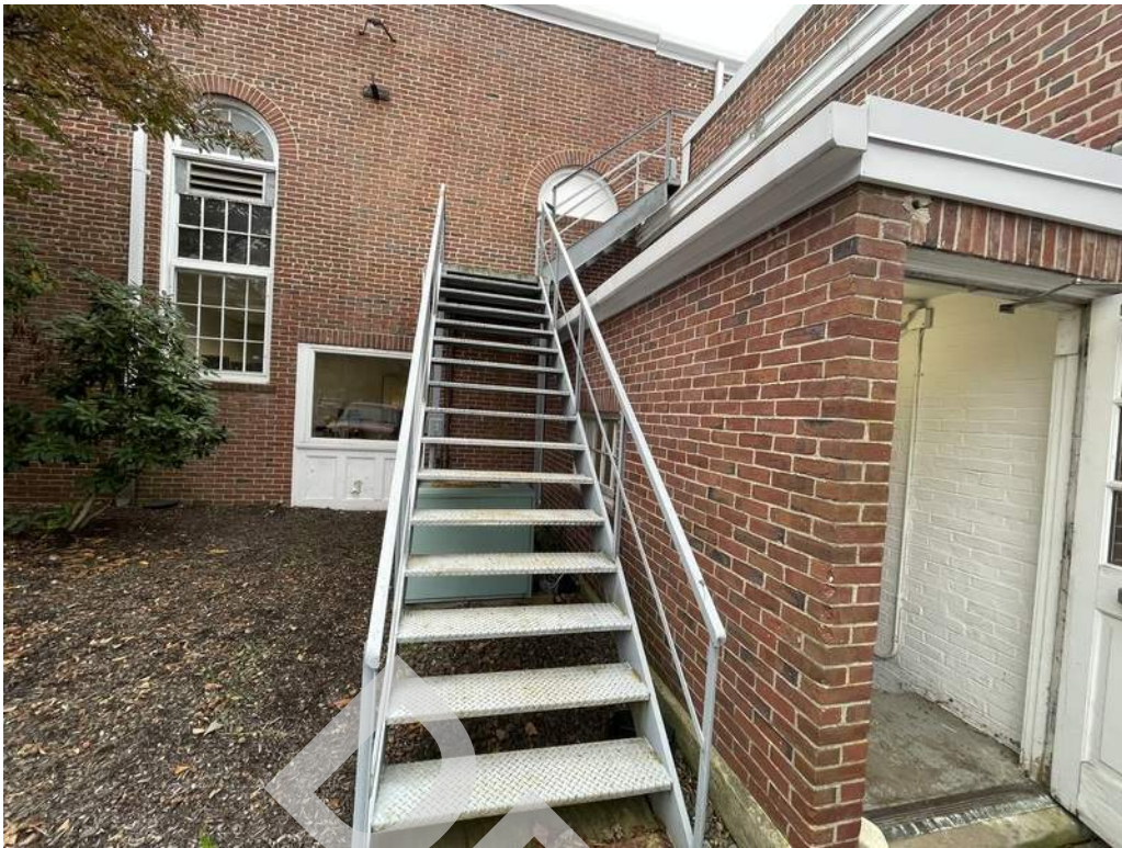
31 - Metal egress stair from the roof.
