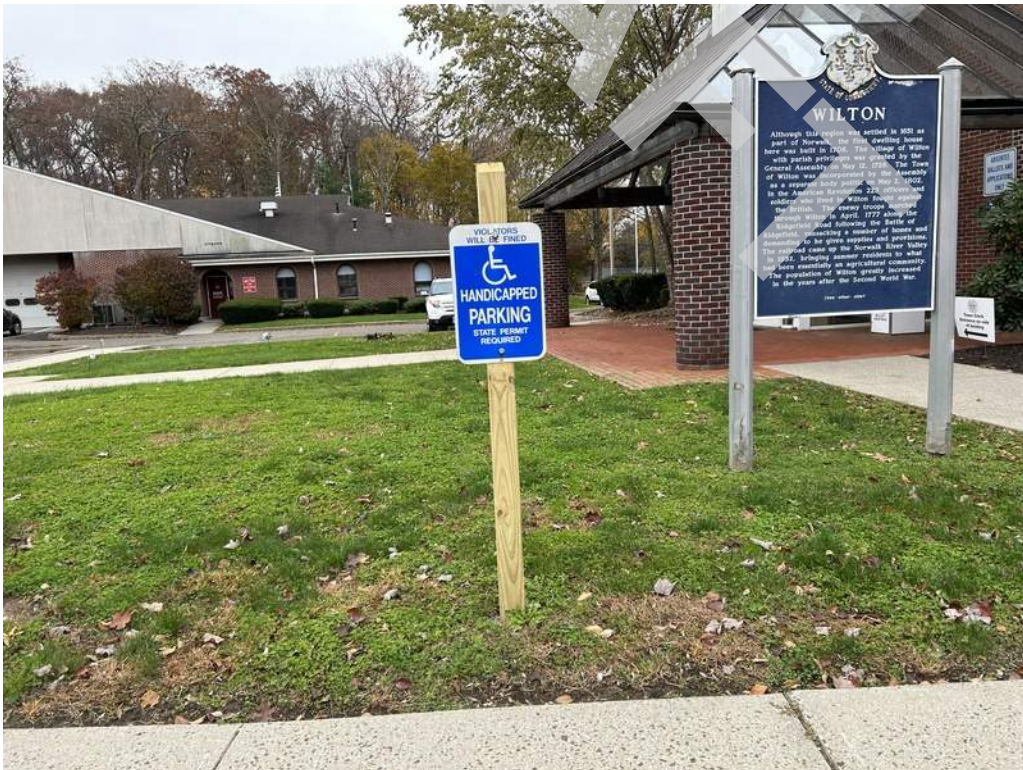
56 - Parking signage is mounted below the required minimum complaint height.
