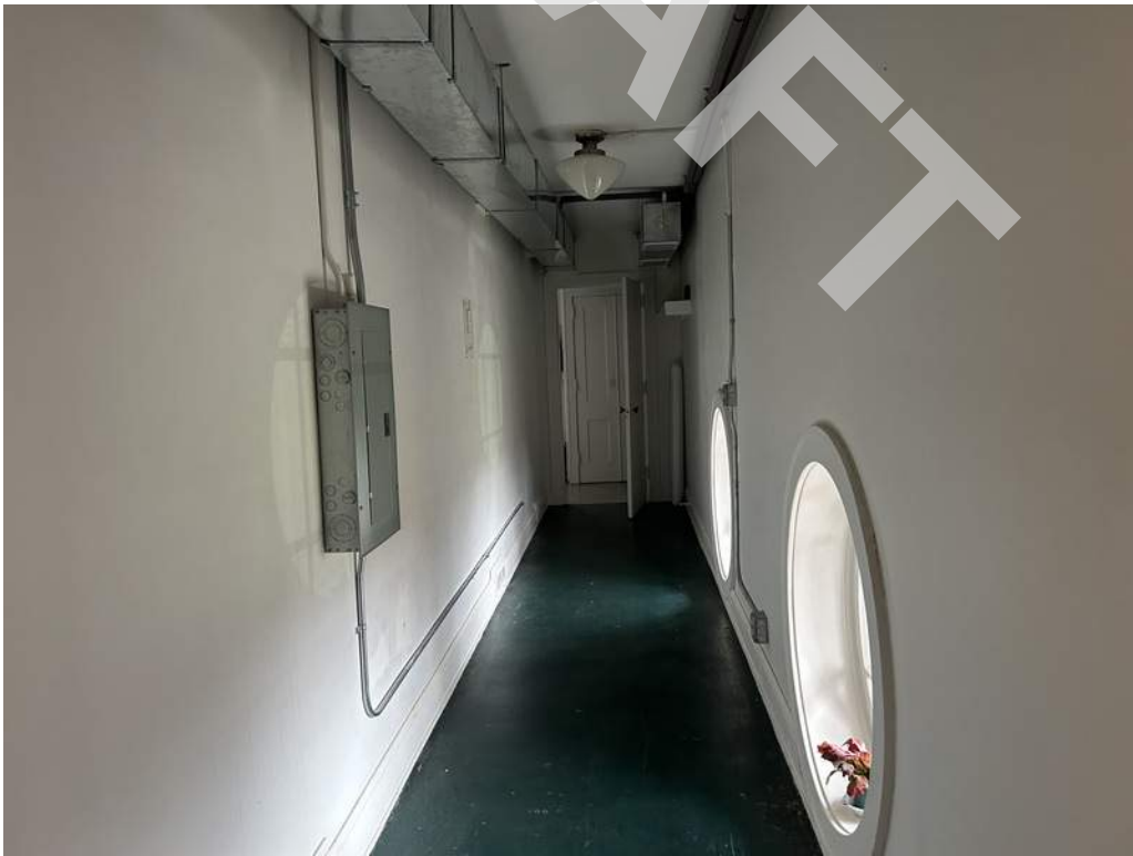
38 - Interior finishes at the second floor corridor consist of painted gypsum wall and ceiling boards and vinyl flooring.
