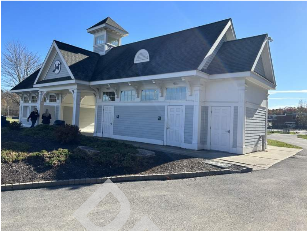
1 - Paving and landscape area along the north side of the building.
