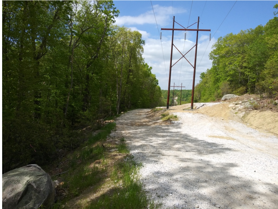
View of power line easement looking north taken by Vincent OBrien on May 22, 2020
