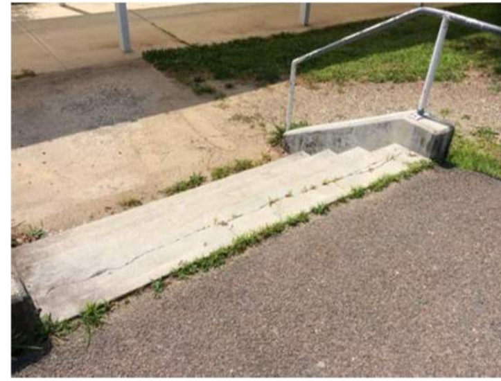
Rusting/Non-compliant railing
