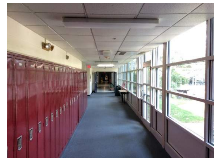
Old windows/limited insulation
