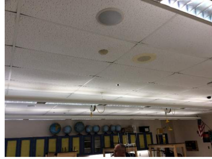
Replace ceiling tiles & lighting
