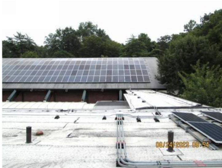
Replace built-up roofing
