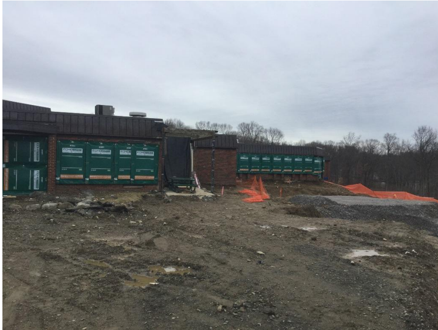
Demolition at Miller Connector
