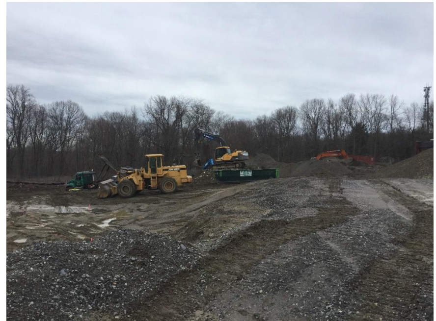
Crushed Peach Core Foundations
