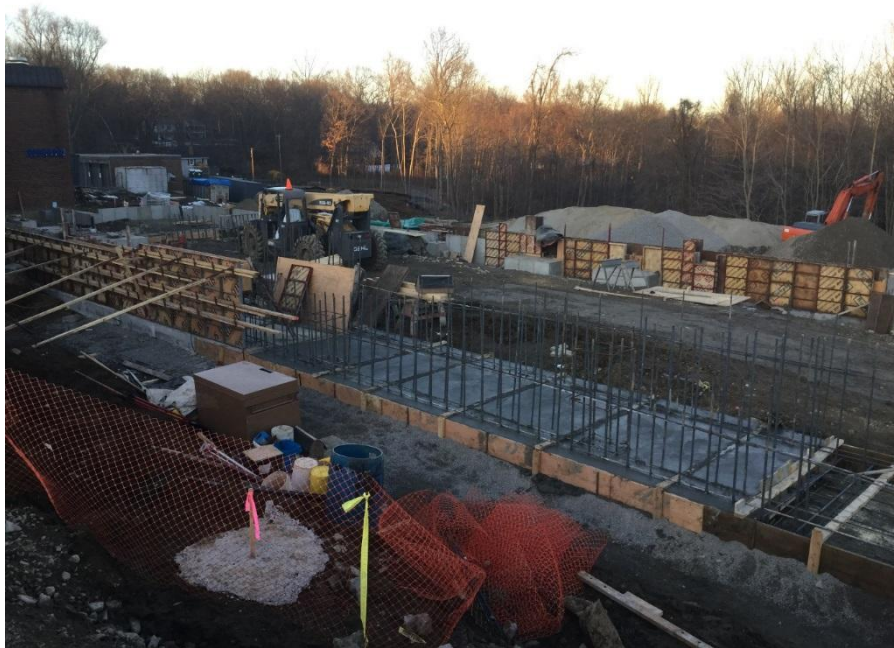
New Addition Foundations
