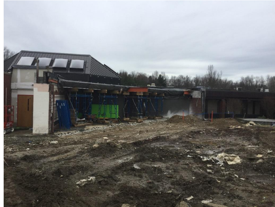
Demolition at Driscoll Connector
