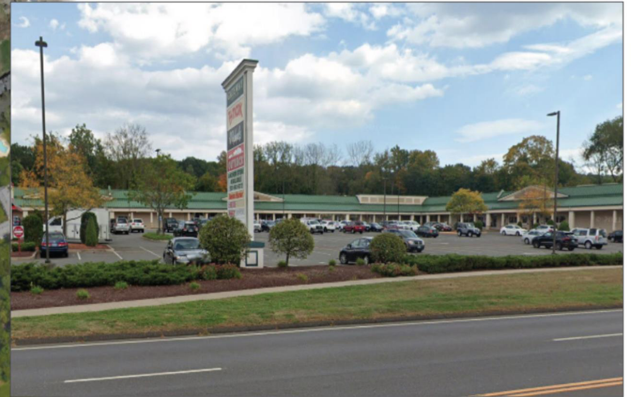
GATEWAY SHOPPING CENTER ADJACENT CONTEXT TO THE EAST 3
