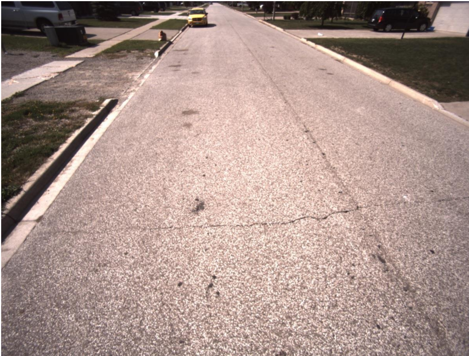
Sample good road – (71-85) (Light Green)
